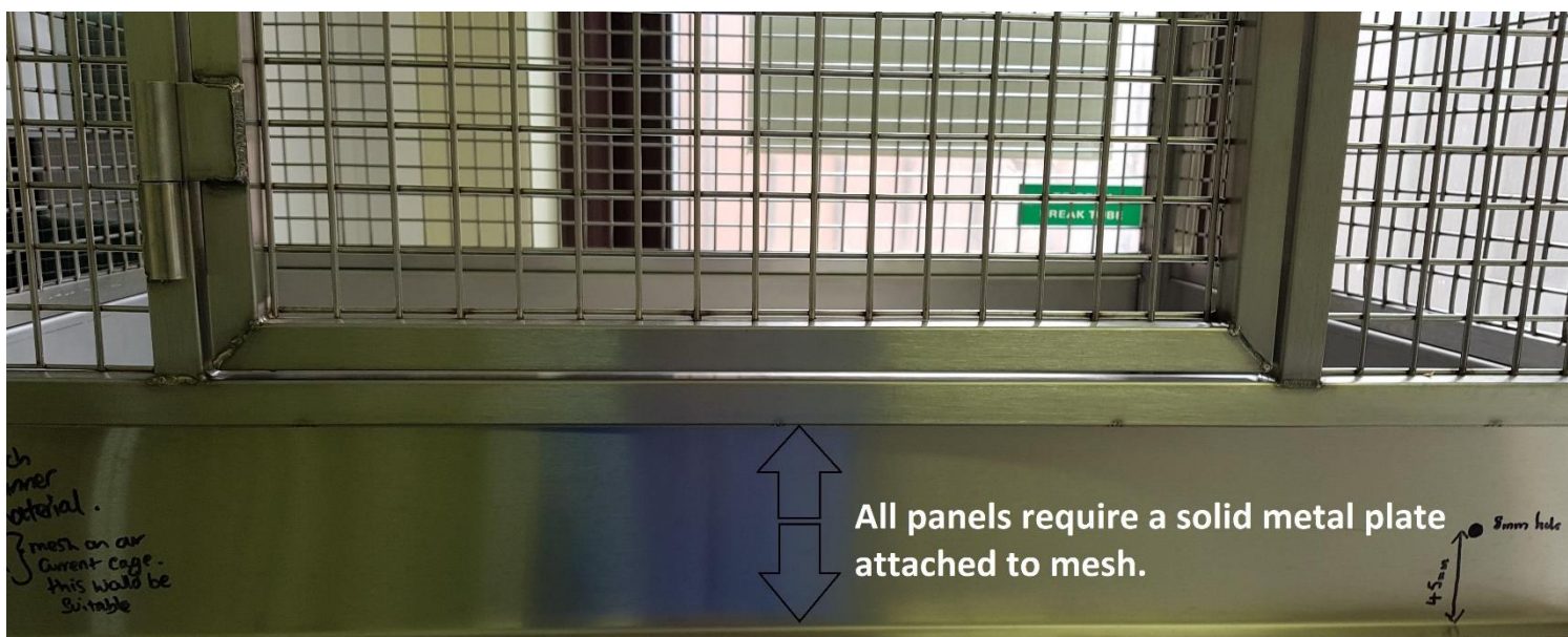
Fig. 14 & 15 – All sides of the cage will require a solid metal plate which is then attached to mesh. Mesh can be fused straight onto the metal plate, rather than the cage having further framing.
