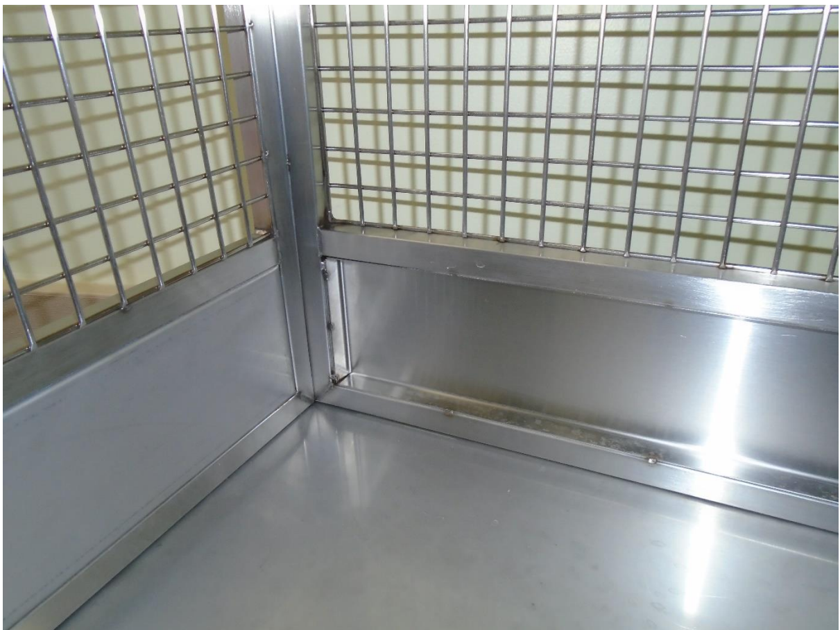
Fig. 15 – Another aspect of the metal plates. All internal areas must be smooth, like the left-hand panel in this photo.
