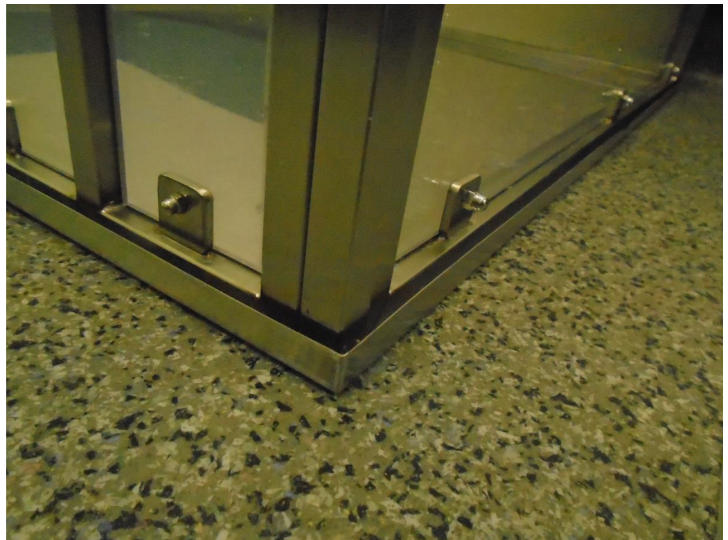
Fig. 3 - An example of the way in which the 4 side panels will sit into a metal base. They will not be fixed/attached to this base.
