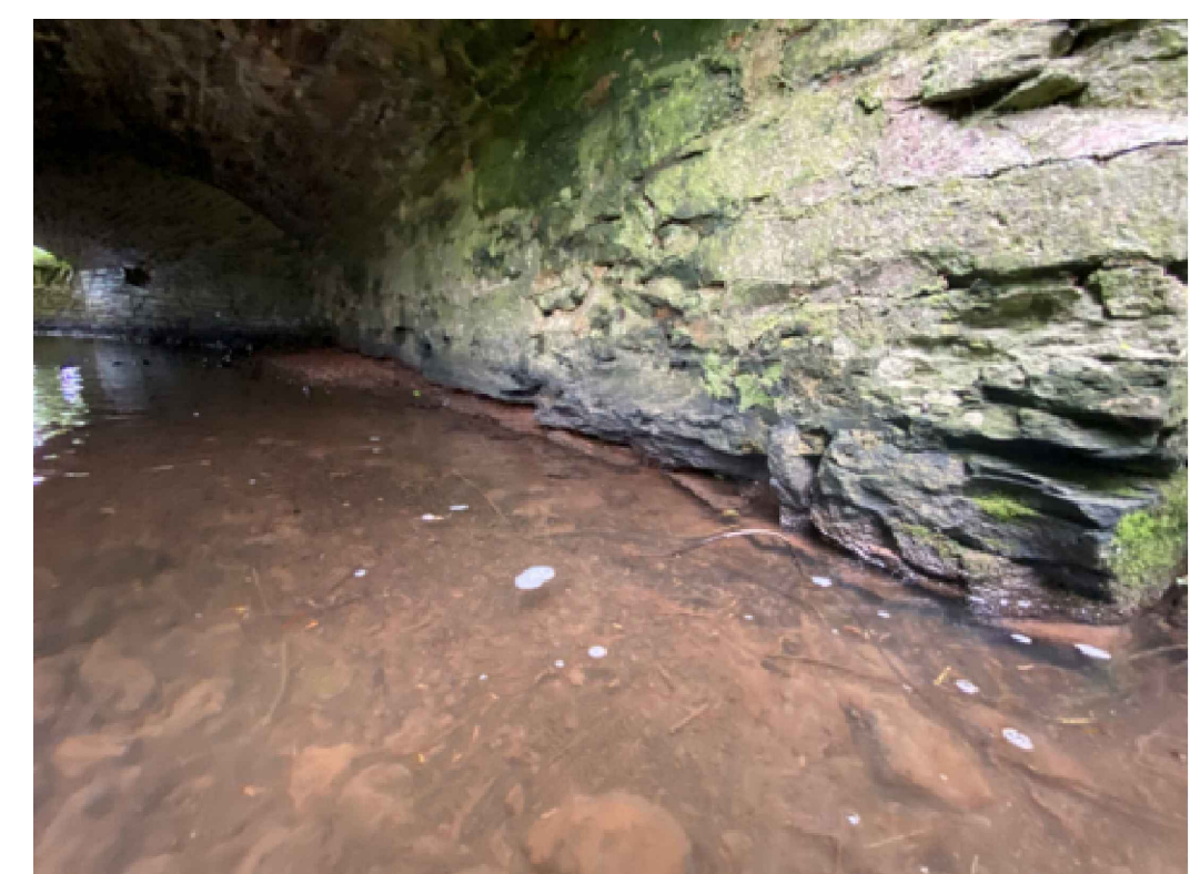
Photograph 1 - Scour at base of abutment
