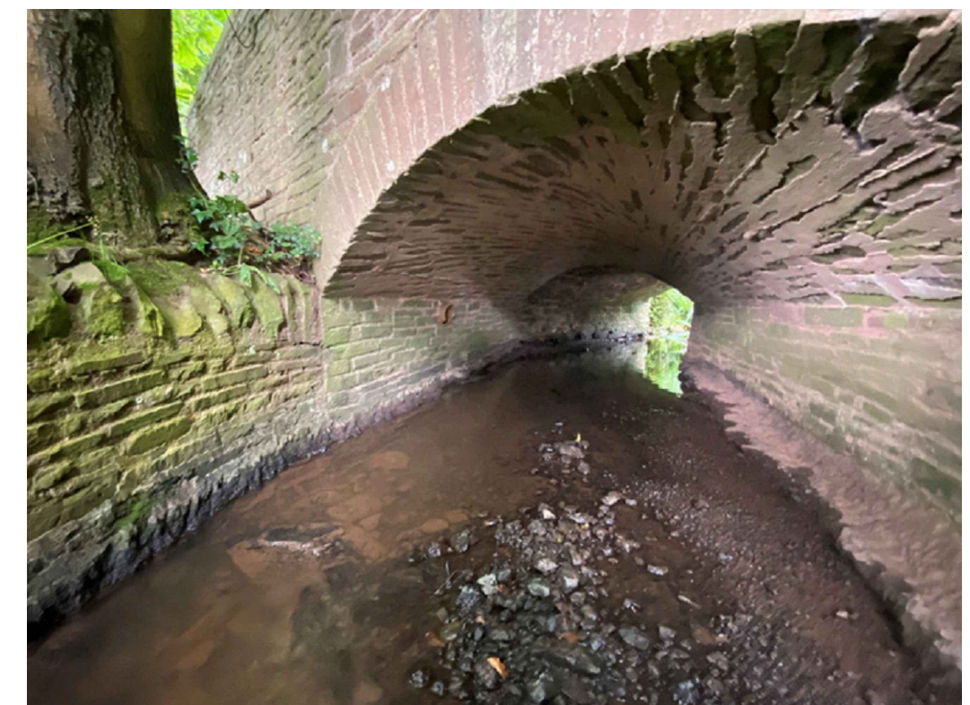
Photograph 2 - Bend in alignment of bridge
