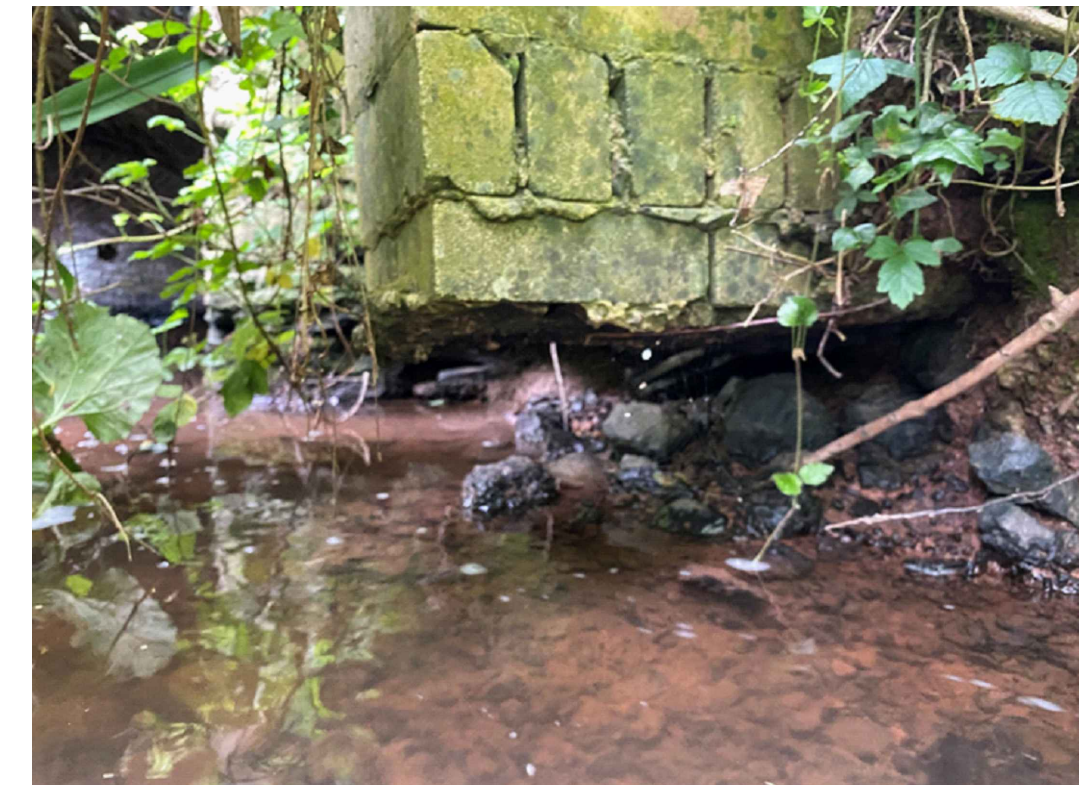
Photograph 3 - Complete scour under upstream wingwall
