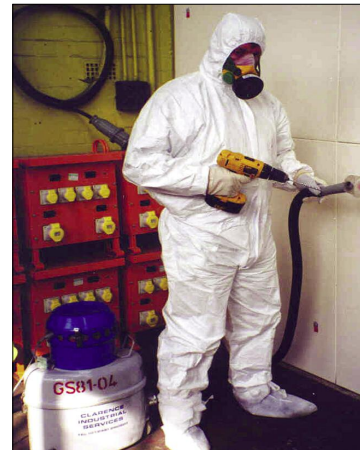
Using a Class H vacuum cleaner and a drill cowl
