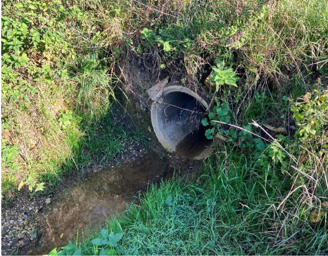
Photograph 9 showing culvert beneath track (centre of site)
