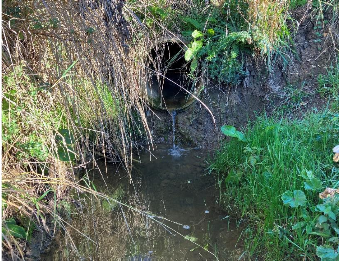
Photograph 5 showing culvert – 450mm diameter (north of site).
