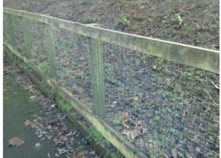
Finding: There are a number of loose posts around the Action: Monitor for any further deterioration and reset as required fence
