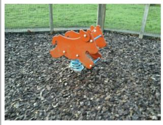
Finding: The paintwork on the spring has been damaged or worn exposing the metal underneath which is rusting
