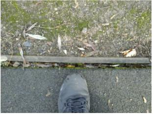
There are gaps opening between the wet pour surfacing and the edging surround or between the joints in the surfacing Monitor for any further deterioration and repair as required Finding: Action:
