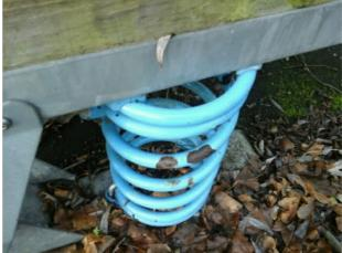
The paintwork on the spring has been damaged or worn exposing the metal underneath which is rusting Finding:
