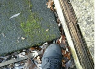
The wet pour surfacing is lifting at the edges and creating trip points Finding:
