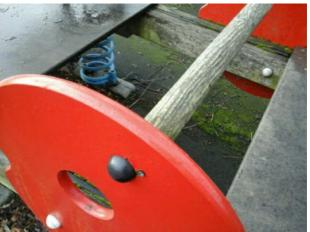
A number of fixing(s) have worked loose and **Action:** the handgrip is not secured Finding:
