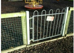
Finding: The gate is closing too quickly (less than 4 seconds)
