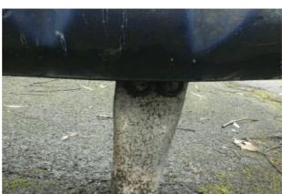
There is/are bolt cap covers missing or damaged on the item Finding:
