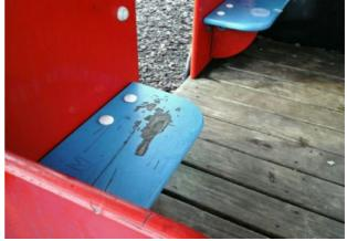
**Finding:** Parts of the timber are rough or splintered **Action:** Remove all rough or sharp edges and repaint affected areas
