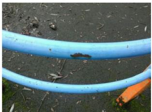
Finding: The paintwork on this item has been damaged or worn exposing the metal underneath which is rusting
