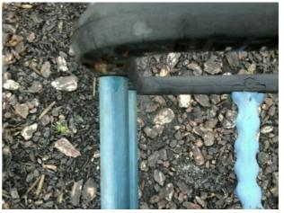
Finding: There are caps missing from the underside of **Action**: Replace missing caps under the seats
