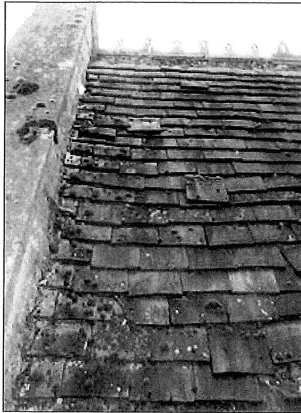
13. Typical slipped/replacement tiles and mortar flaunching to gable
