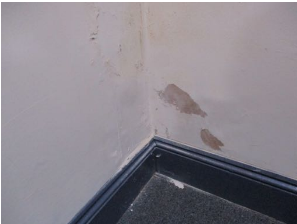
Photographs of Internal Dampness
