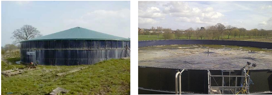
Figure 5. Slurry store covers; self-supporting cover on above ground slurry tank (left) and plastic floating cover (right)
