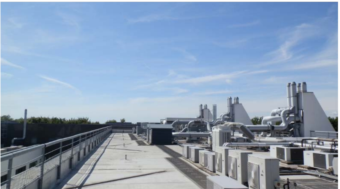
Image 5. General Roof view showing AHUs and Condenser Units
