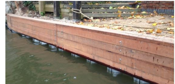
Image shows hard wood capping and waling
