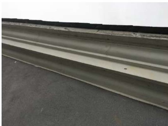
Photograph 11. Tightly fitted soffit of R3. Photograph 12. Gaps between soffit and slates on R3.
