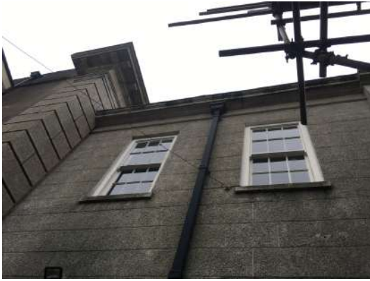
Photograph 4. Granite cornices of Roof No R1.
