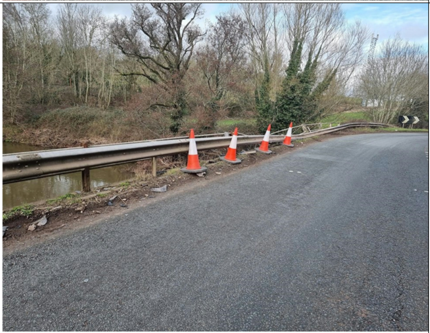
Damage upstream VRS
