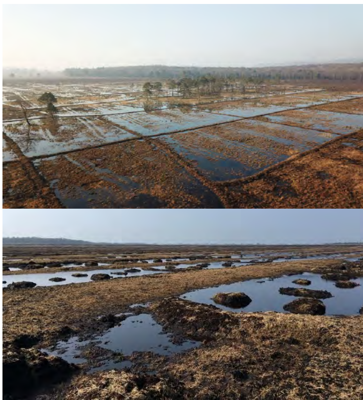
Figure 9 Top: Cell bunding at Roundsea woods & Mosses NNR. Photo Credit: Conservfor. Bottom: Horseshoe bunds at Bolton Fell Moss. Photo Credit: Deborah Land
