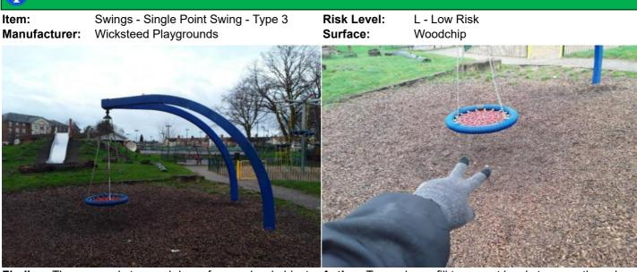
Finding: The exposed stone sub base forms a hard object within the impact area of the equipment in contravention of the requirements of BS EN 1176 Part 1
