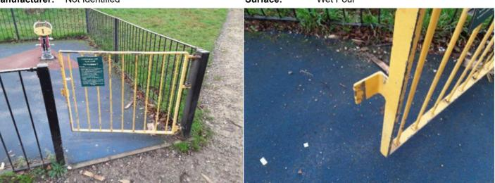
Finding: The rubber buffer is missing from the latch plate
