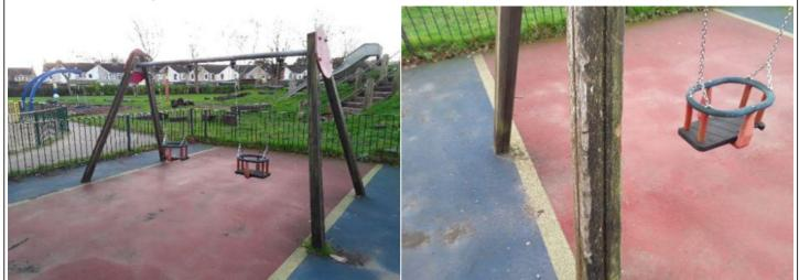
Finding: Parts of the timber are rough or splintered
