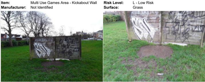
**Finding:** The surface has eroded in some areas and may be **Action:** Reinstate the surface slippery in wet conditions
