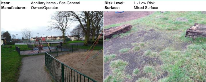
**Finding:** There is algae, silt or moss growth on the surface **Action:** Clean and treat appropriately resulting in slippery conditions
