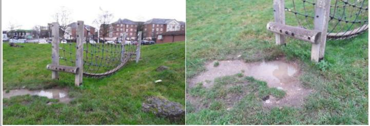
**Finding:** The grass has eroded within the impact area of the **Action:** Reinstate the grass or provide an all weather equipment and may not provide the necessary impact attenuating properties for the equipment fall height; the surface may also be slippery in wet weather
