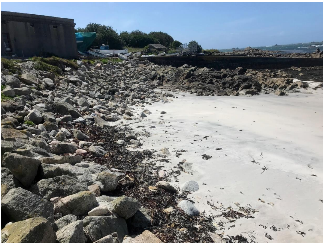
Figure 12: South end of Periglis where beach meets the slipway, showing informal dumping of rock on rock bar and sand foreshore (middle distance) and more formally placed rock (foreground)
