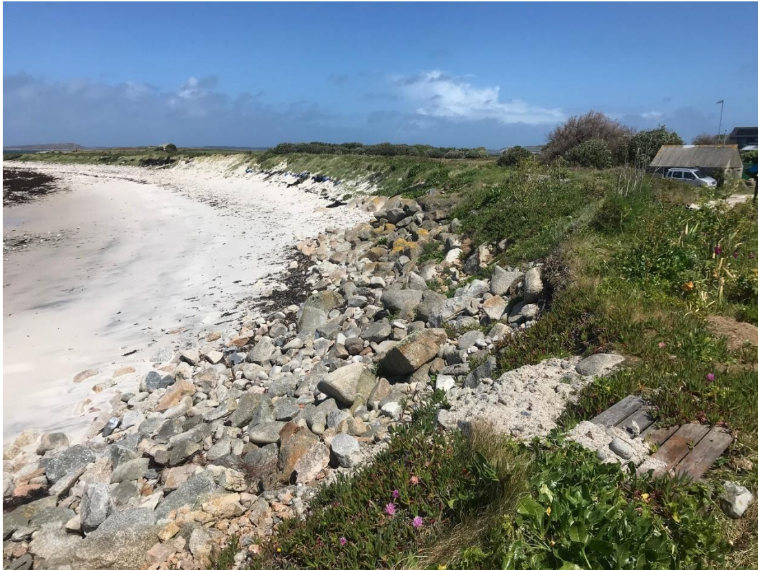
Figure 9: Periglis to the north of the beach access, mixture of rock of varying sizes, rock encapsulated in mesh bags (in distance) and sand beach
