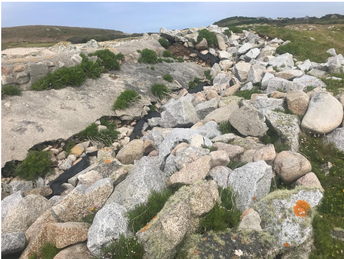
Figure 13: Scouring of the north-eastern seawall at Great Popplestone, Bryher
