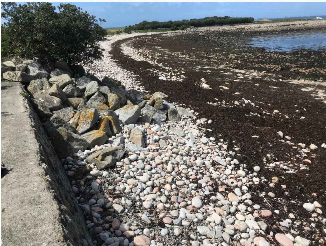
Figure 6: Porth Killier showing the rock revetment at the transition between the two elements of sea defences, looking west
