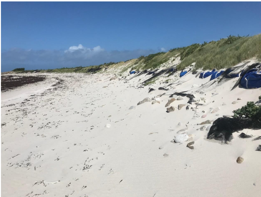
Figure 10: Periglis in the middle of the beach, showing blue dumpy bags filled with sand overlying mesh layers covering rock armour and beach with sand dunes vegetated with marram
