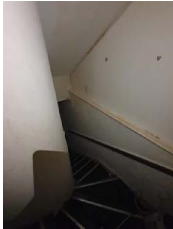
Photo006 – B01 - Top of Basement Stair
