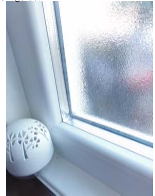
Photo296 – G11 - WC 3 - Window WG2
