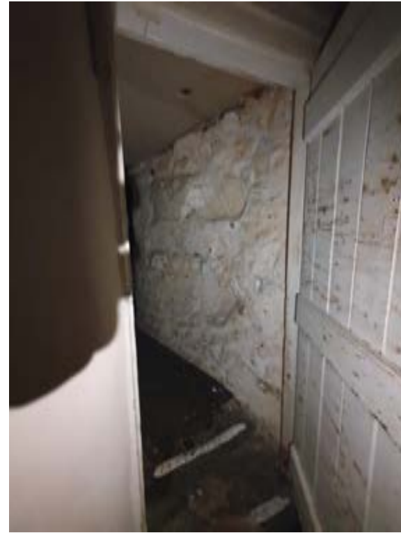
Photo021 – B02 - Basement Hall and Bottom of Stair - Door DB6
