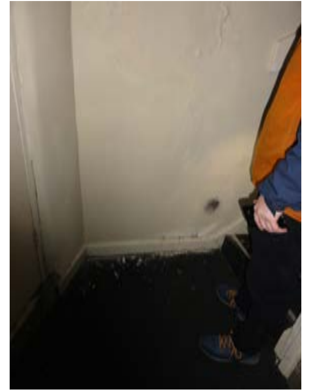
Photo031 – B02 - Basement Hall and Bottom of Stair
