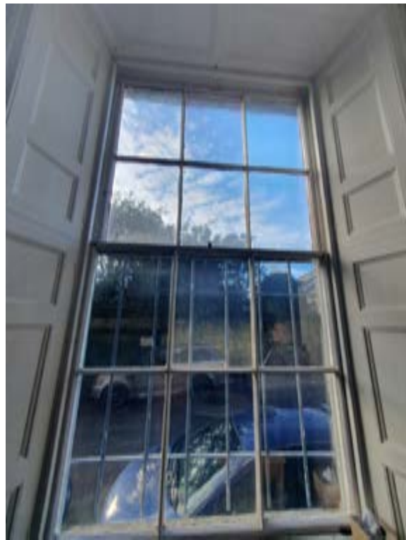
Photo251 – G06 - Office 3 - Window WG6 and shutters.
