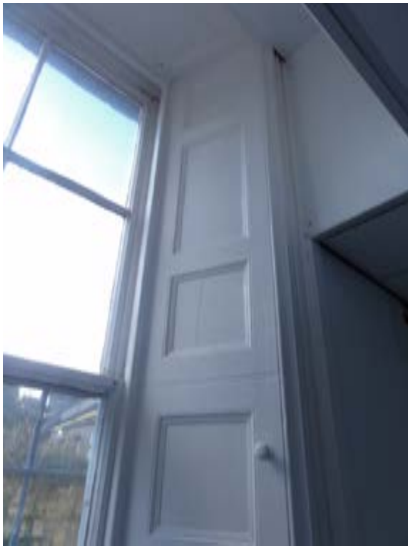
Photo234 – G04a - Lobby - Window WG7 and shutter
