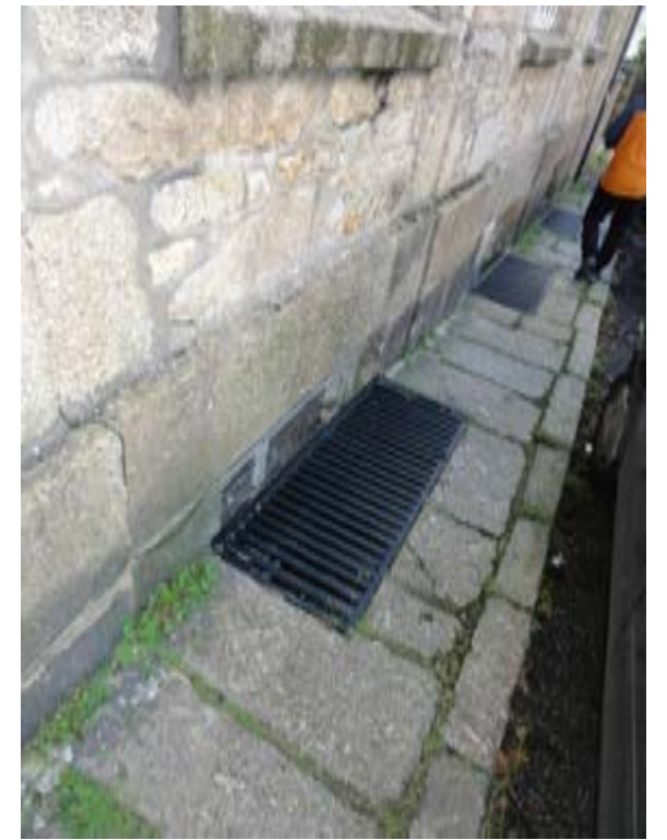
Photo383 – External - Basement Window Grilles
