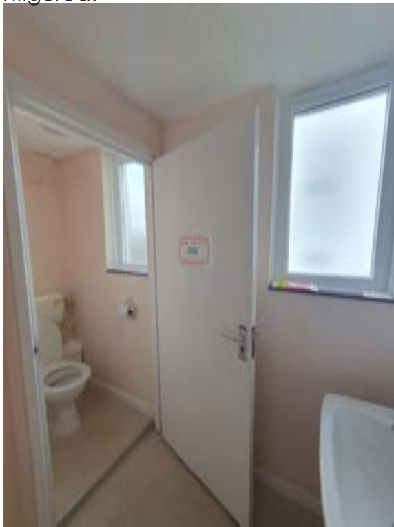
Photo290 – G10 - WC 2 - Windows WG3 and WG4. Door DG26 (To be removed). Layout to be reconfigured.
