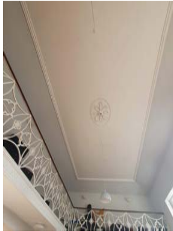
Photo339 – F05 - Meeting Room - Balcony Above
