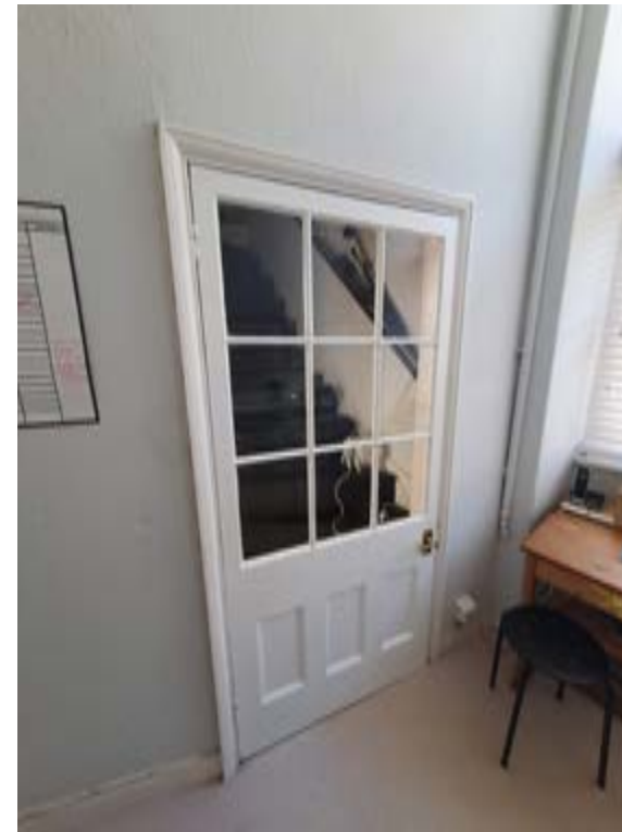
Photo326 – F03 - Kitchen 2 - Window WF6 and Door DF3
