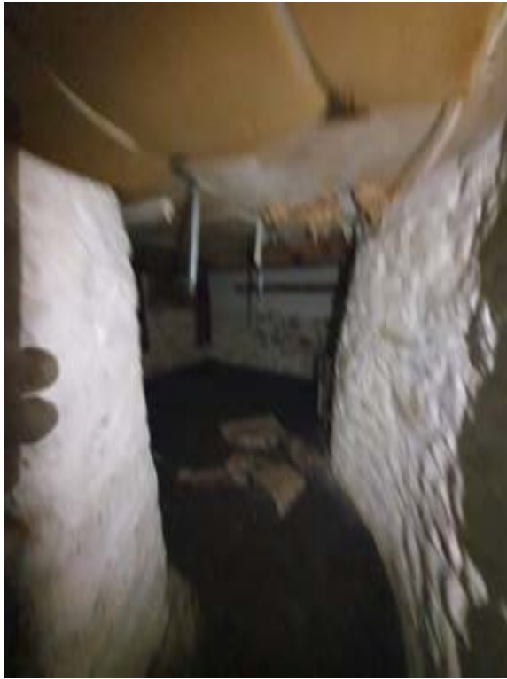
Photo033 – B03 - Basement Room 1
