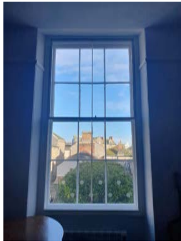
Photo315 – F02 - Office 3 - Window WF1 with Secondary Glazing.
