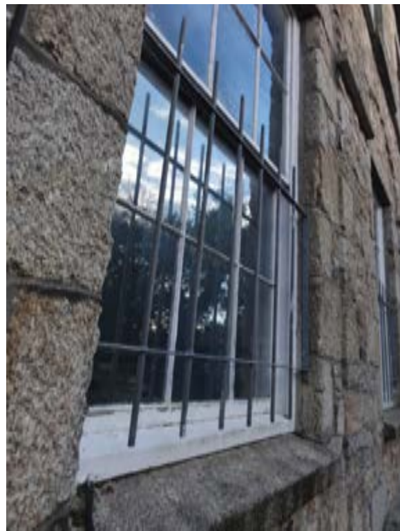
Photo388 – External - Window WG8
