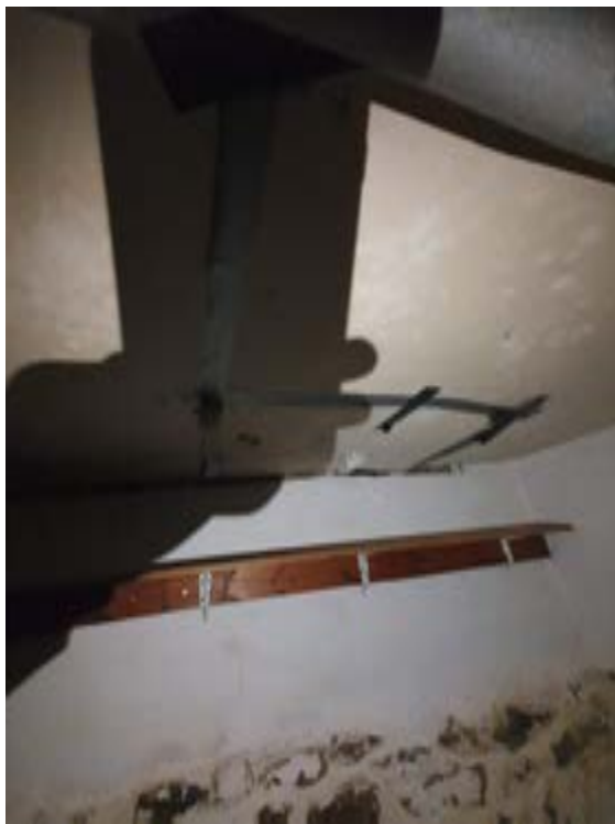
Photo042 – B03 - Basement Room 1
