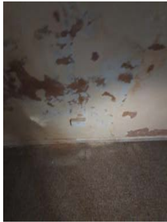
Photo099 – B05 - Basement Room 3
