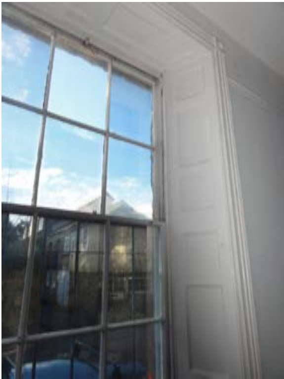
Photo216 – G04 - Office 2 - Window WG8 and shutter
