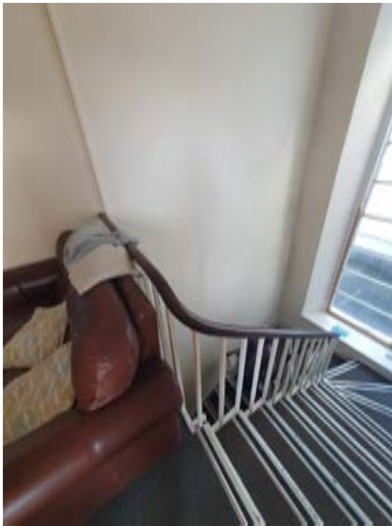
Photo306 – F01 - Landing - Top of Stair - Window WF2
