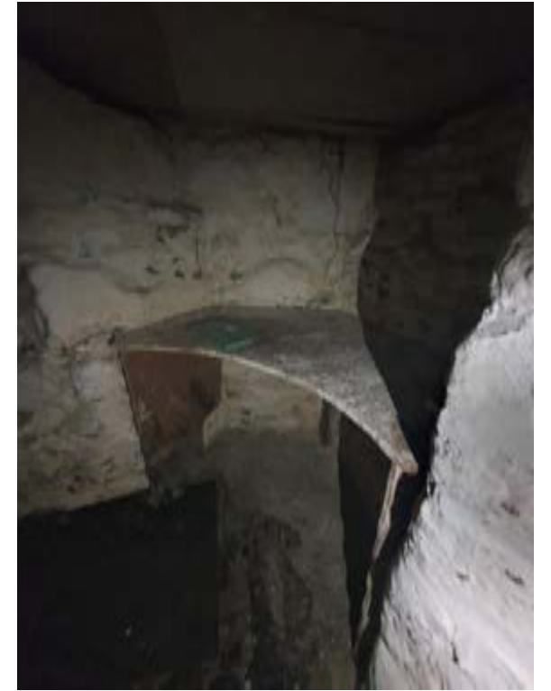
Photo047 – B03 - Basement Room 1
