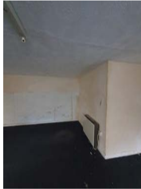
Photo069 – B04 - Basement Room 2
