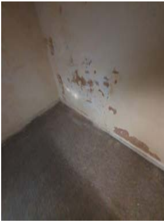
Photo097 – B05 - Basement Room 3
