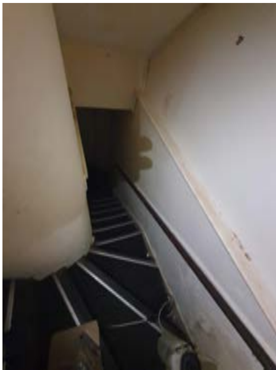
Photo005 – B01 - Top of Basement Stair
