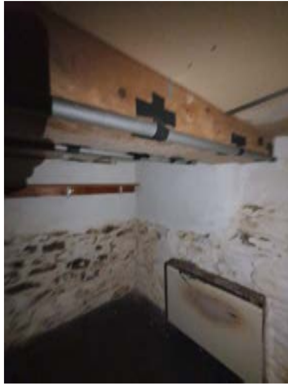
Photo043 – B03 - Basement Room 1
