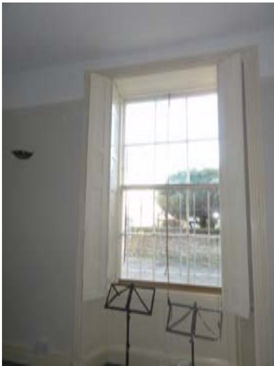
Photo130 – G01 - Office 1 - Window WG1
