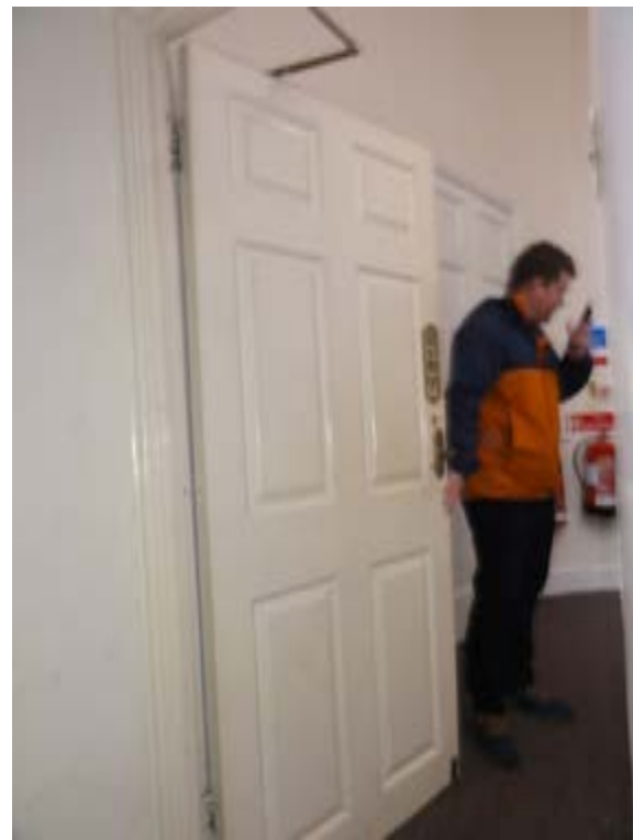
Photo012 – B01 - Top of Basement Stair - Door DG10
