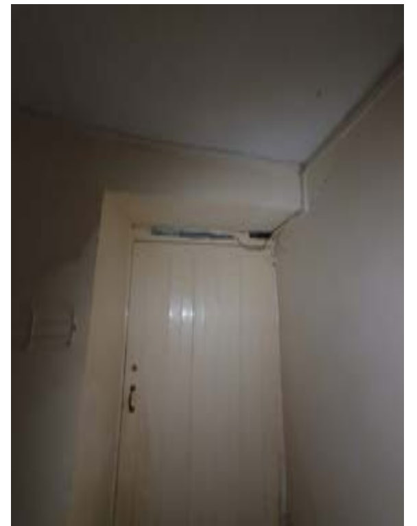
Photo024 – B02 - Basement Hall and Bottom of Stair - Door DB3
