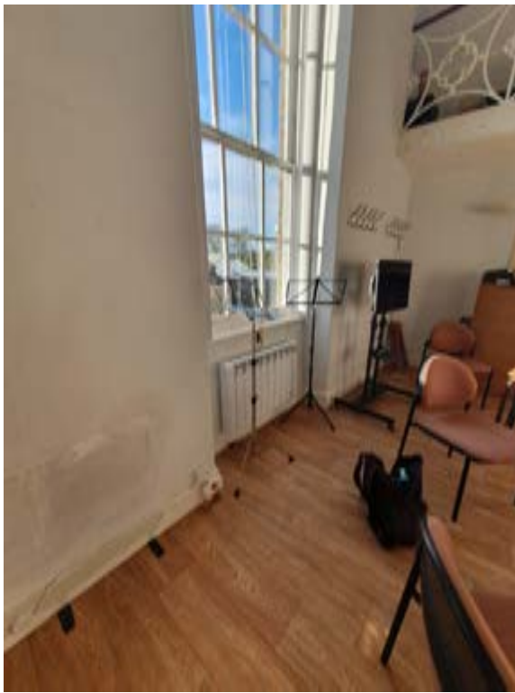
Photo345 – F05 - Meeting Room - Window WF5
