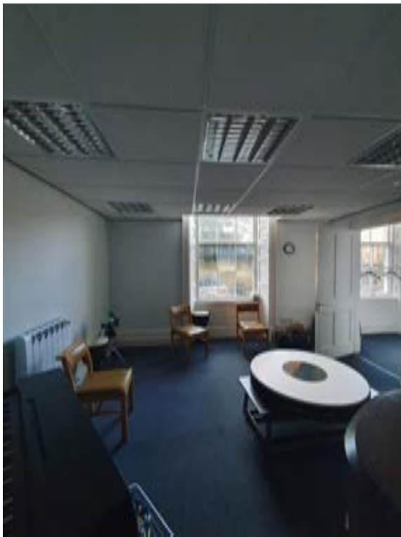
Photo257 – G06 - Office 3 - Window WG6 and Door DG22 (To be removed). Suspended ceiling to be removed.
