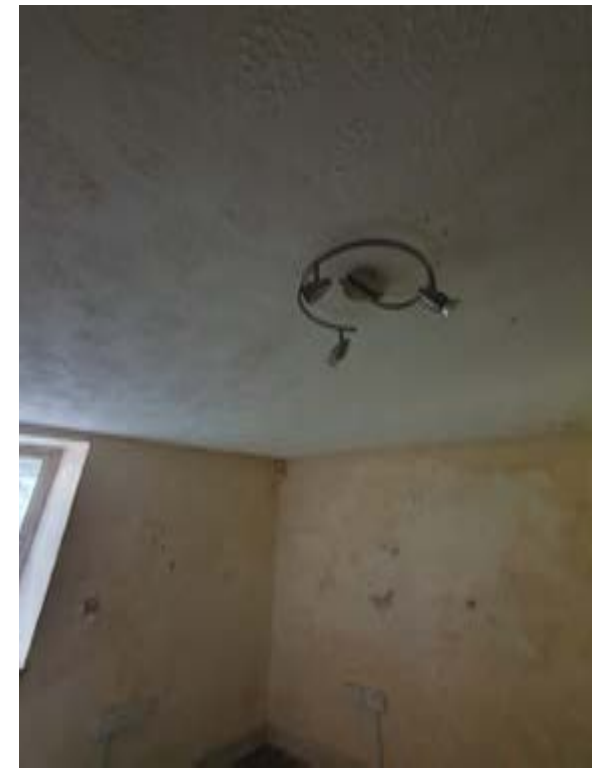
Photo103 – B05 - Basement Room 3
