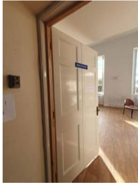
Photo307 – F01 - Landing - Door DF1
