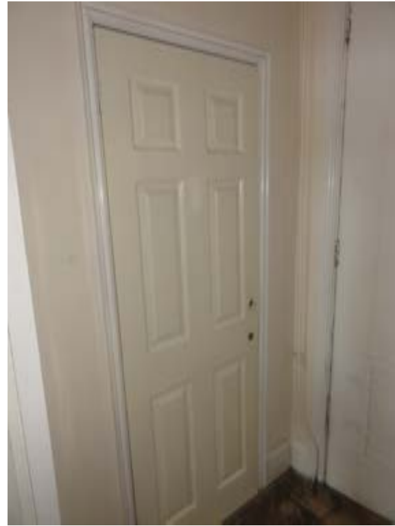
Photo147 – G02 - Entry - Doors DG1 and DG2
