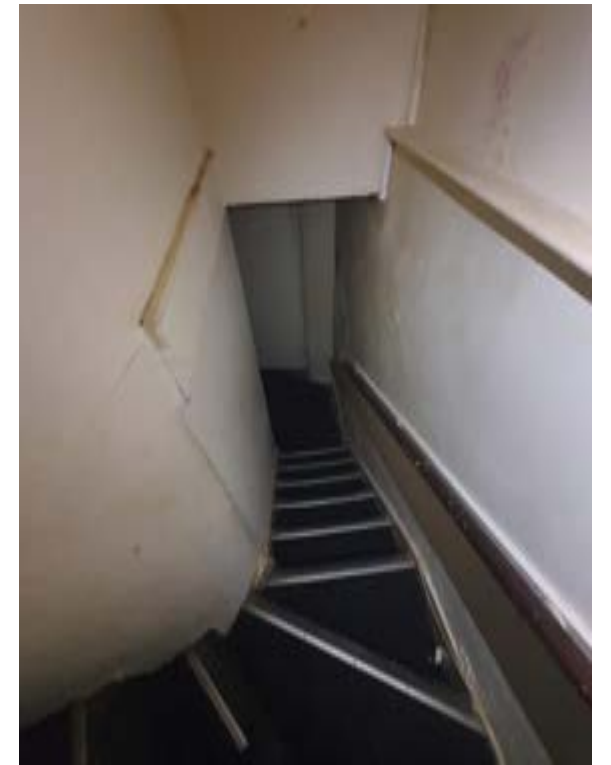
Photo008 – B01 - Top of Basement Stair
