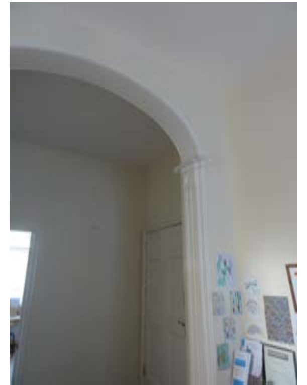
Photo312 – F01 - Landing - Doors DF4 and DF5
