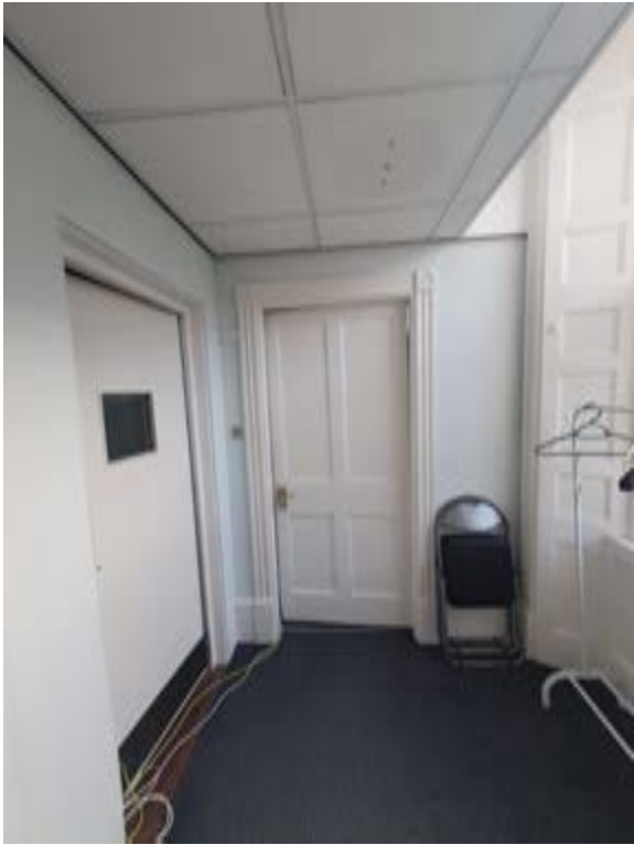
Photo221 – G04a - Lobby - Doors DG21 and DG22 (To be removed) - Suspended ceiling to be removed.
