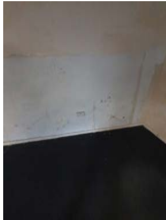
Photo076 – B04 - Basement Room 2
