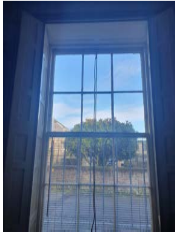
Photo115 – G01 - Office 1 - Window WG1
