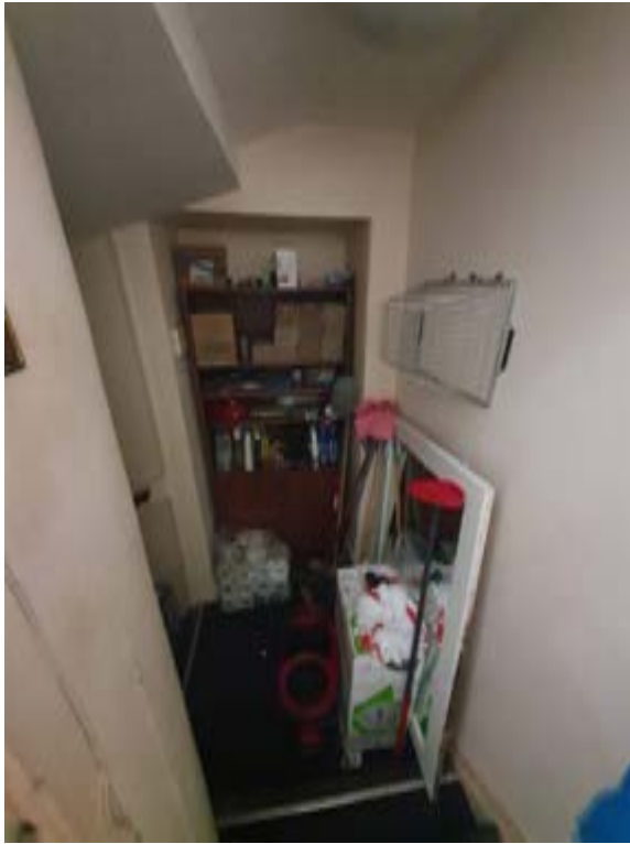
Photo001 – B01 - Top of Basement Stair
