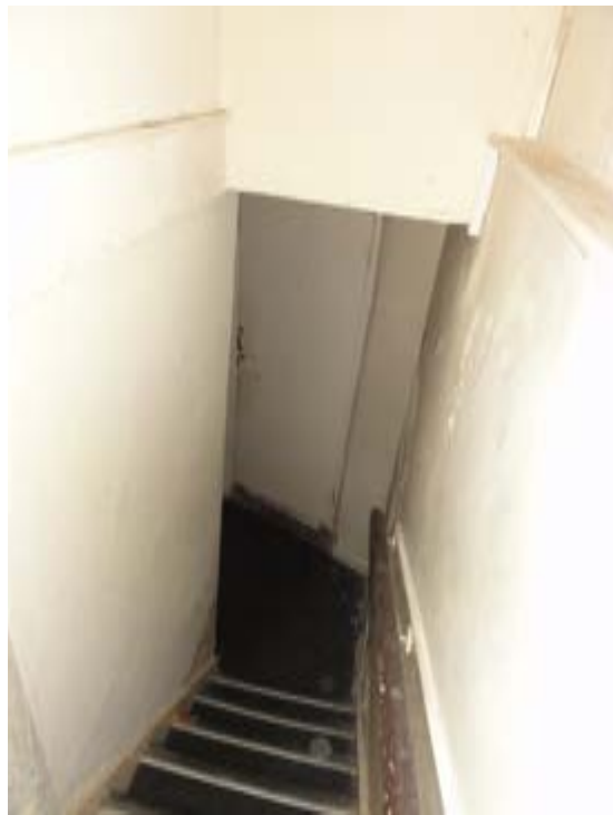
Photo010 – B01 - Top of Basement Stair
