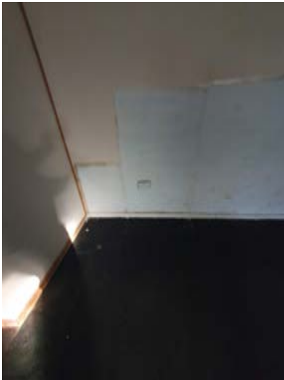
Photo074 – B04 - Basement Room 2
