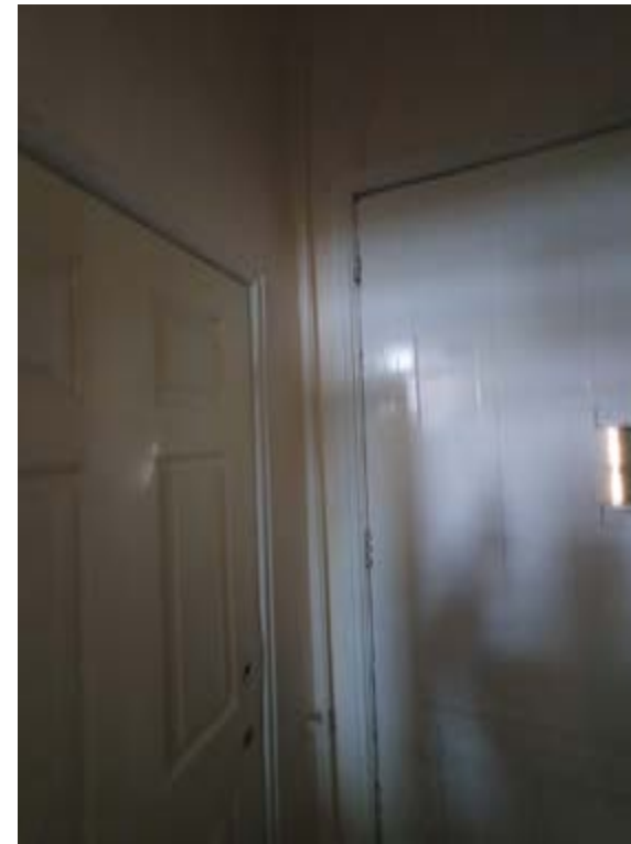
Photo142 – G02 - Entry - Doors DG1 and DG2
