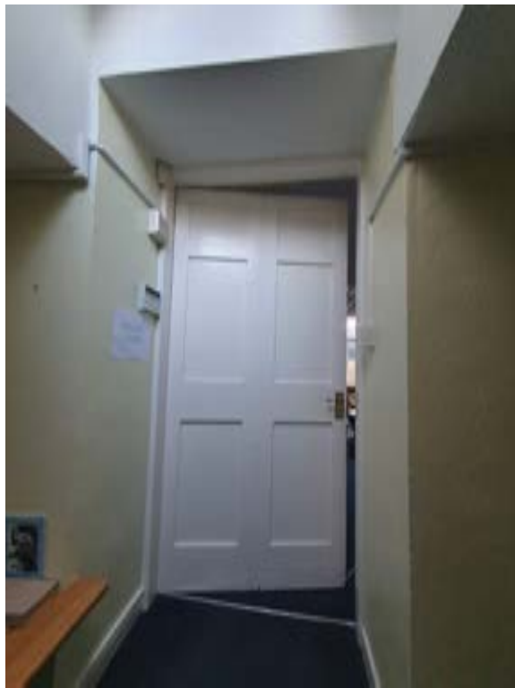
Photo271 – G07 - Kitchen 1 - Door Dg14
