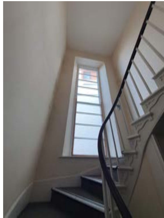
Photo156 – G03 - Ha11 1 and bottom of stair - Window WF2
