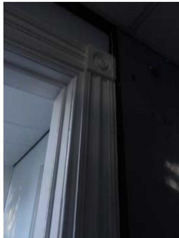
Photo260 – G06 - Office 3 - Door DG22 (To be removed)
