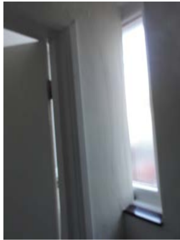
Photo299 – G11 - WC 3 - Window WG2 and Door DG24. . Layout to be reconfigured.
