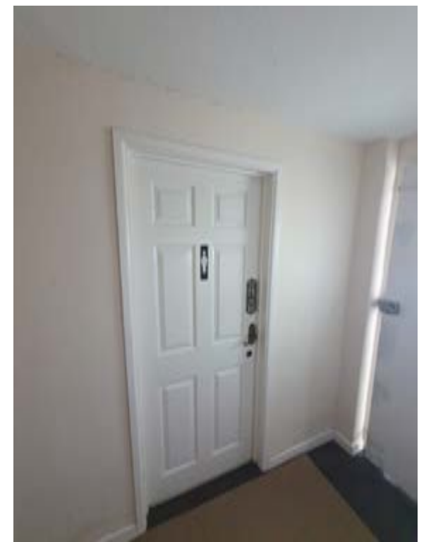
Photo288 – G09 - Entry Lobby - Doors DG9 and DG25 (To be removed). Layout to be reconfigured.
