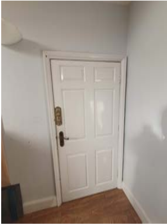
Photo337 – F05 - Meeting Room - Door DF2
