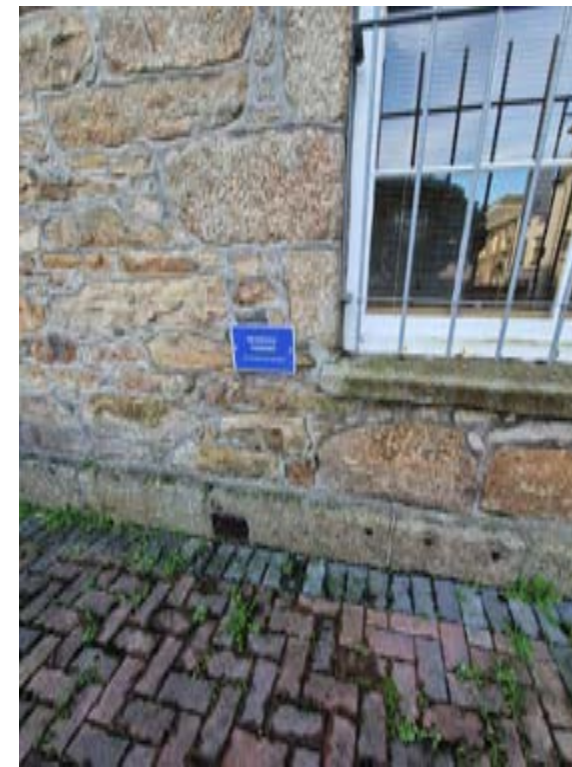
Photo358 – External - Window WG1
