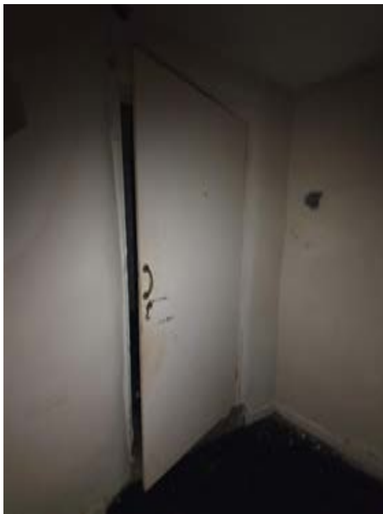
Photo018 – B02 - Basement Hall and Bottom of Stair - Door DB6
