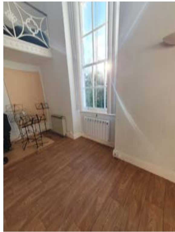
Photo347 – F05 - Meeting Room - Window WF3
