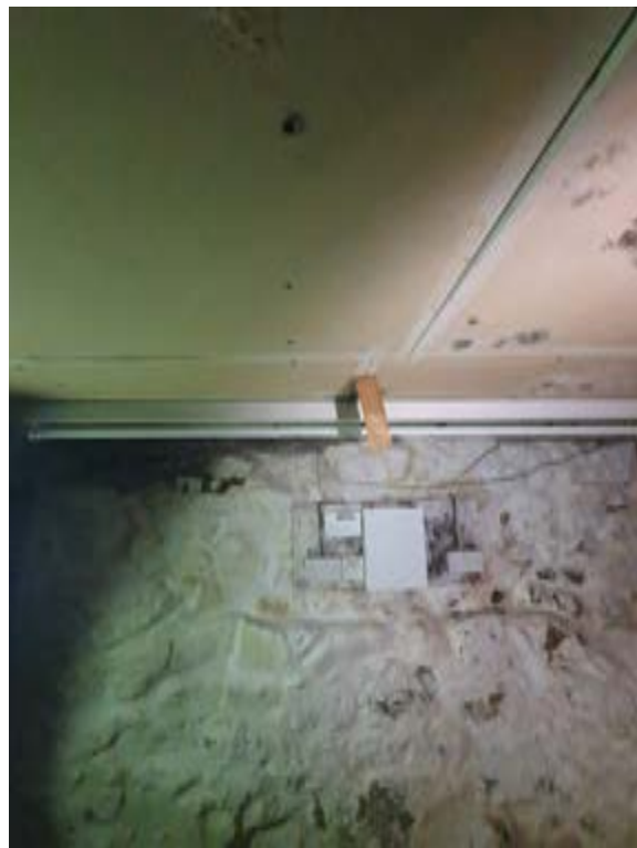
Photo044 – B03 - Basement Room 1
