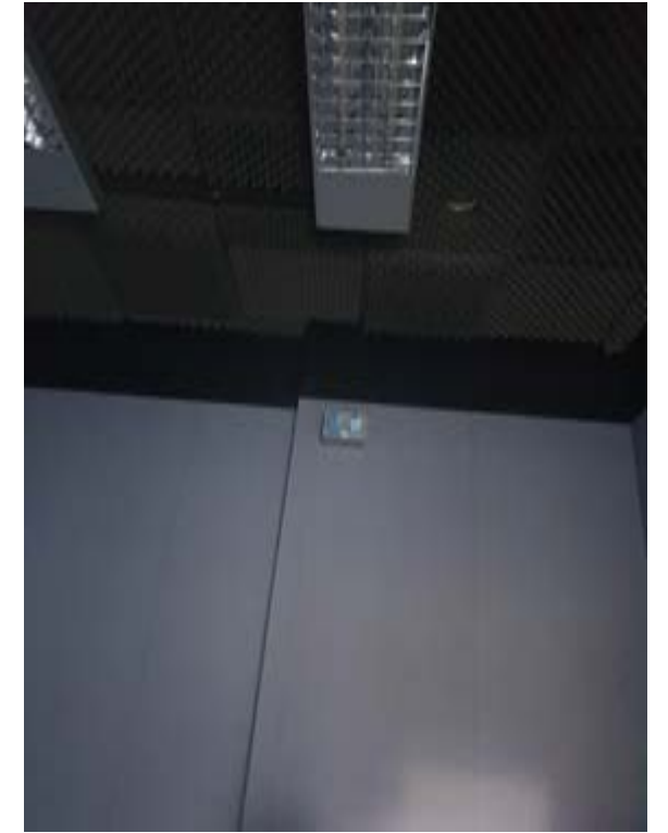
Photo247 – G05 - Storage - Wall between G045 and G04a to be removed.
