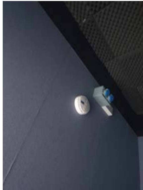
Photo244 – G05 - Storage - Wall between G045 and G04a to be removed.
