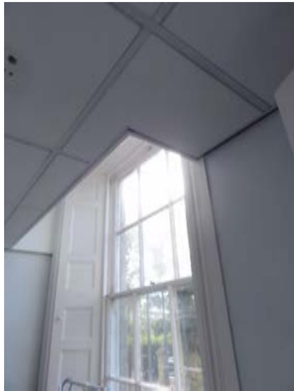
Photo228 – G04a - Lobby - Window WG7. Suspended ceiling to be removed.
