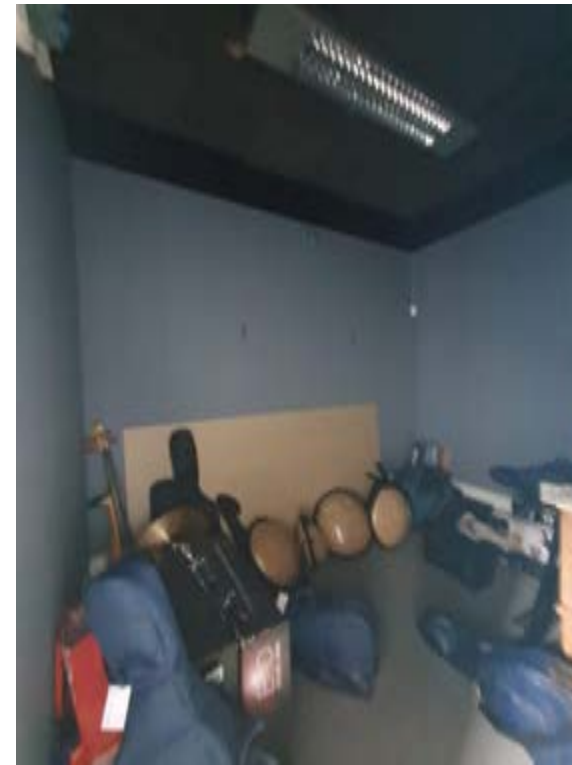
Photo238 – G05 - Storage - Wall between G045 and G04a to be removed.
