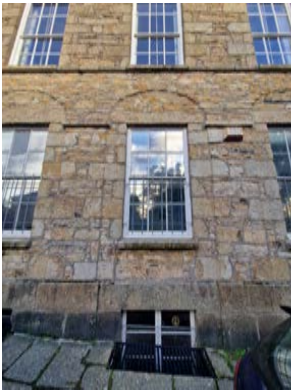
Photo362 – External - Windows WB2, WG6, WG7, WG8, WF3, WF4 and WF5
