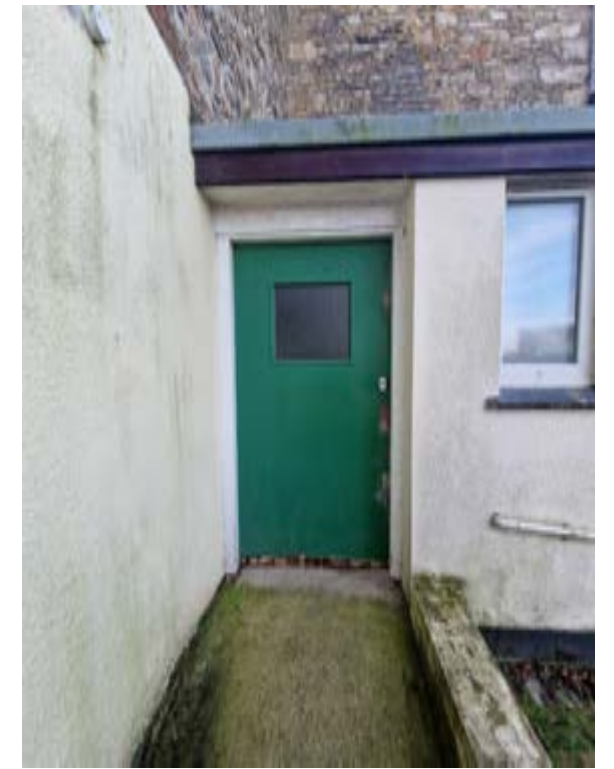
Photo359 – External - Door DG9 (To be removed and replaced)
