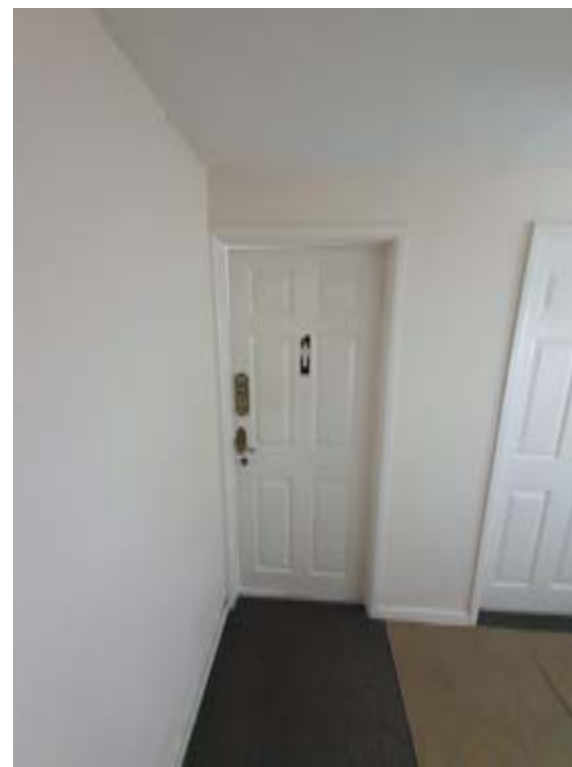
Photo286 – G09 - Entry Lobby - Doors DG23 and DG25 (To be removed). Layout to be reconfigured.
