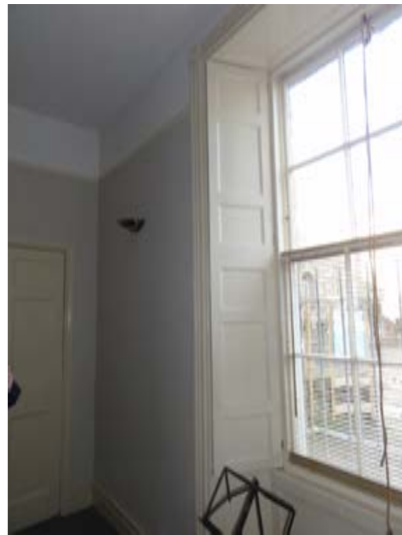
Photo132 – G01 - Office 1 - Window WG1 and Door DG5
