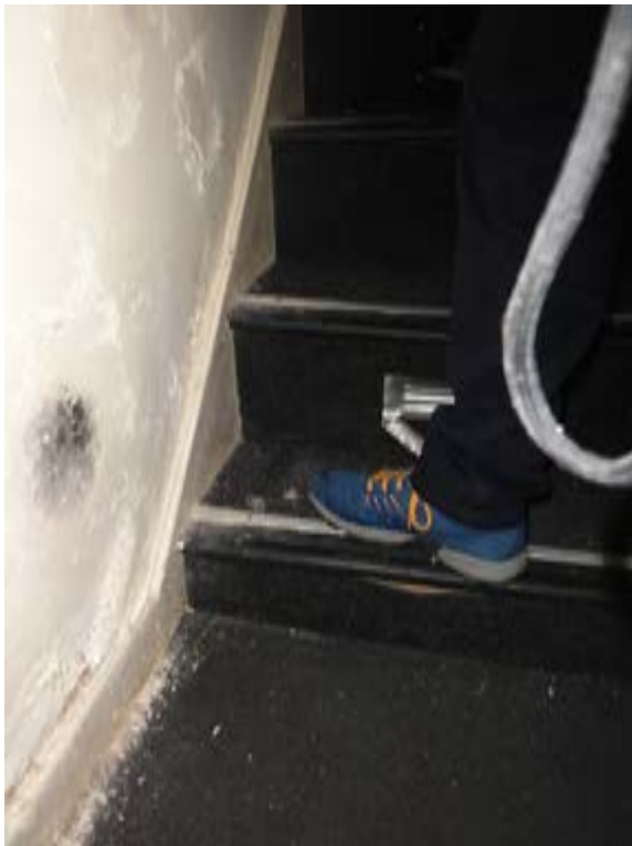
Photo026 – B02 - Basement Hall and Bottom of Stair
