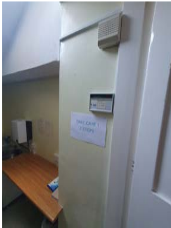
Photo267 – G07 - Kitchen 1 - Door DG14
