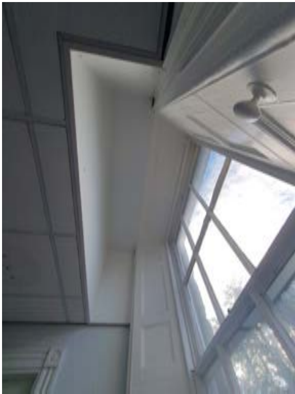
Photo218 – G04a - Lobby - Window WG7 - Suspended ceiling to be removed.
