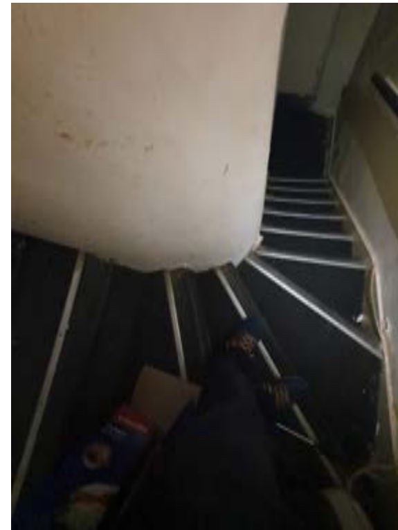
Photo007 – B01 - Top of Basement Stair
