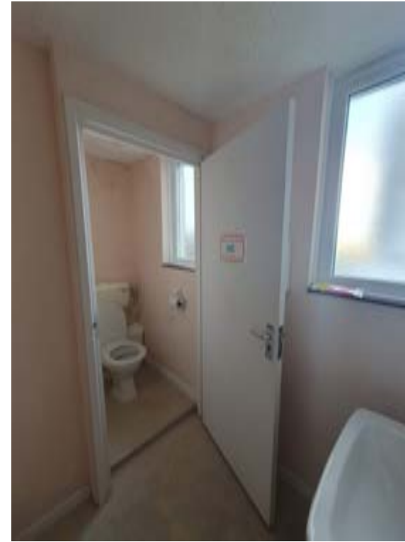
Photo293 – G10 - WC 2 - Windows WG3 and WG4. Door DG26 (To be removed). Layout to be reconfigured.
