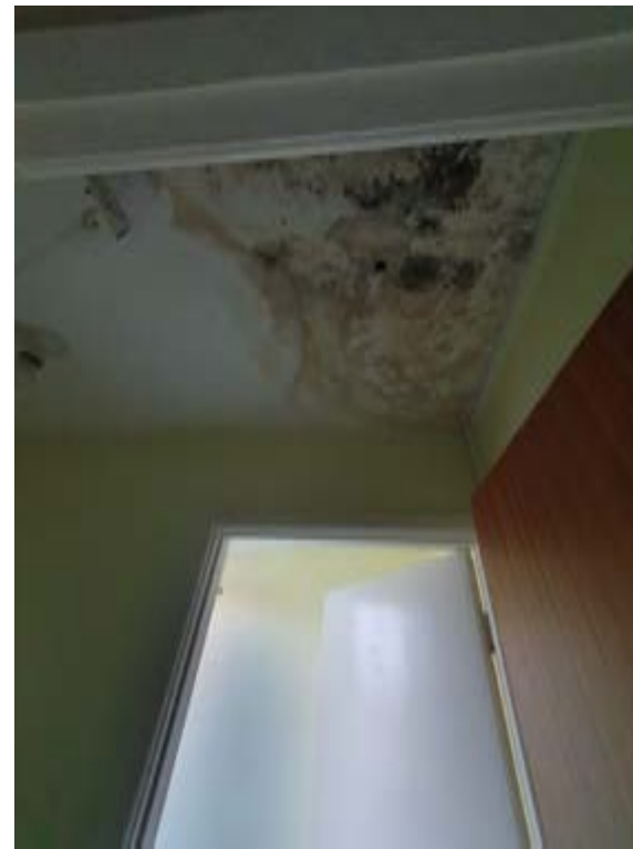
Photo285 – G08 - WC1 - Doors DG12 and DG13
