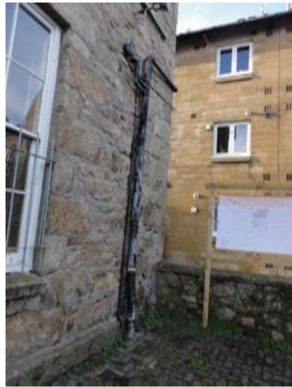
Photo379 – External - Window WG1
