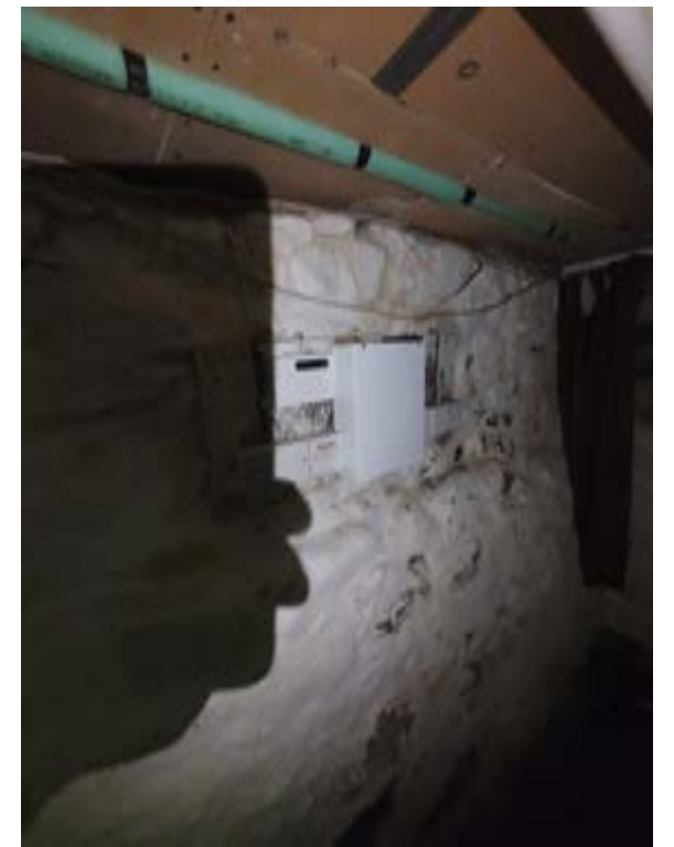
Photo048 – B03 - Basement Room 1
