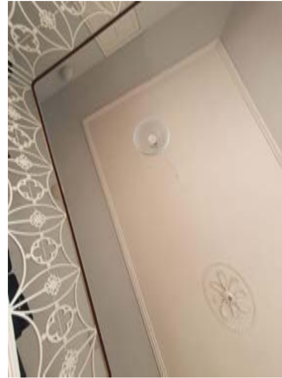
Photo341 – F05 - Meeting Room - Balcony Above
