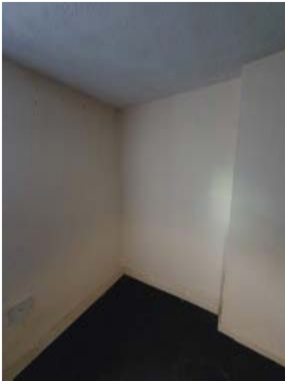
Photo066 – B04 - Basement Room 2
