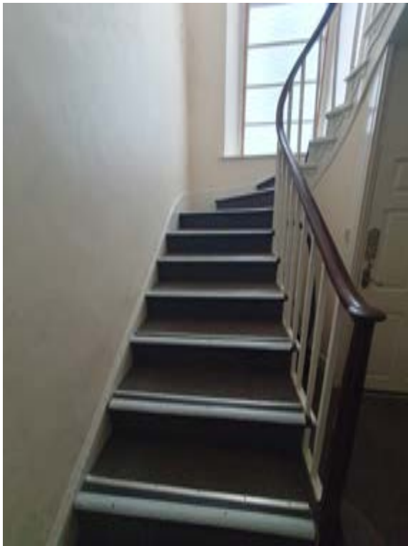
Photo154 – G03 - Ha11 1 and bottom of stair - Window WF2
