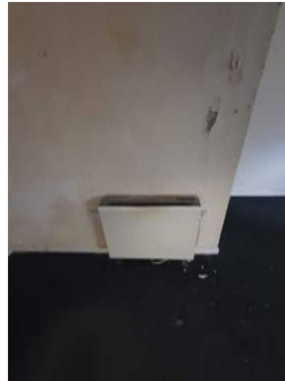
Photo078 – B04 - Basement Room 2
