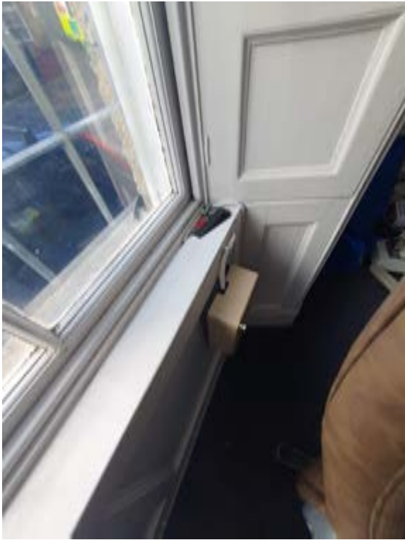
Photo205 – G04 - Office 2 - Window WG8 and shutter
