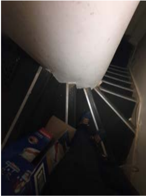
Photo009 – B01 - Top of Basement Stair
