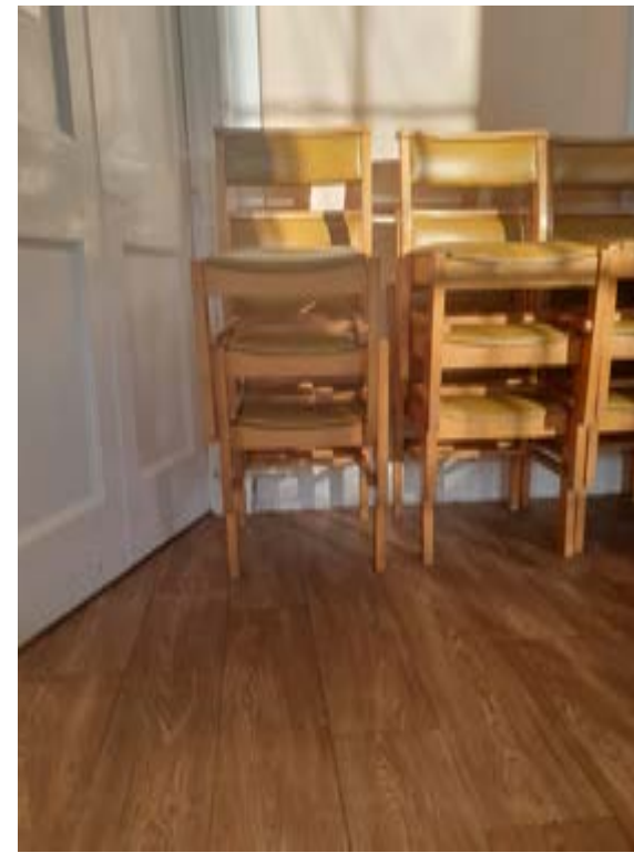
Photo349 – F05 - Meeting Room - Door DF1
