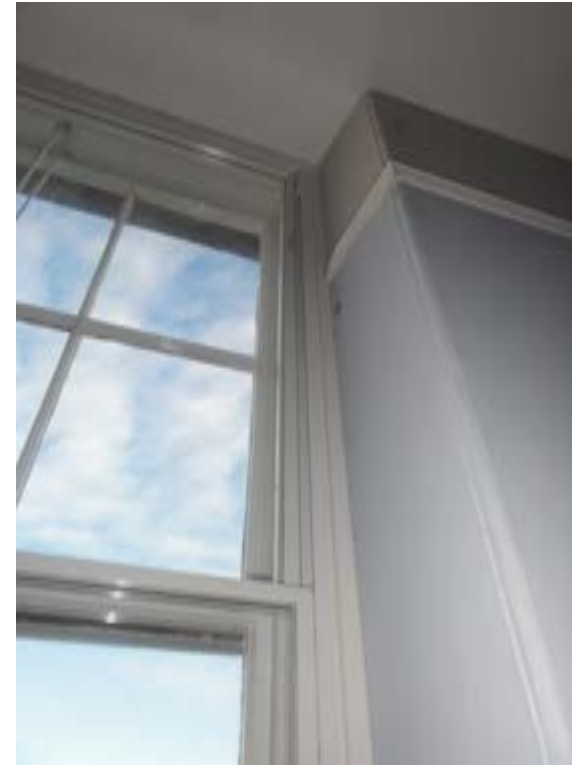
Photo325 – F02 - Office 3 - Window WF1 with Secondary Glazing.
