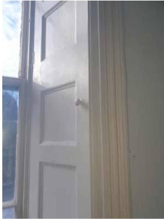
Photo227 – G04a - Lobby - Window WG7 and shutter
