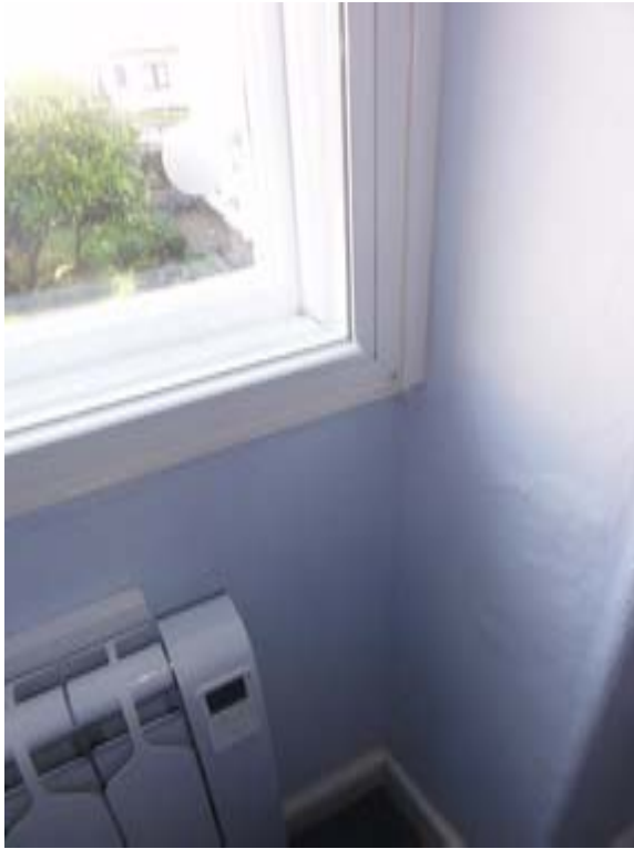
Photo321 – F02 - Office 3 - Window WF1 with Secondary Glazing.
