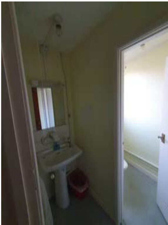
Photo281 – G08 - WC1 - Doors DG12 and DG13
