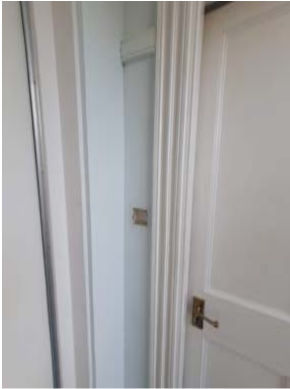
Photo225 – G04a - Lobby - Doors DG21 and DG22 (To be removed)
