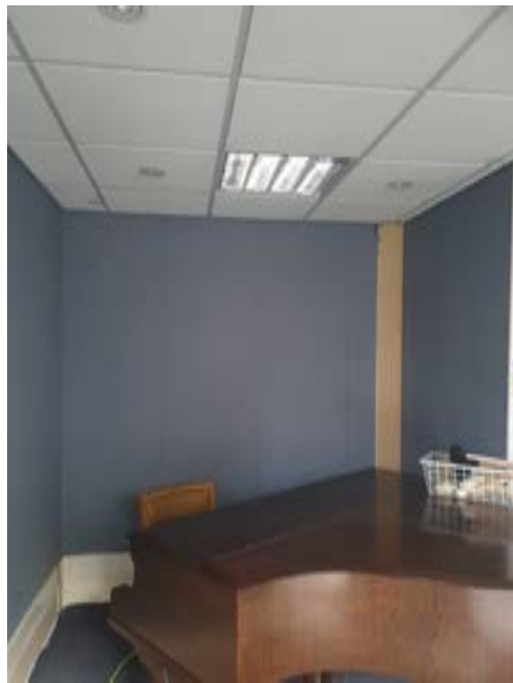
Photo252 – G06 - Office 3 - Suspended ceiling to be removed.
