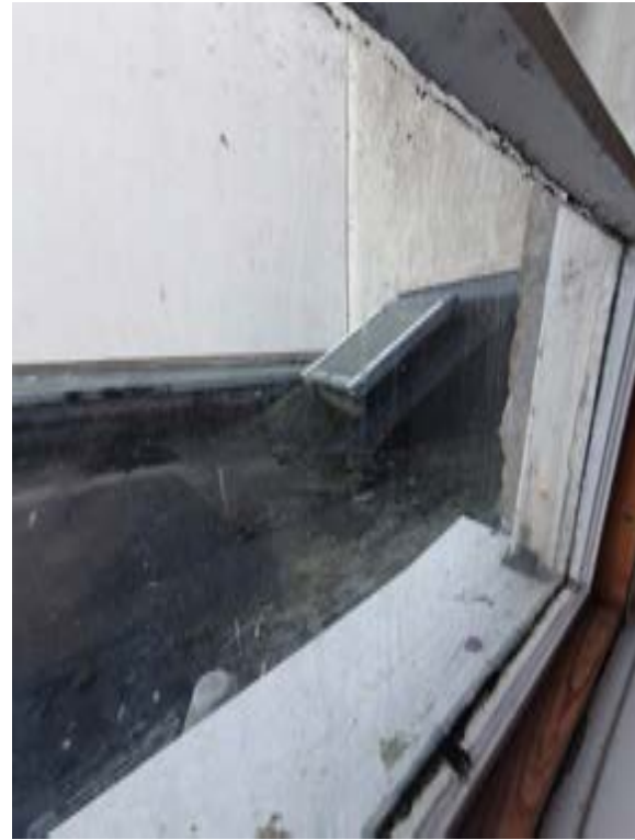
Photo171 – G03 - Ha11 1 - Window WF2 and Roof Light RF1
