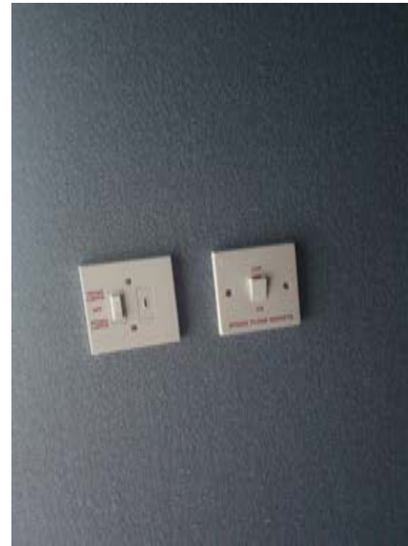
Photo246 – G05 - Storage - Wall between G045 and G04a to be removed.
