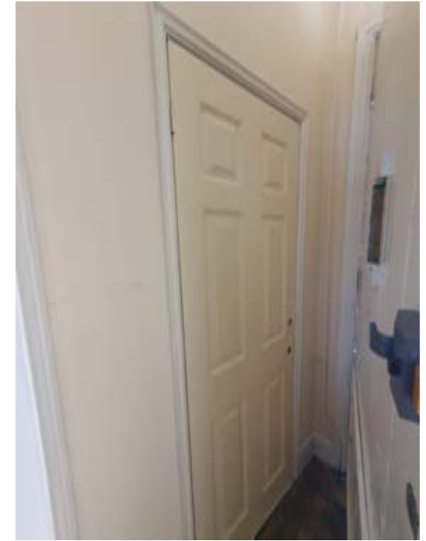
Photo143 – G02 - Entry - Doors DG1 and DG2
