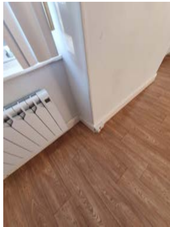
Photo340 – F05 - Meeting Room - Window WF3
