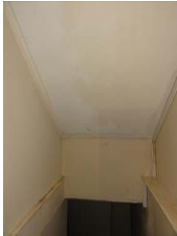
Photo028 – B02 - Basement Hall and Bottom of Stair
