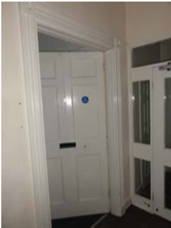
Photo186 – G03 - Ha11 1 - Doors DG3 and DG6
