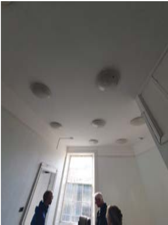
Photo208 – G04 - Office 2 - Window WG8 and Door DG17
