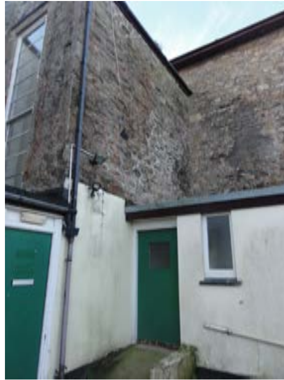
Photo373 – External - Windows WG4 and WF2 and Doors DG9 and DG11
