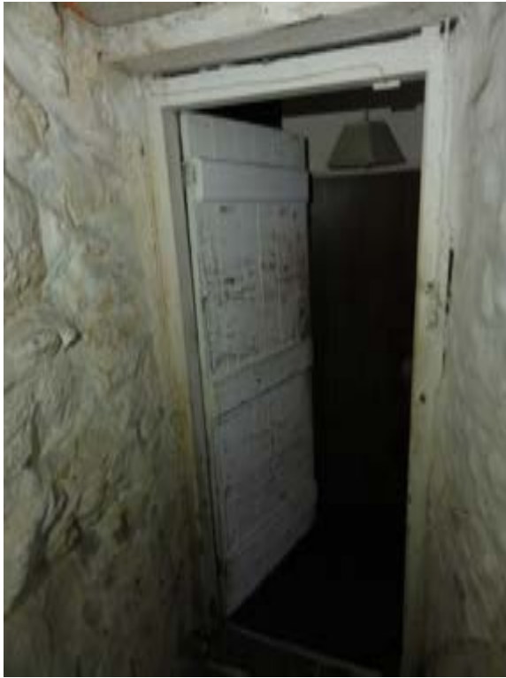
Photo041 – B03 - Basement Room 1 - Door DB6
