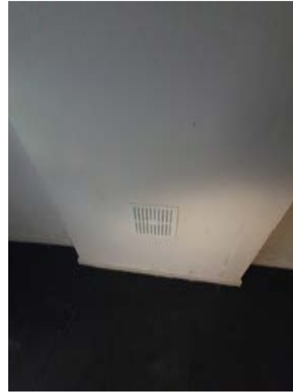
Photo077 – B04 - Basement Room 2
