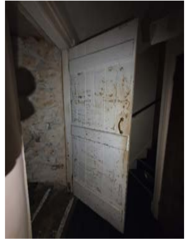
Photo023 – B02 - Basement Hall and Bottom of Stair - Door DB6
