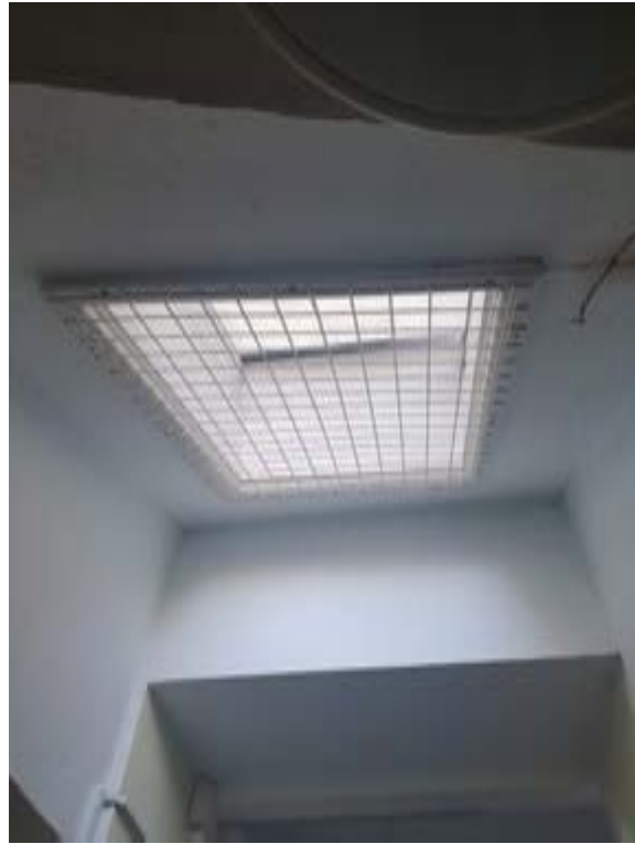
Photo275 – G07 - Kitchen 1 - Roof Light RL1
