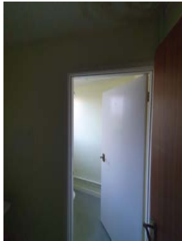
Photo283 – G08 - WC1 - Doors DG12 and DG13
