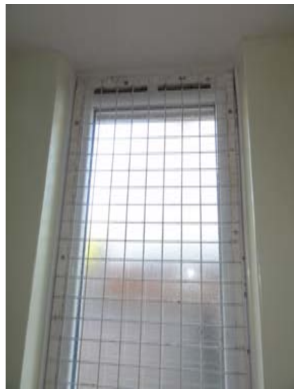
Photo284 – G08 - WC1 - Window WG5
