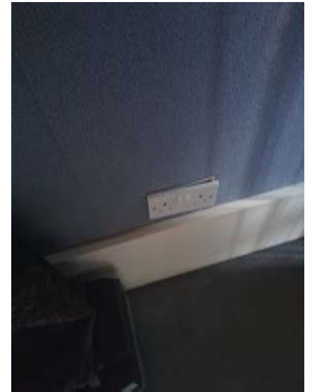
Photo248 – G05 - Storage - Wall between G045 and G04a to be removed.
