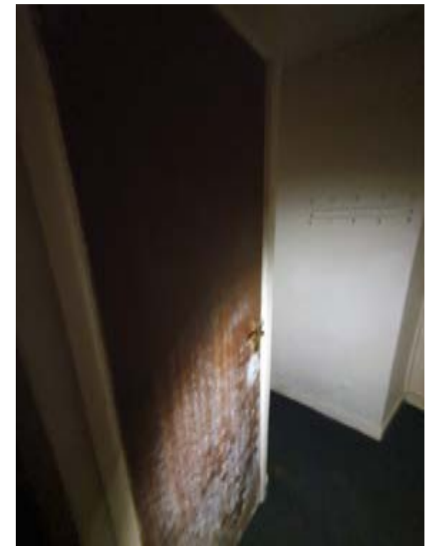
Photo016 – B02 - Basement Hall and Bottom of Stair - Door DB1
