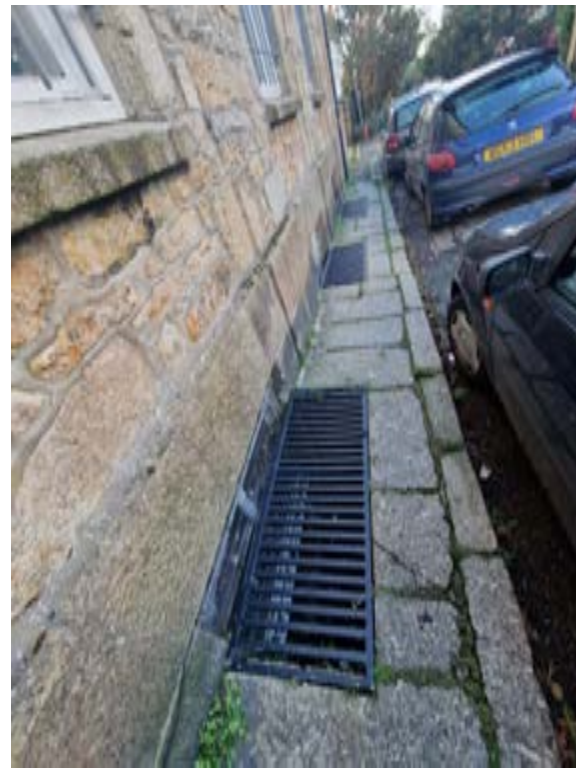
Photo363 – External - Windows WG6, WG7 and WG8 and grilles to Basement Windows
