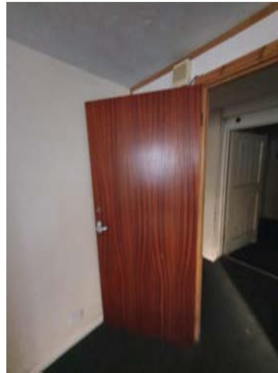
Photo070 – B04 - Basement Room 2 - Door DB4
