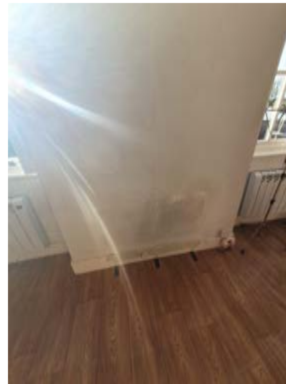
Photo342 – F05 - Meeting Room - Windows WF4 and WF5
