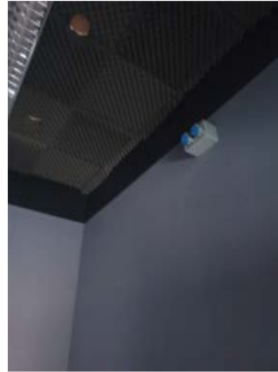
Photo245 – G05 - Storage - Wall between G045 and G04a to be removed.
