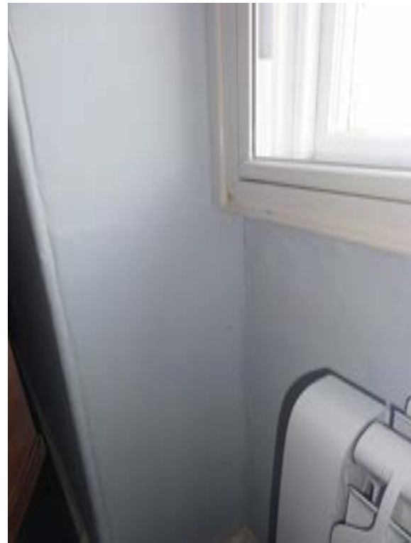
Photo324 – F02 - Office 3 - Window WF1 with Secondary Glazing.
