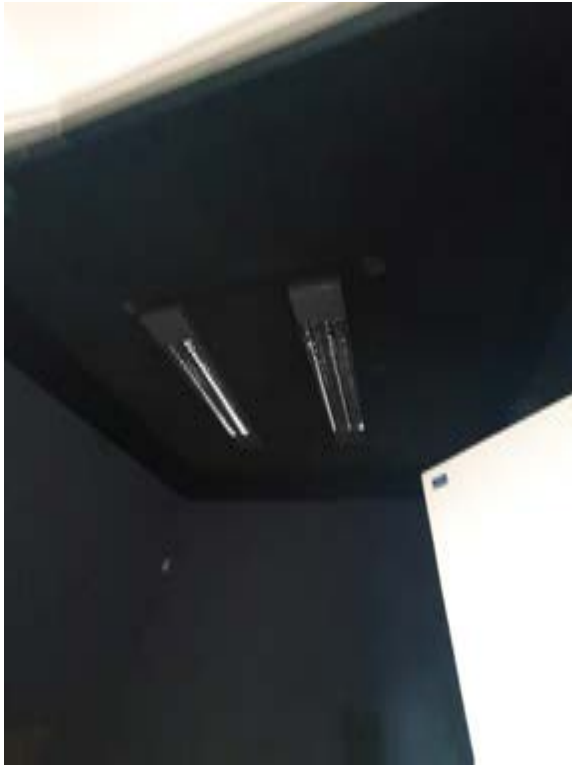
Photo241 – G05 - Storage - Wall between G045 and G04a to be removed.
