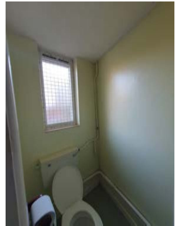
Photo287 – G08 - WC1 - Window WG5
