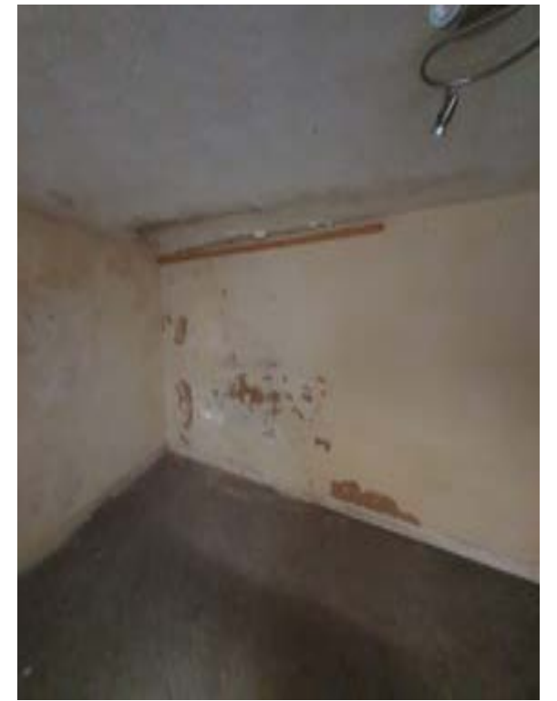
Photo095 – B05 - Basement Room 3
