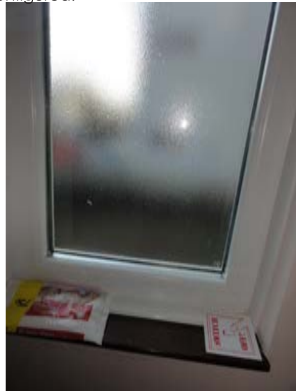
Photo292 – G10 - WC 2 - Window WG4
