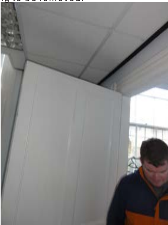
Photo258 – G06 - Office 3 - Door DG22 (To be removed)
