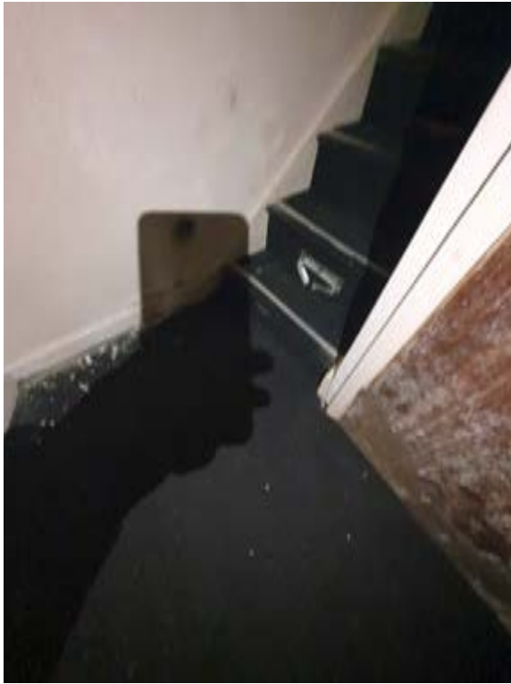
Photo025 – B02 - Basement Hall and Bottom of Stair
