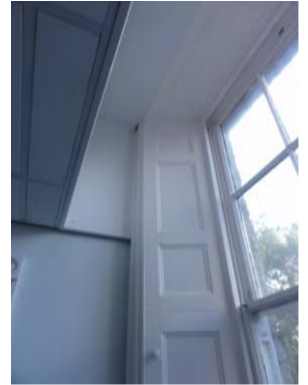
Photo239 – G04a - Lobby - Window WG7 and shutter
