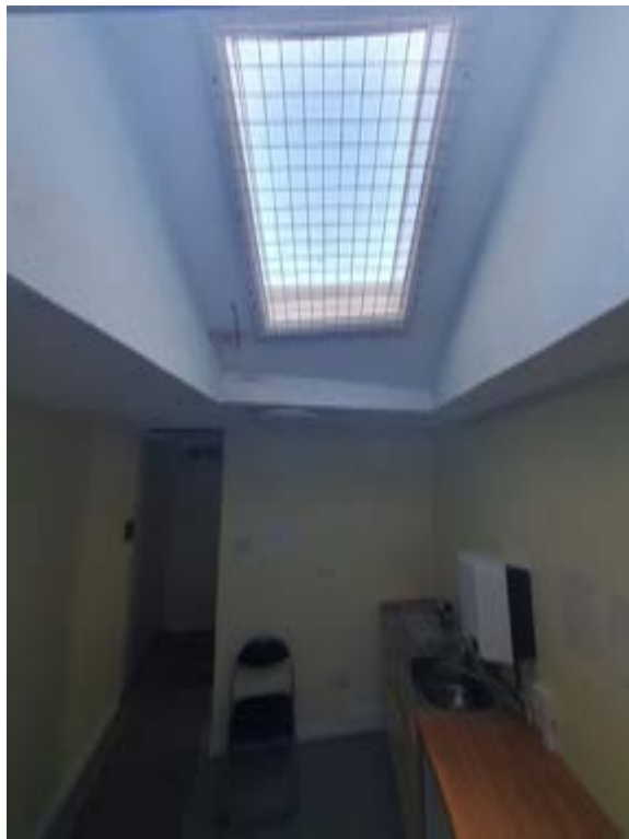
Photo269 – G07 - Kitchen 1 - Roof Light RL1
