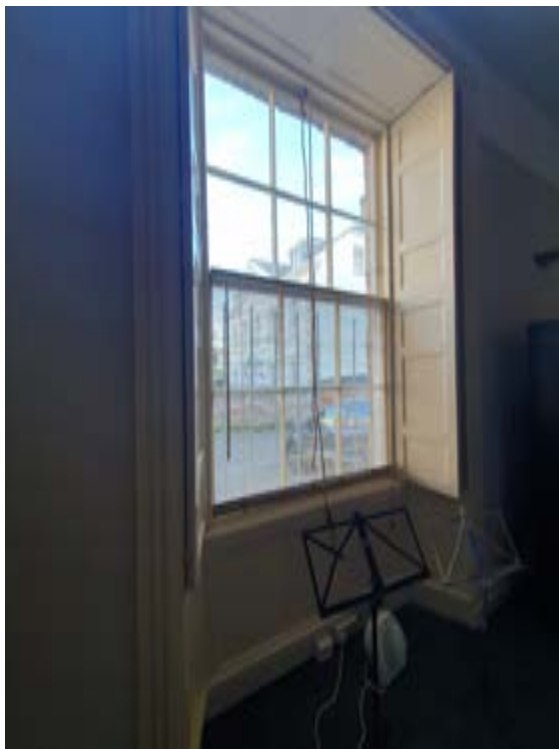
Photo122 – G01 - Office 1 - Window WG1
