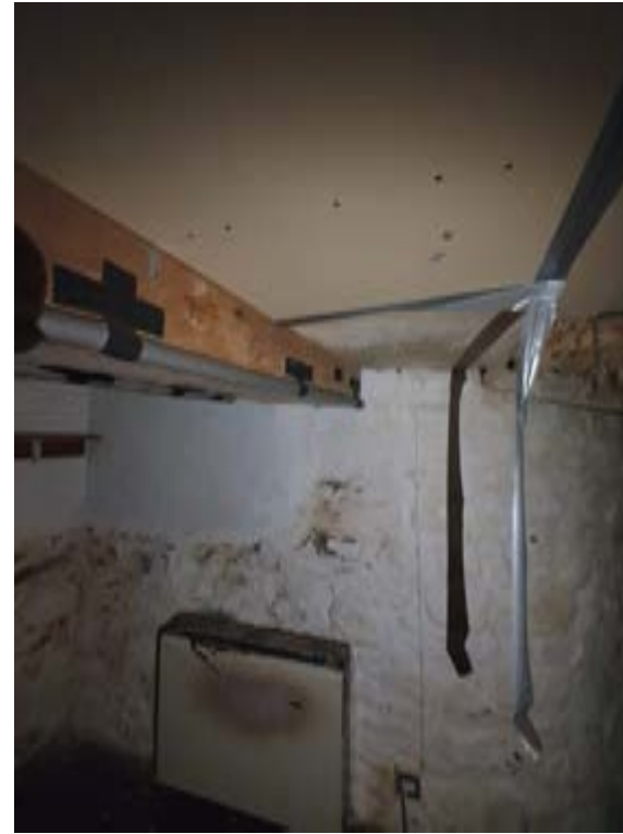
Photo045 – B03 - Basement Room 1
