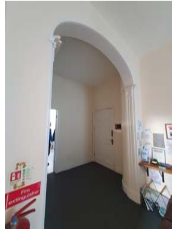
Photo309 – F01 - Landing - Doors DF4 and DF5
