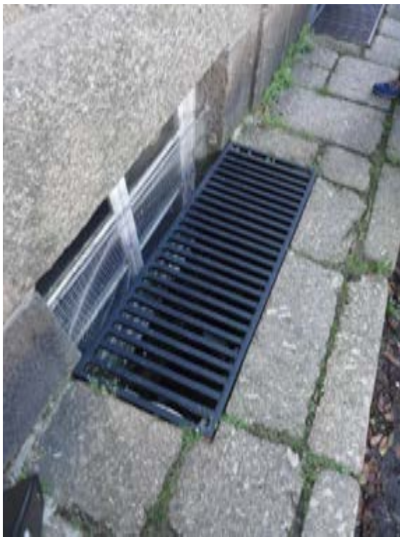
Photo378 – External - Window WB3
