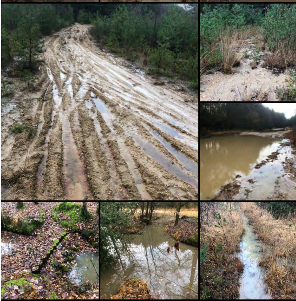
Significant ruts across sandy tracks showing turbid water displaced into adjacent areas.
