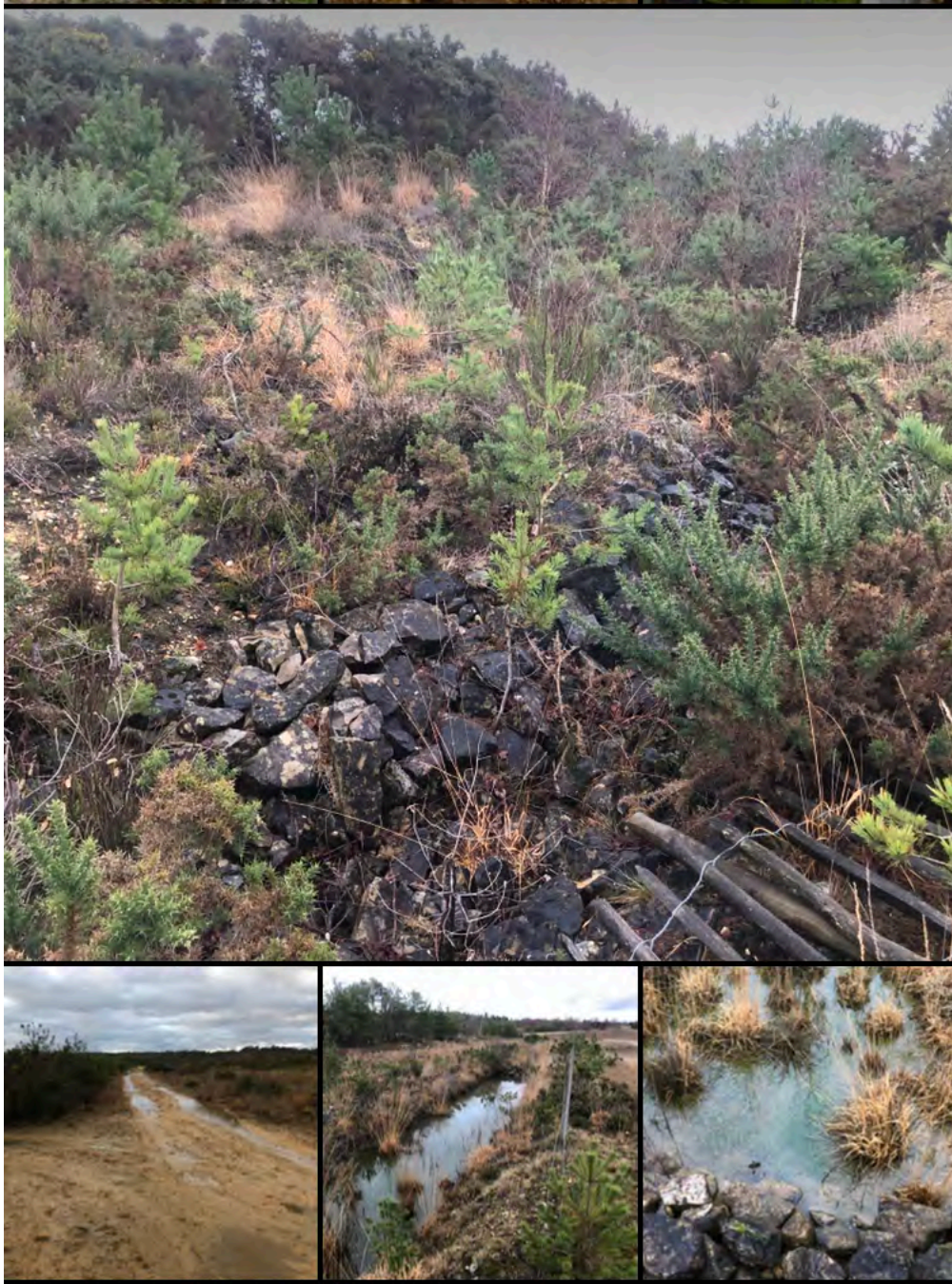
Stable and vegetated features by upper holding lagoon, also some eroding tracks in the vicinity
