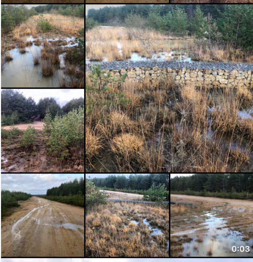
Functioning sediment traps with vegetation showing flow of turbid water downslope
