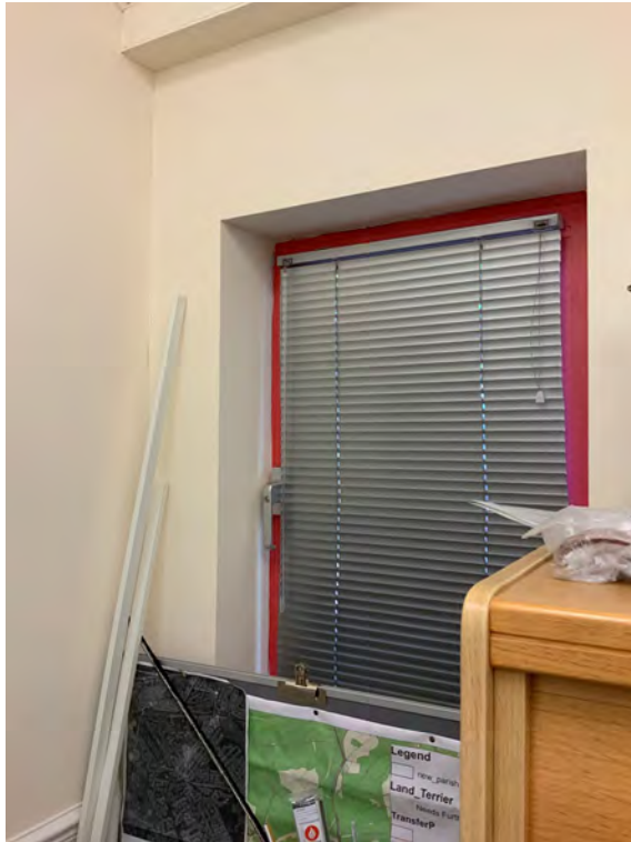
P95 Ben's Office – Open joints around window into wall joint
