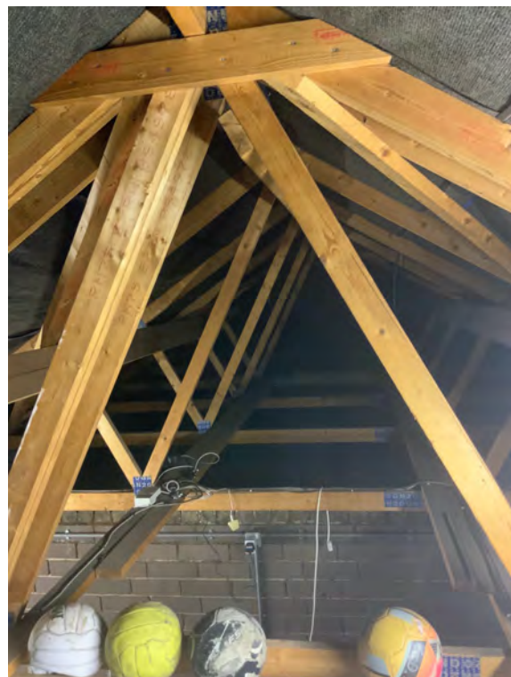
P170 Roof space above kitchen – roof structure
