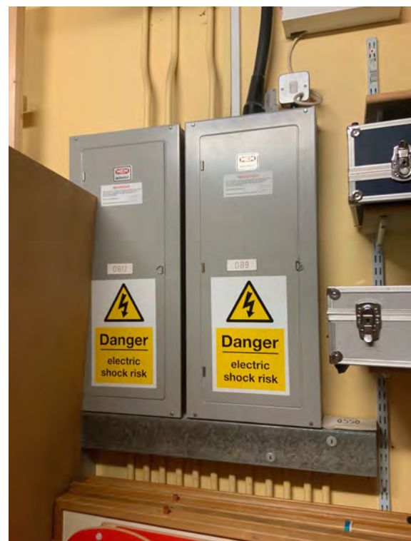
P178 The Point – Distribution Board in left hand store
