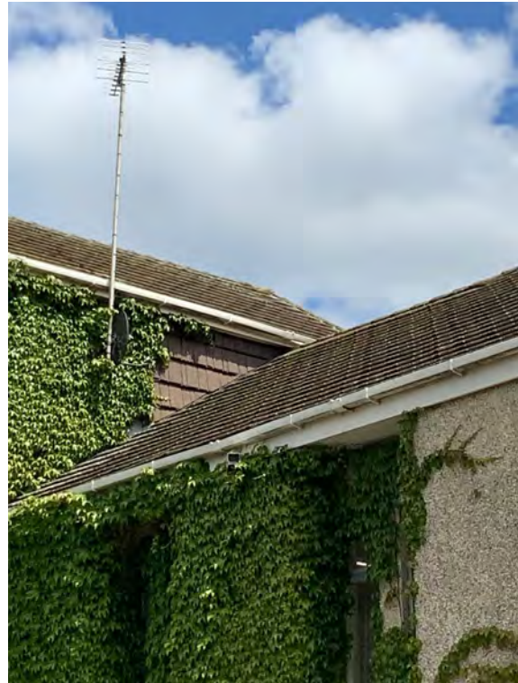
P10 Gutter to roof above the bar store requires repair just above ridge to the function room.
