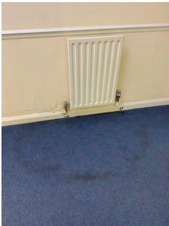
P97 Upper Office Lobby – Leak to radiator and localised deteriorated finishes
