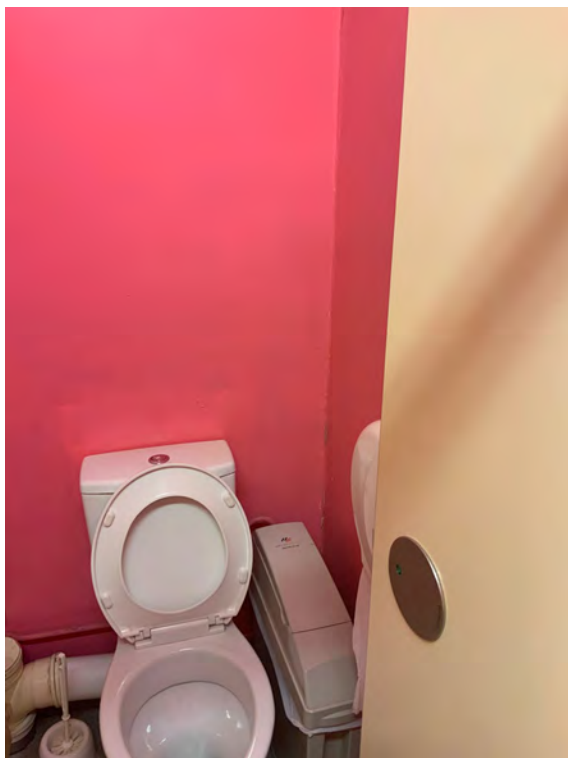
P84 The Point, Ladies Toilet. Cracking to the joint between the walls in the right hand cubicle
