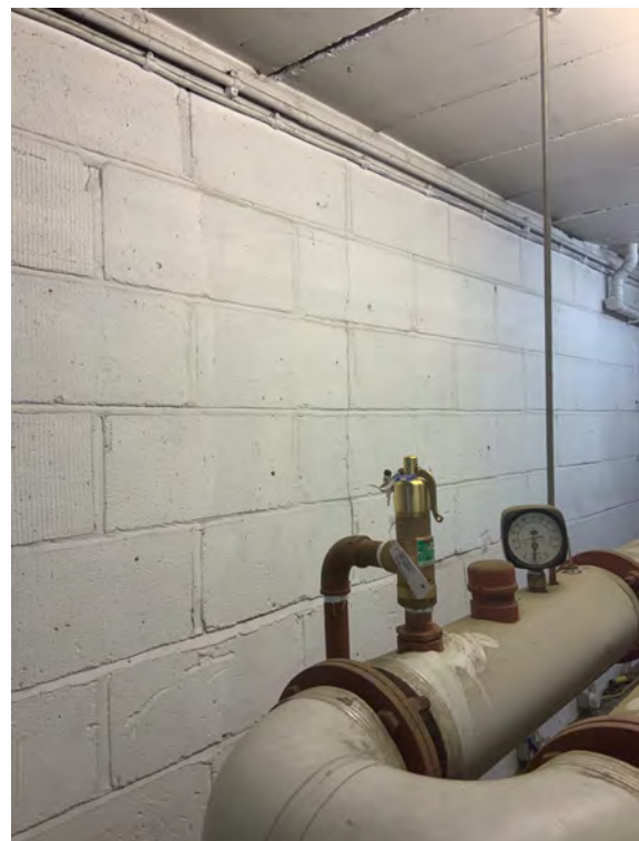
P106 Boiler Room – Hairline crack behind the boiler. These cracks are replicated at approx. 1m intervals along the wall
