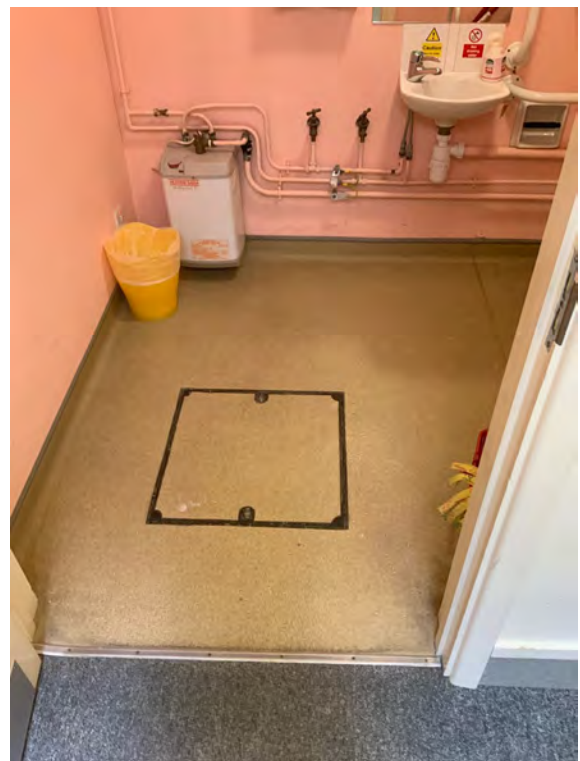
P118 RVS Accessible Toilet – Manhole set into toilet floor
