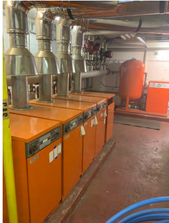
P184 Boiler room – Five boilers
