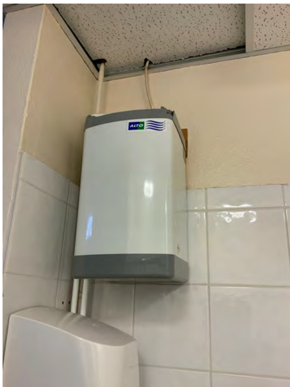
P185 Dressing Room 1 – Alto wall mounted water heater
