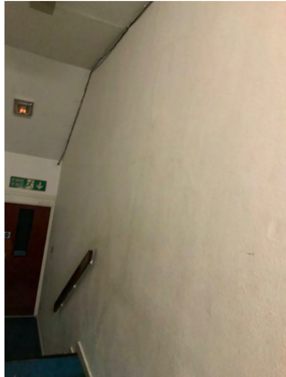
P100 Dressing Room Corridor – Floor to ceiling vertical cracking to top of stairs
