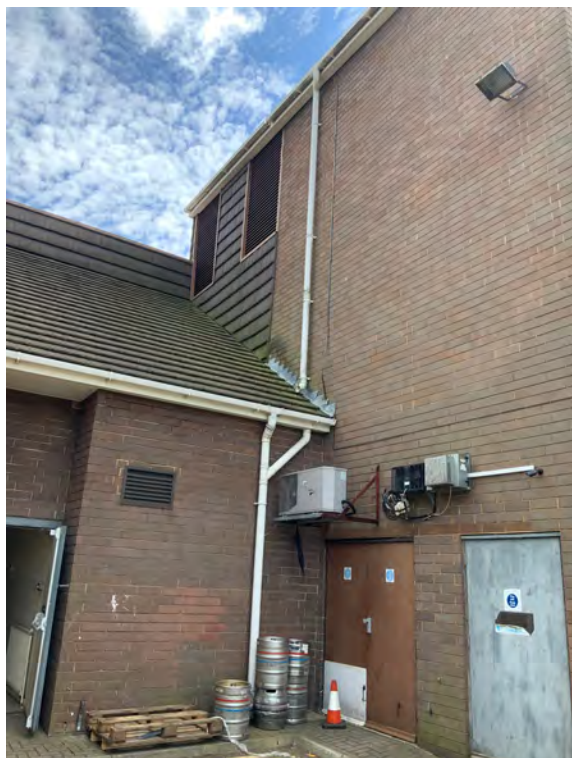
P27 North-west and north-east elevations, Downpipe from high level roof discharging to lower roof.
