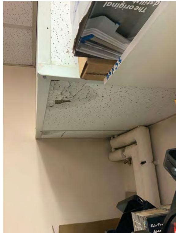
P38 Kitchen store – previous leak to base of extract housing
