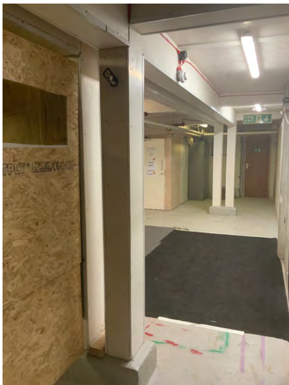
P113 Basement Stage Store – Supporting piers.
