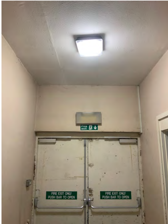
P74 Corridor from auditorium to outside – Cracking above external fire doors and to left hand wall
