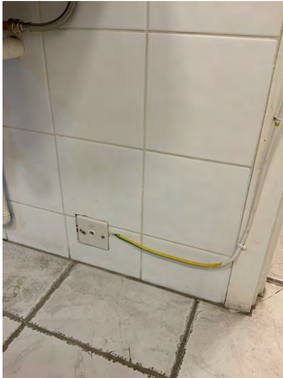
P179 Dressing Room 1 -Earth set into tiling beneath wash basin
