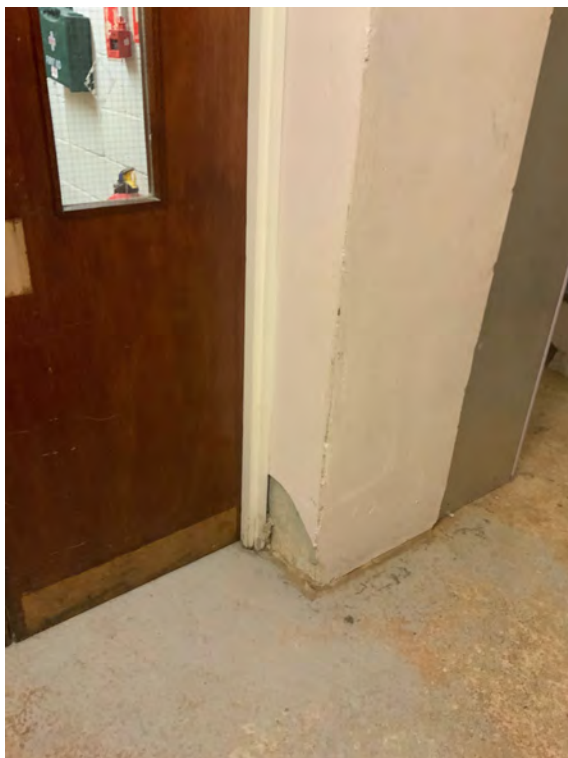
P109 Basement Main Lobby – Area of plaster missing from bottom of door and isolated areas of impact damage
