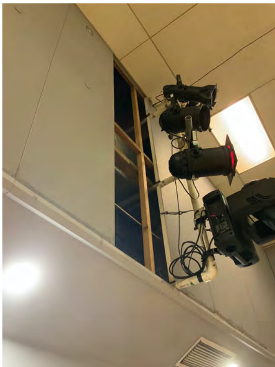
P88 Auditorium – acoustic panels to upper walls. The walls behind are blockwork.
