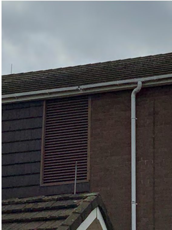
P9 Gap in gutter to north-east elevation of high level function room
