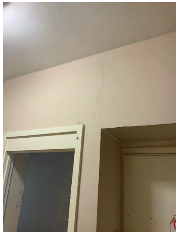
P73 Corridor from auditorium to outside - Crack to right hand wall between doors
