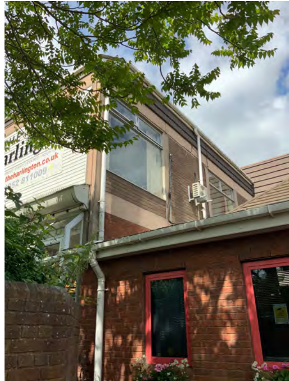
P6 Downpipes to right hand side of reception
