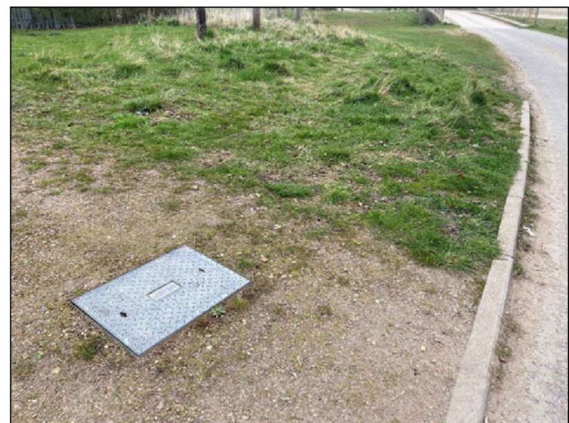
IMAGE 1 Existing primary incoming buried mains cold water stop valve / meter at site entrance (assumed - see spec.)
