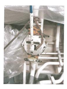
Defect 14/24 - Reweld/replace the Port Generator supply and return fuel pipe clamp bracket.
