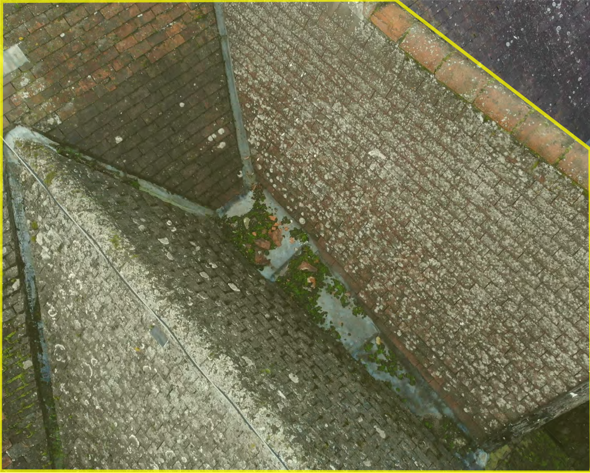
PHOTO 9 - CONCEALED VALLEY AND INNER ROOF SLOPE OVER MAIN STAIRCASE TO BE REPLACED AND RE-TILED RESPECTIVELY
