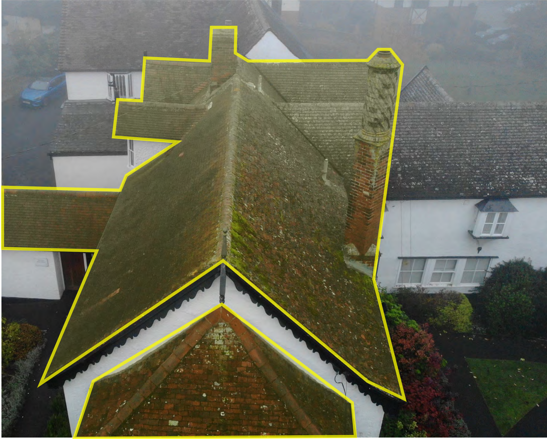
PHOTO 6 - COUNCIL CHAMBER ROOF AND CHIMNEY. NOTE: CONCEALED STUB GABLE TO BUSINESS SUITE TO REAR
