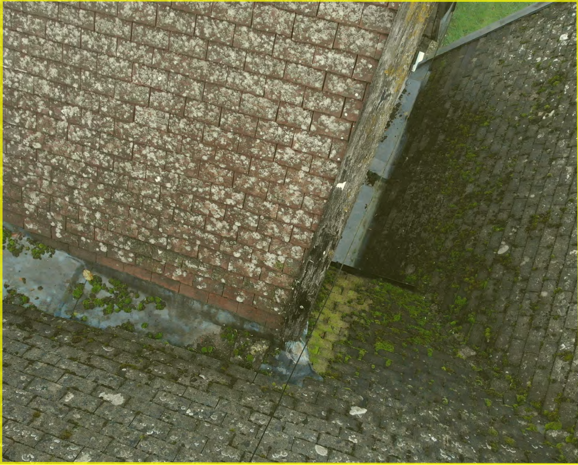
PHOTO 8 - CONCEALED VALLEY GUTTERS OVER MAIN STAIRCASE TO BE REPLACED.
