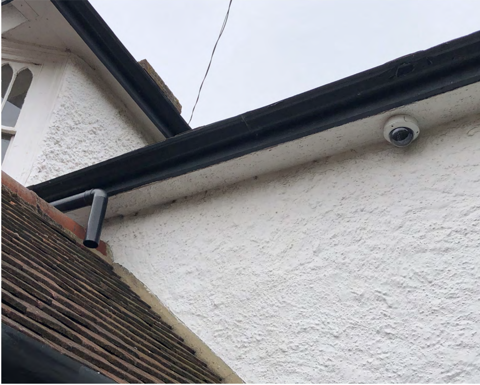
PHOTO 14 - CCTV ON EAVES TO BE RELOCATED, PROTECTED, MAINTAINED DURING THE WORKS.
