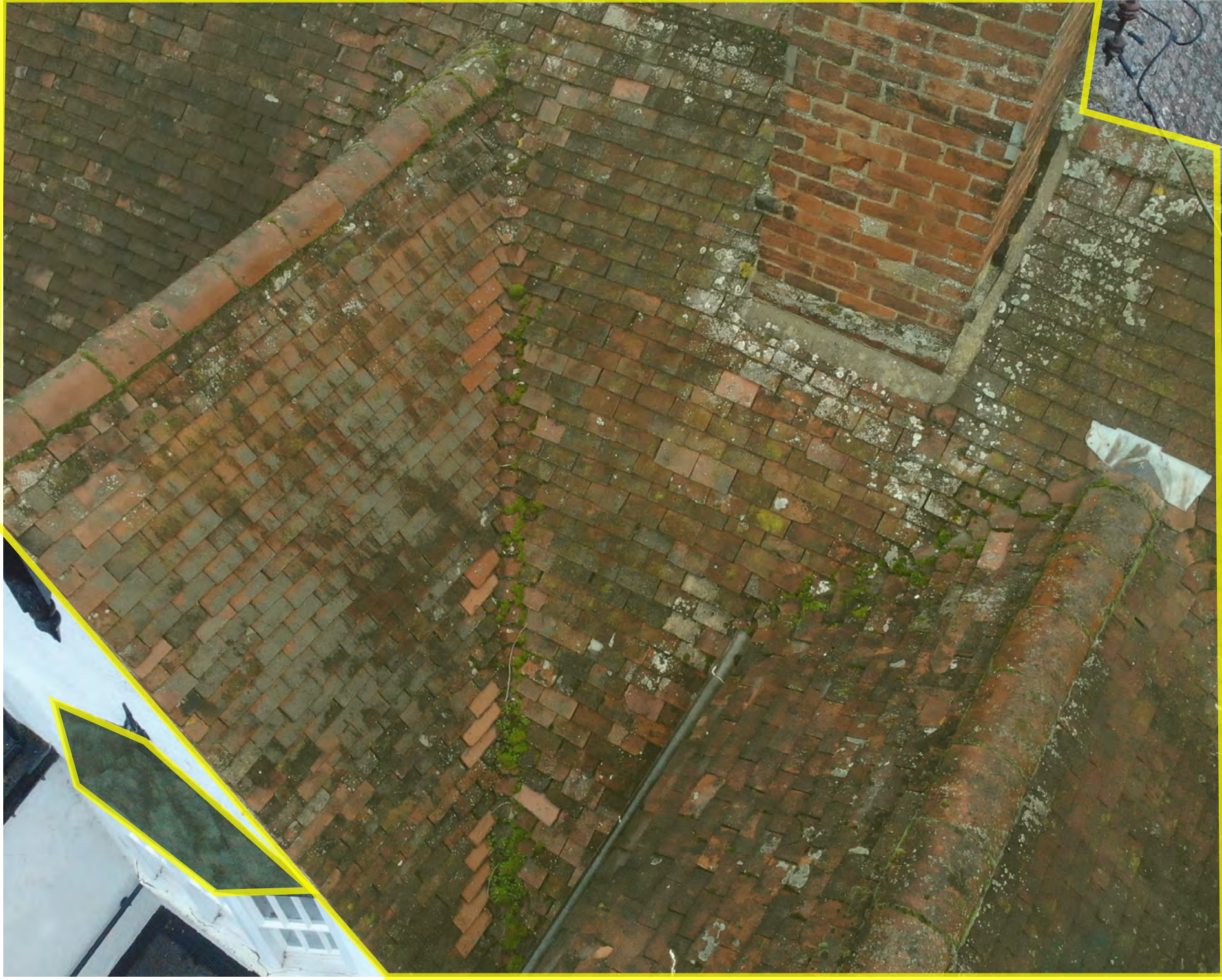
PHOTO 5 - SWEPT VALLEY TO WEST ELEVATION GABLE AND DORMER. NOTE ALSO ROOF TO ORIEL WINDOW.
