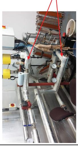
The steam hot water generation plant is to be removed from the plant room together with all pipework and fittings. This does not include the hot water distribution pipework.
