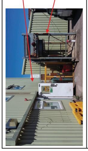
Hot water supply and return pipework to/from the new hot water generation plant to run along this wall towards the hot water distribution tie in points
