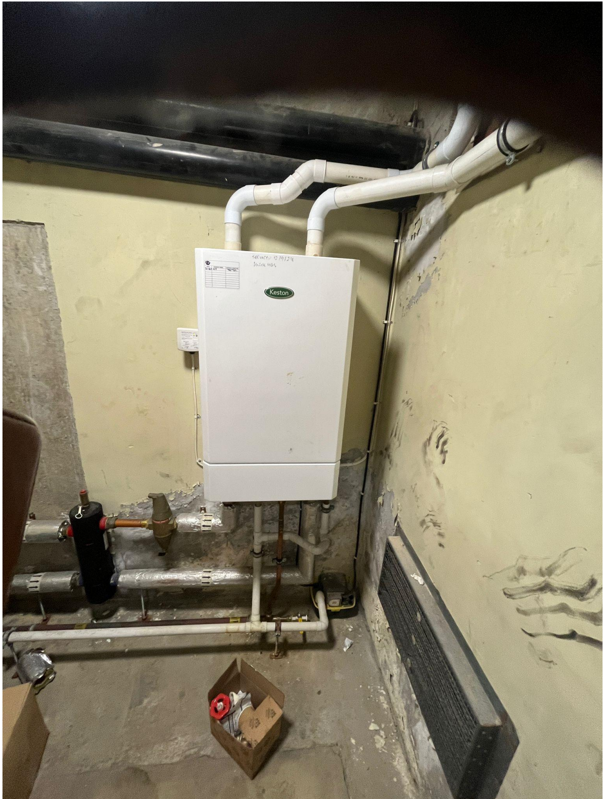
Wall Mounted Gas Boiler
