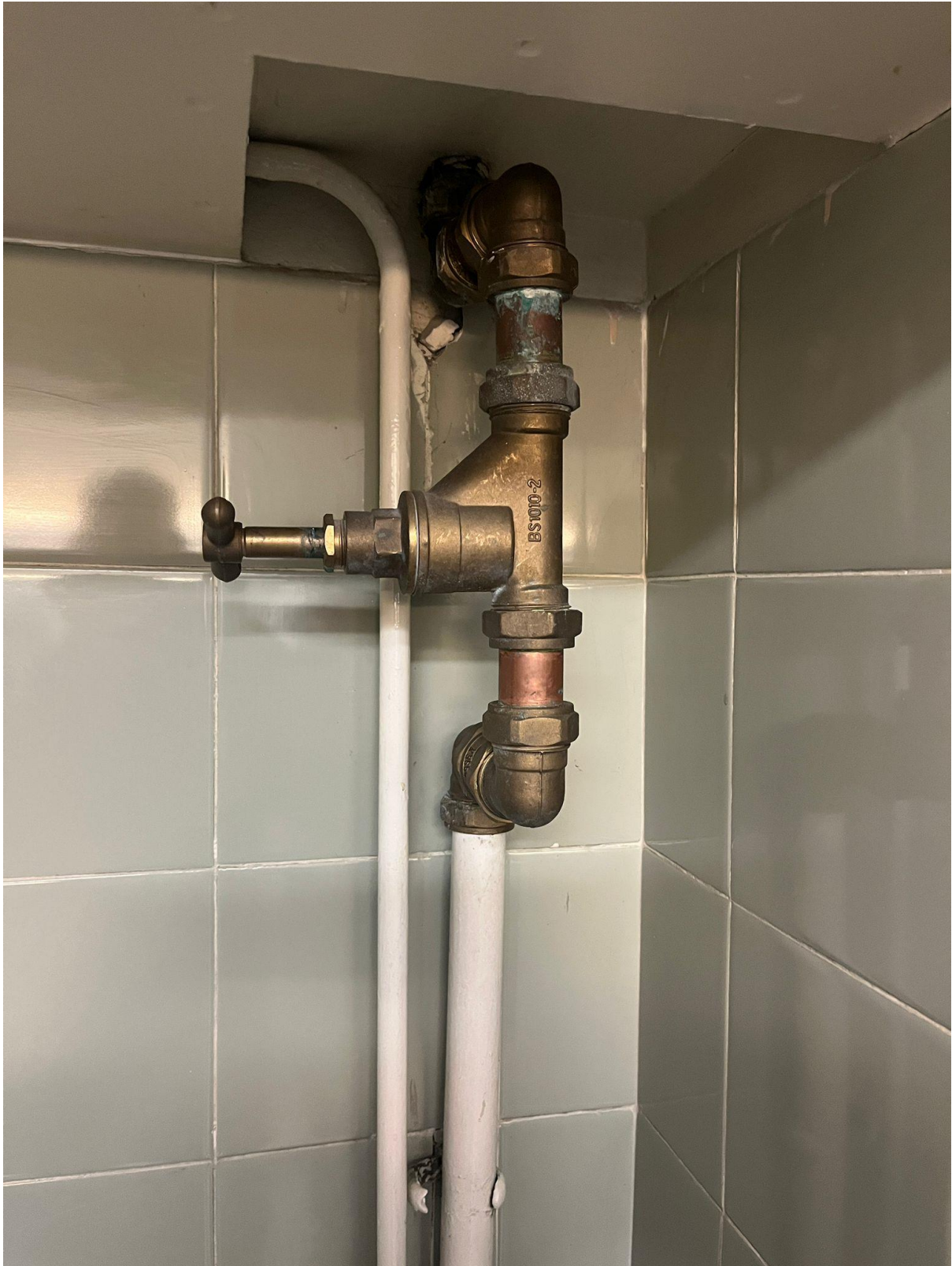
Mains Water Stop Cock (28mm) in Basement Ladies Toilets
