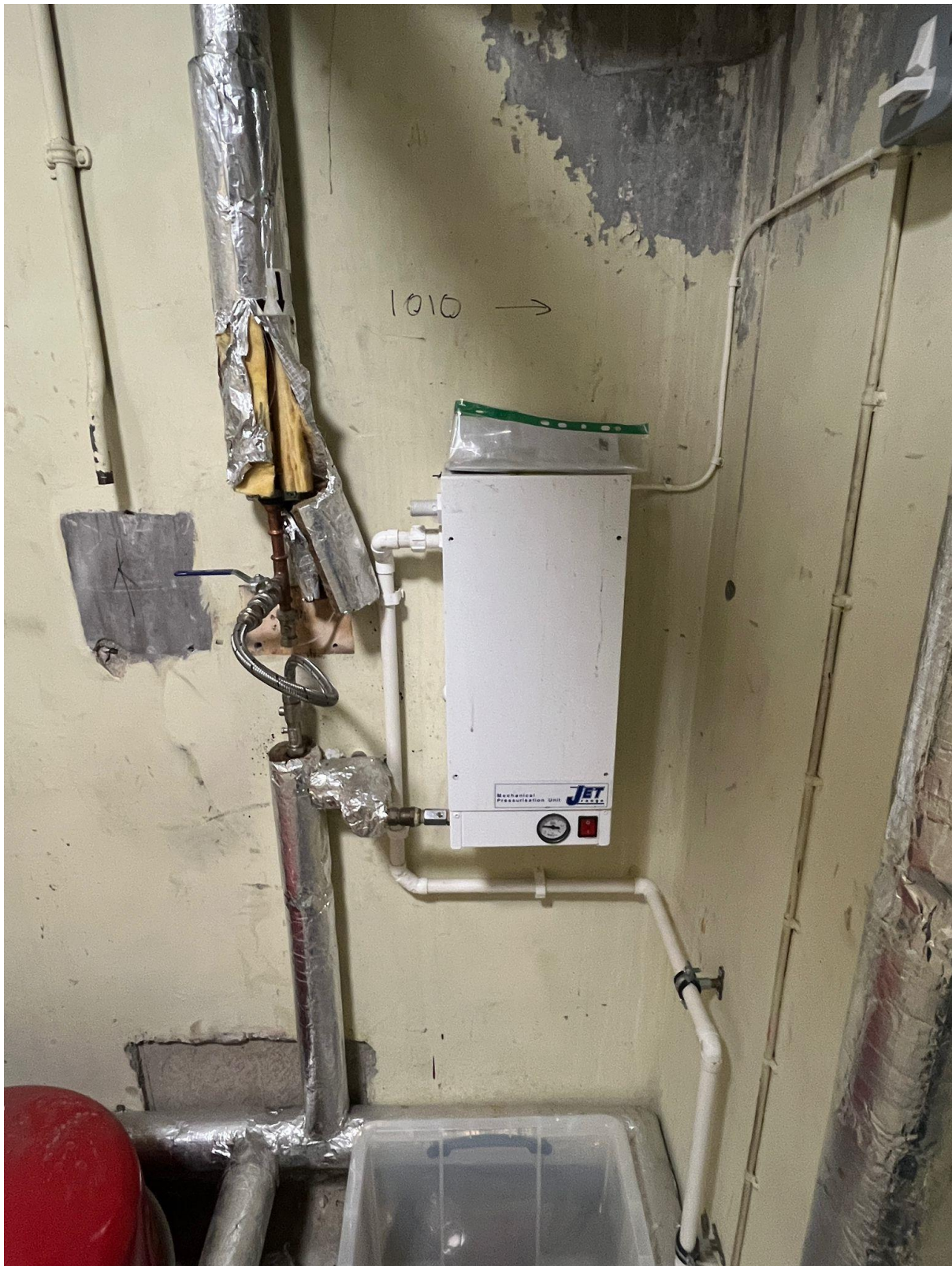
Heating System Pressurisation Unit
