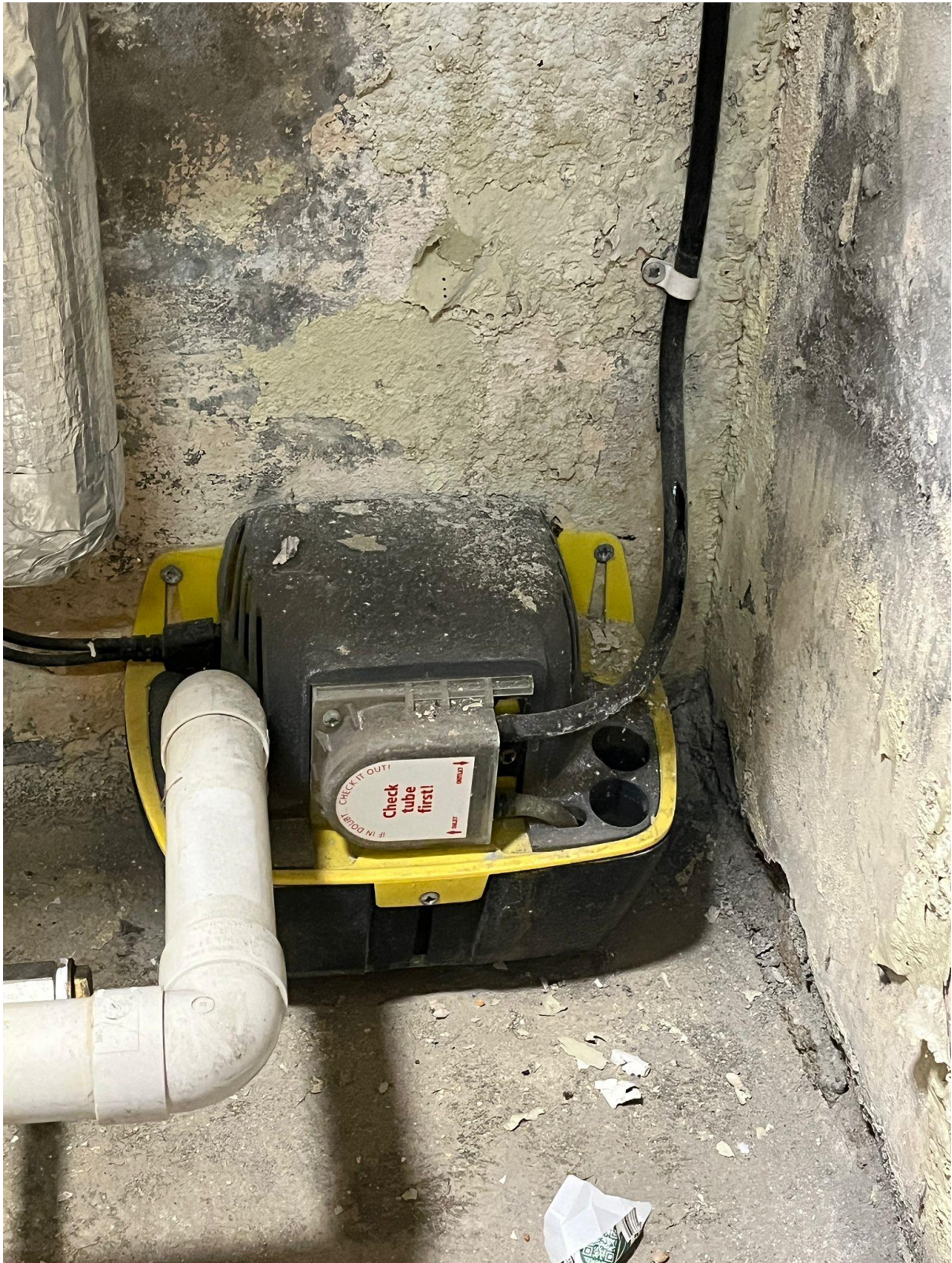
Boiler Condensate Pump
