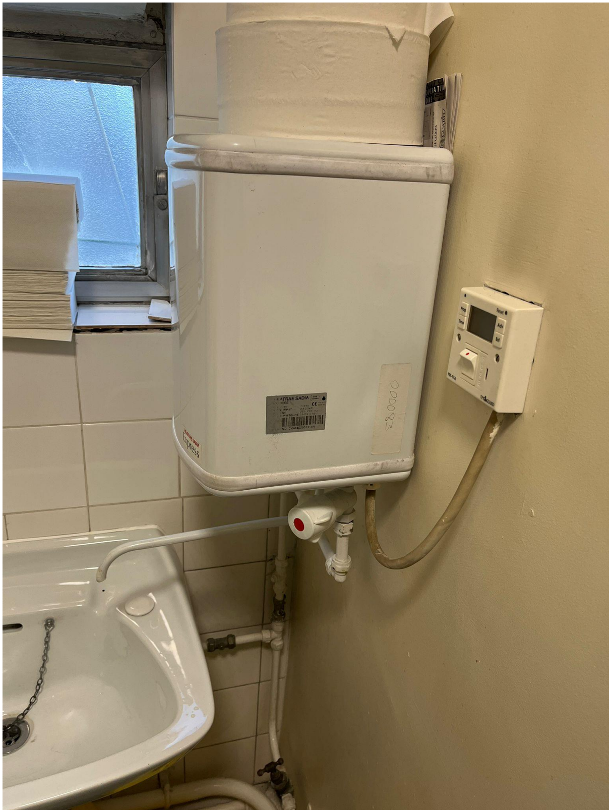
Point of Use Hot Water Heater in Ground Floor W.C.
