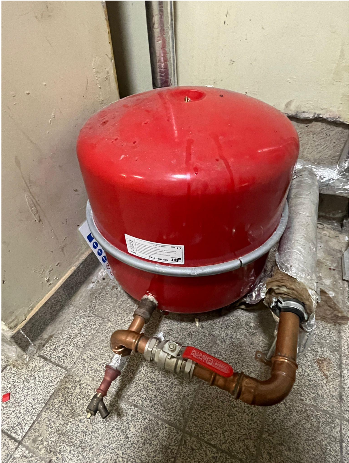
Heating Expansion Vessel
