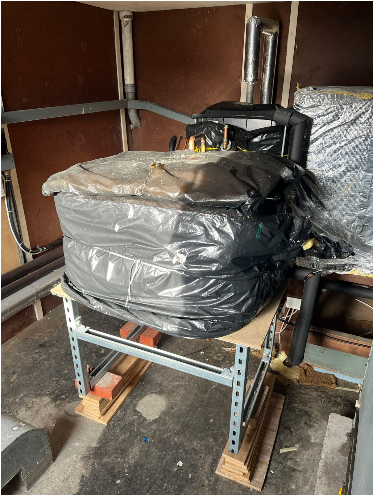
Cold Water Storage Tank in First Floor Roof Space
