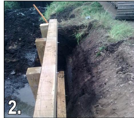
2. Structural timber headwall driven so that the top is at ground level.
