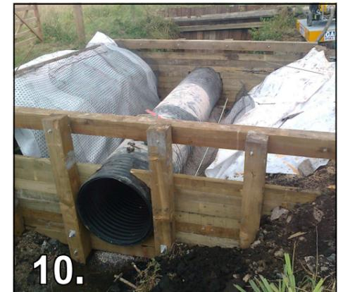
10. Geotextile laid under pipe. Pipe installed on bedding stone and headwall timbers cut around pipe. Bottom tie-bars installed and tightened
