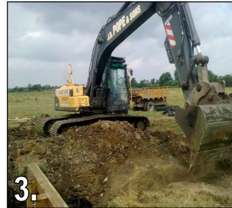
3. Excavating to remove old gateway and culvert.
