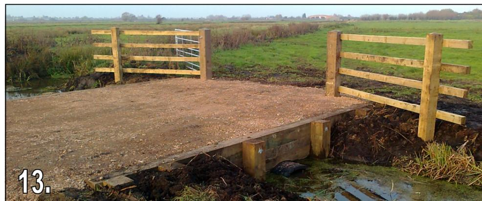
13. Completed headwalls and culvert with gate and back fencing each side.
