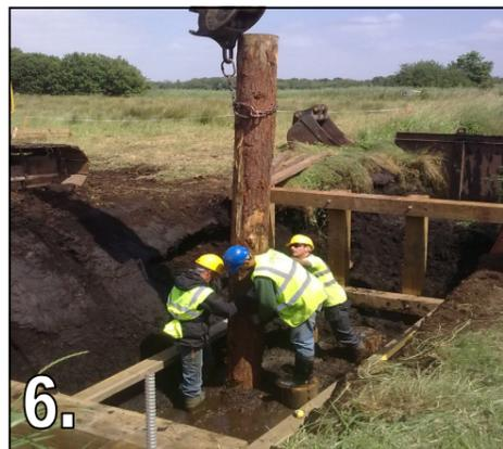
6. Driving large timber piles for pipe support.
