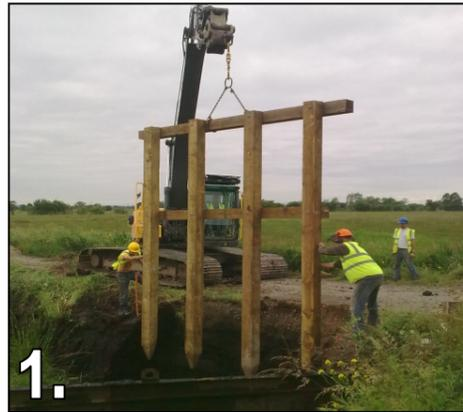
1. Preparing to install pre-assembled structural timber for a headwall (2 required).
