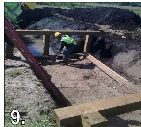
9. Graded stone placed and compacted for the foundation.
