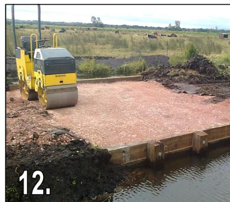
12. Geotextile folded back over pipe bedding, before scalplings laid to finished level and compacted.
