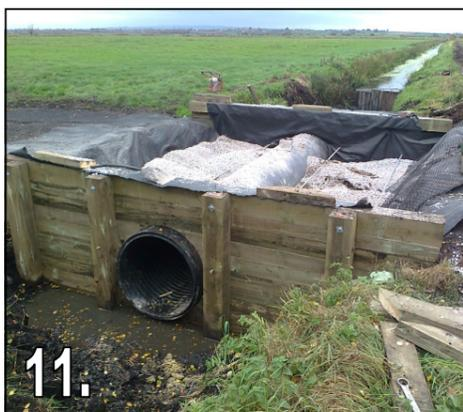
11. Pipe bedding placed and compacted in layers around pipe. Top tie-bars installed and tightened.
