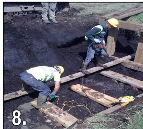
8. Fixing cross timbers for pipe supports.
