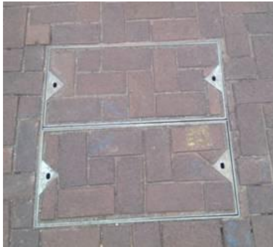
Footway cover - Cover Material: Concrete
