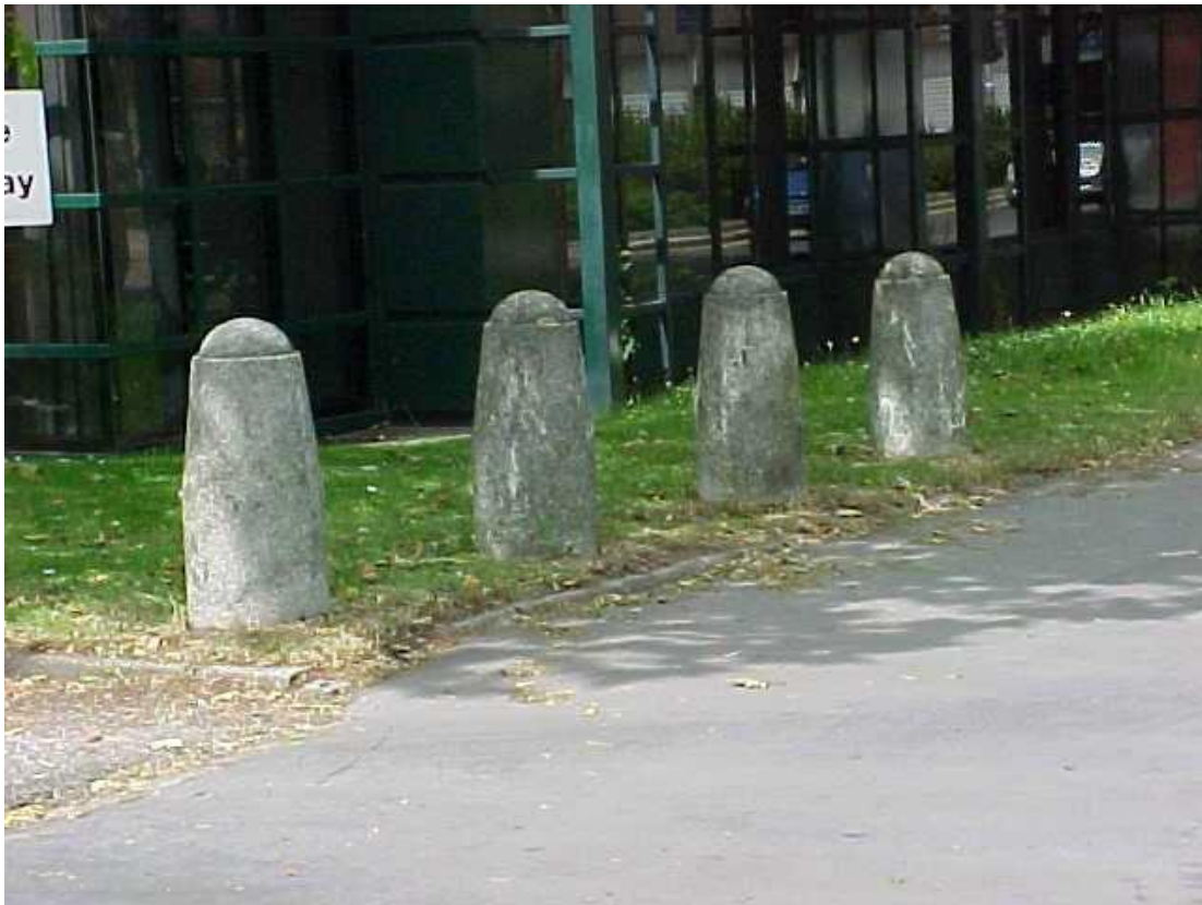
Type: Bollard – Column Material: Concrete
