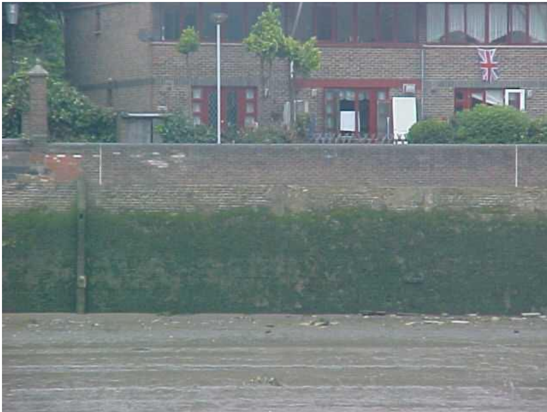
Type: Sheet Piling
