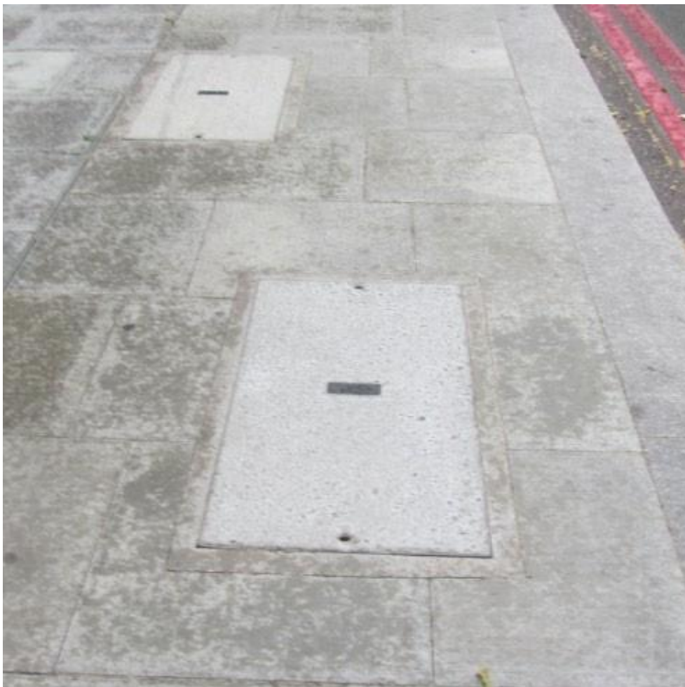
Footway cover - Cover Material: Concrete
