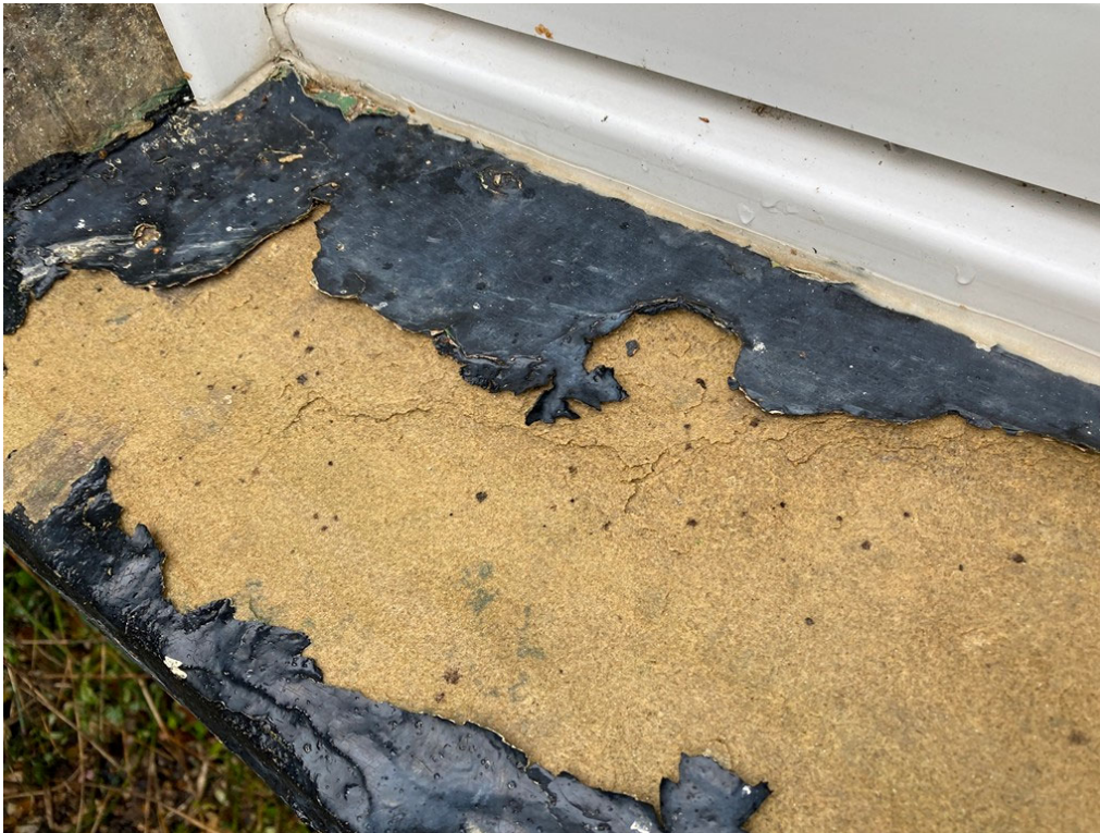
Example of stone sill
