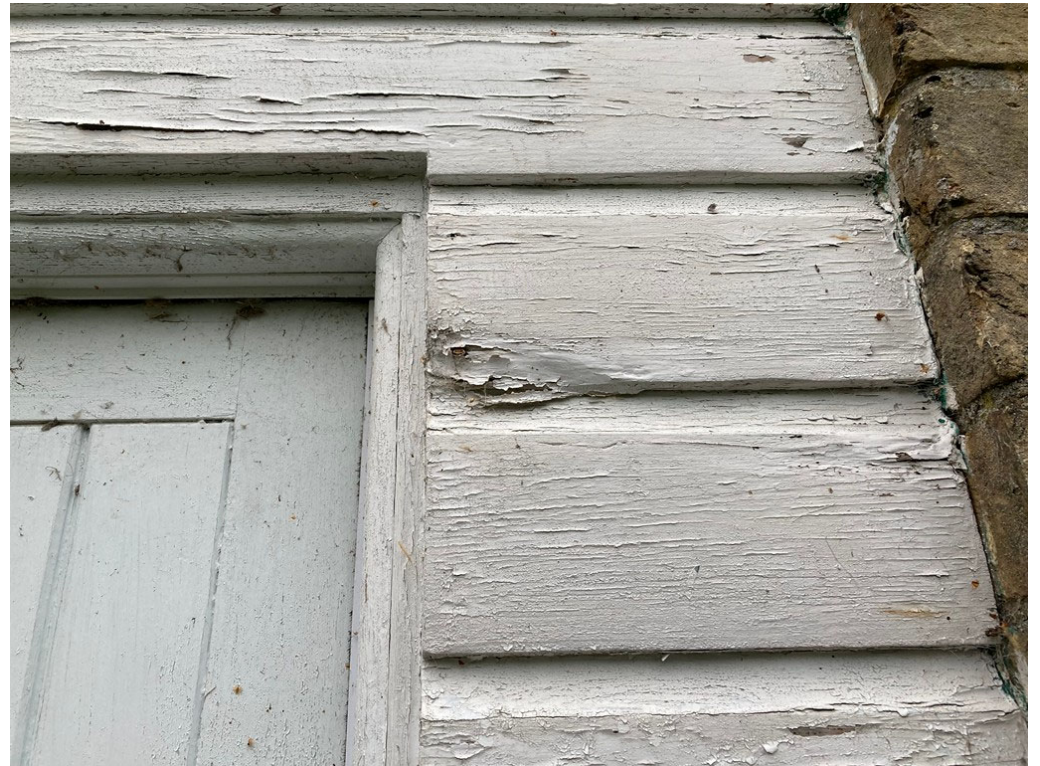
Double timber doors and cladding surround (2)
