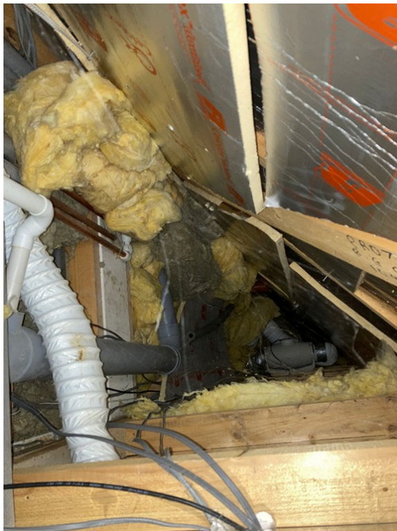
Insulation in eaves space (2)
