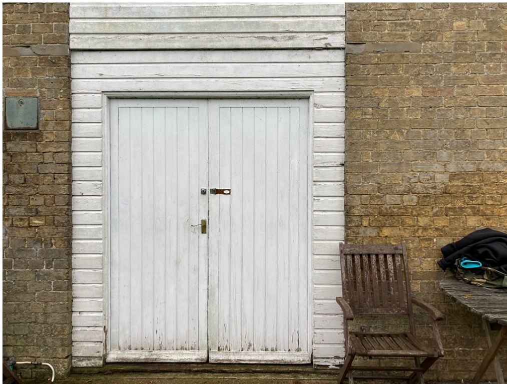
Double timber doors and cladding surround
