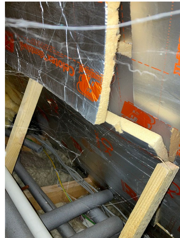
Insulation in eaves space (3)
