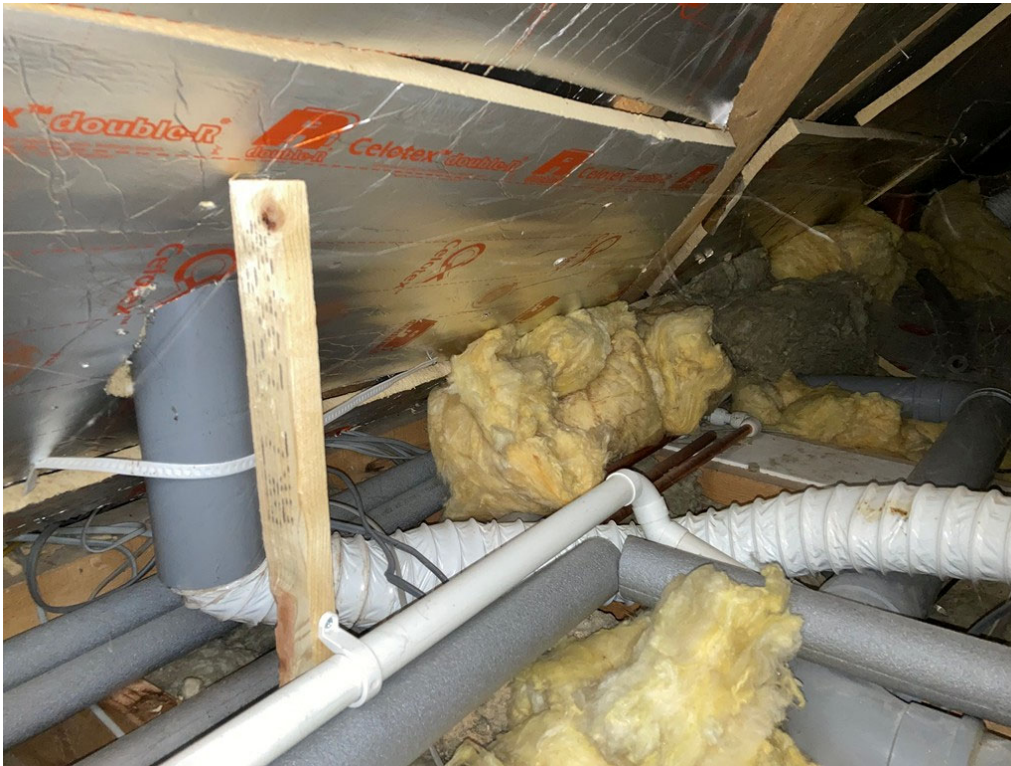
Insulation in eaves space
