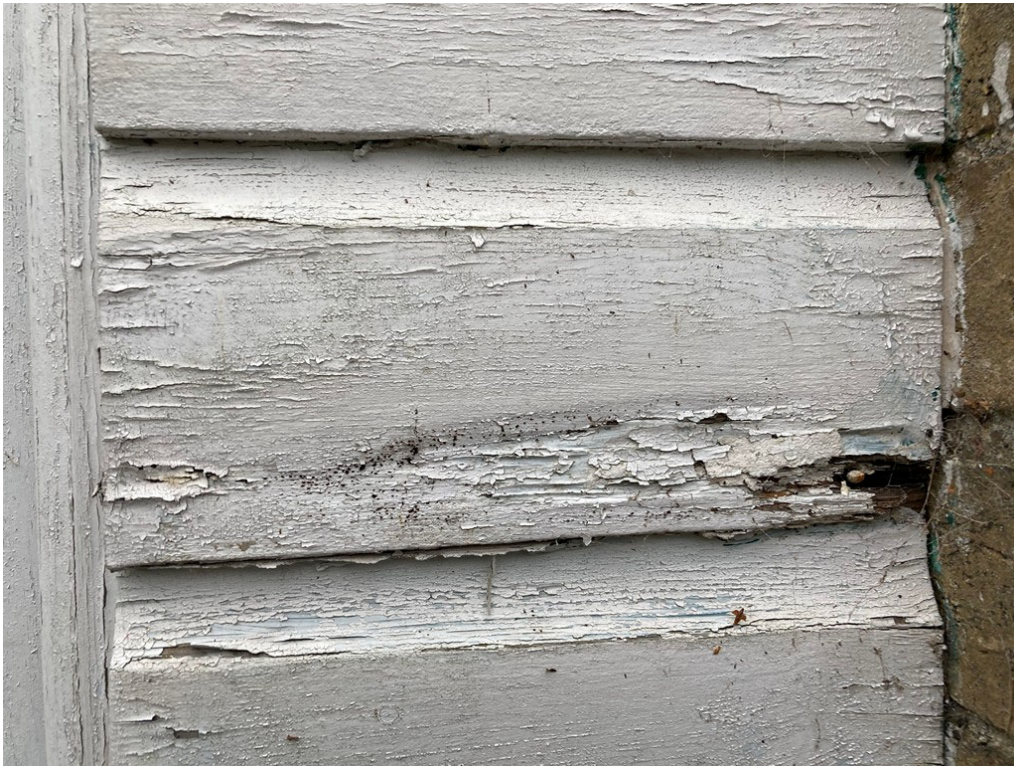
Double timber doors and cladding surround (1)
