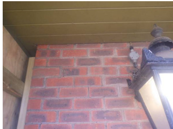
22. Wall 4 High level stepped fracturing adjacent to corner
