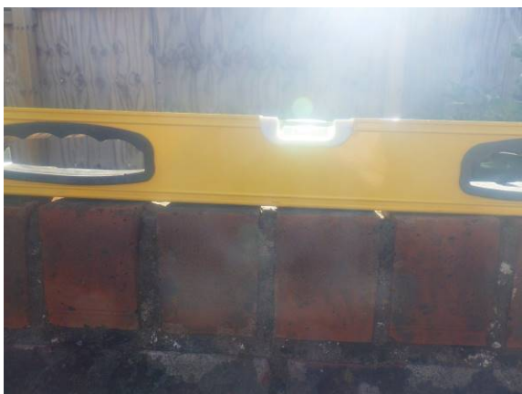
41. Wall C Top of wall falls at 1 in 80
