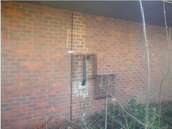
2. Wall 1 brickwork repairs adjacent to joint
