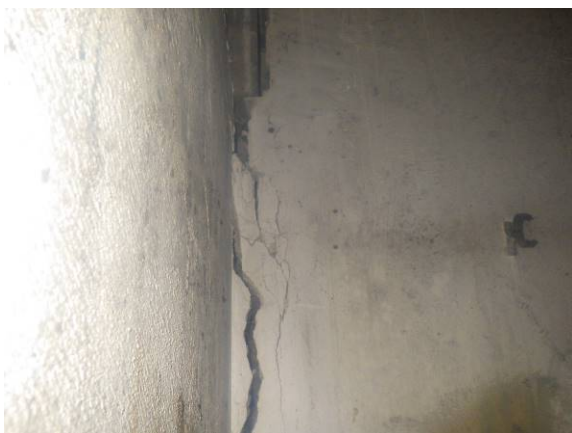
11. Continuation of fracture in 10. Above.
