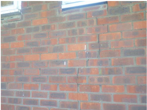
29. Wall 12 Vertical slightly tapering fracture
