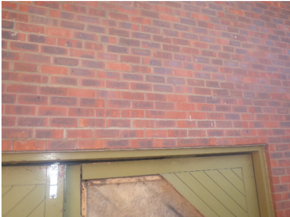
27. Wall 8 Panel over lintel has been repointed
