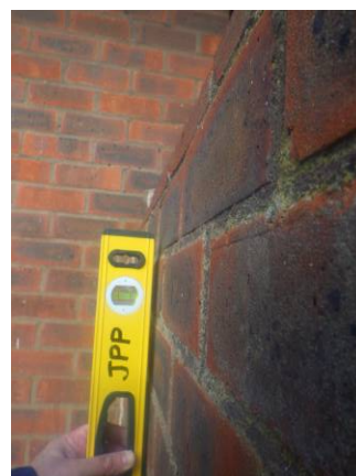
36. Wall A 6mm out of vertical
