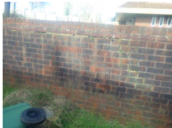
40. Wall C Tapering stepped fracture
