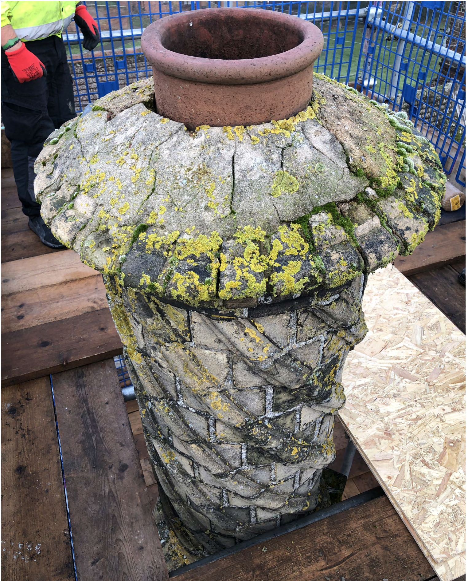
PHOTO 18 - EAST COUNCIL CHAMBER CHIMNEY CAP AND FLAUNCHING PRIOR TO DISMANTLING
