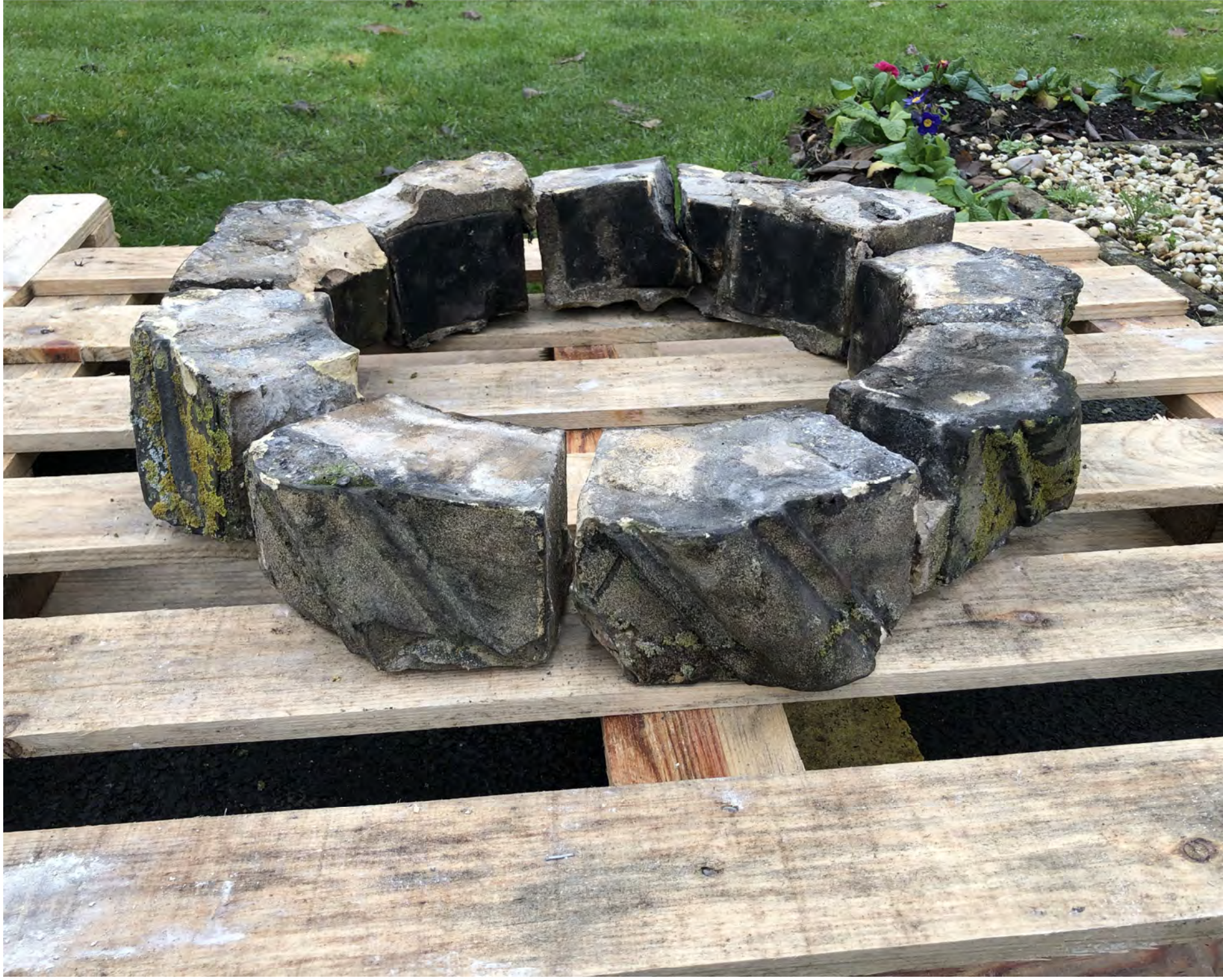
PHOTO 22 - STACK BRICK COURSES FROM EAST CHIMNEY FOR STORAGE AND REUSE
