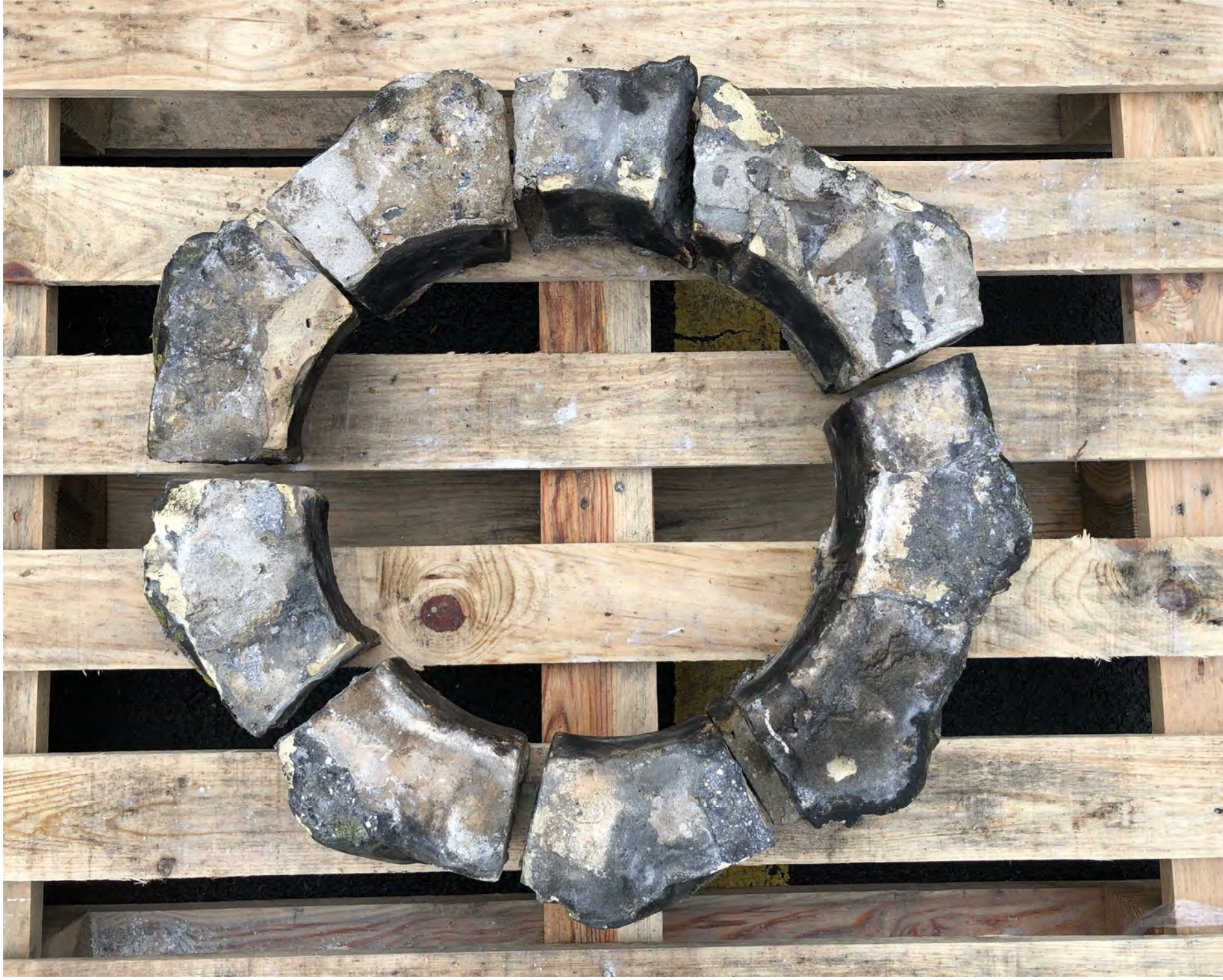
PHOTO 21 - RECLAIMED BRICKS FROM EAST CHIMNEY FLUE STACKED FOR STORAGE AND REUSE AFTER DISMANTLING
