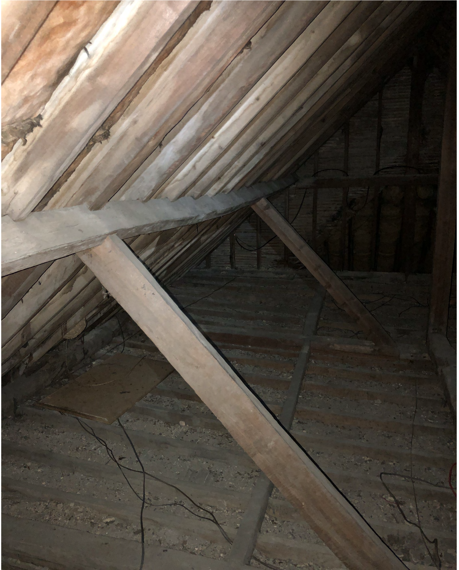
PHOTO 24 - TYPICAL RAFTER, PURLIN AND PROP TO TRUSS ARRANGMENT OVER COUNCIL CHAMBER
