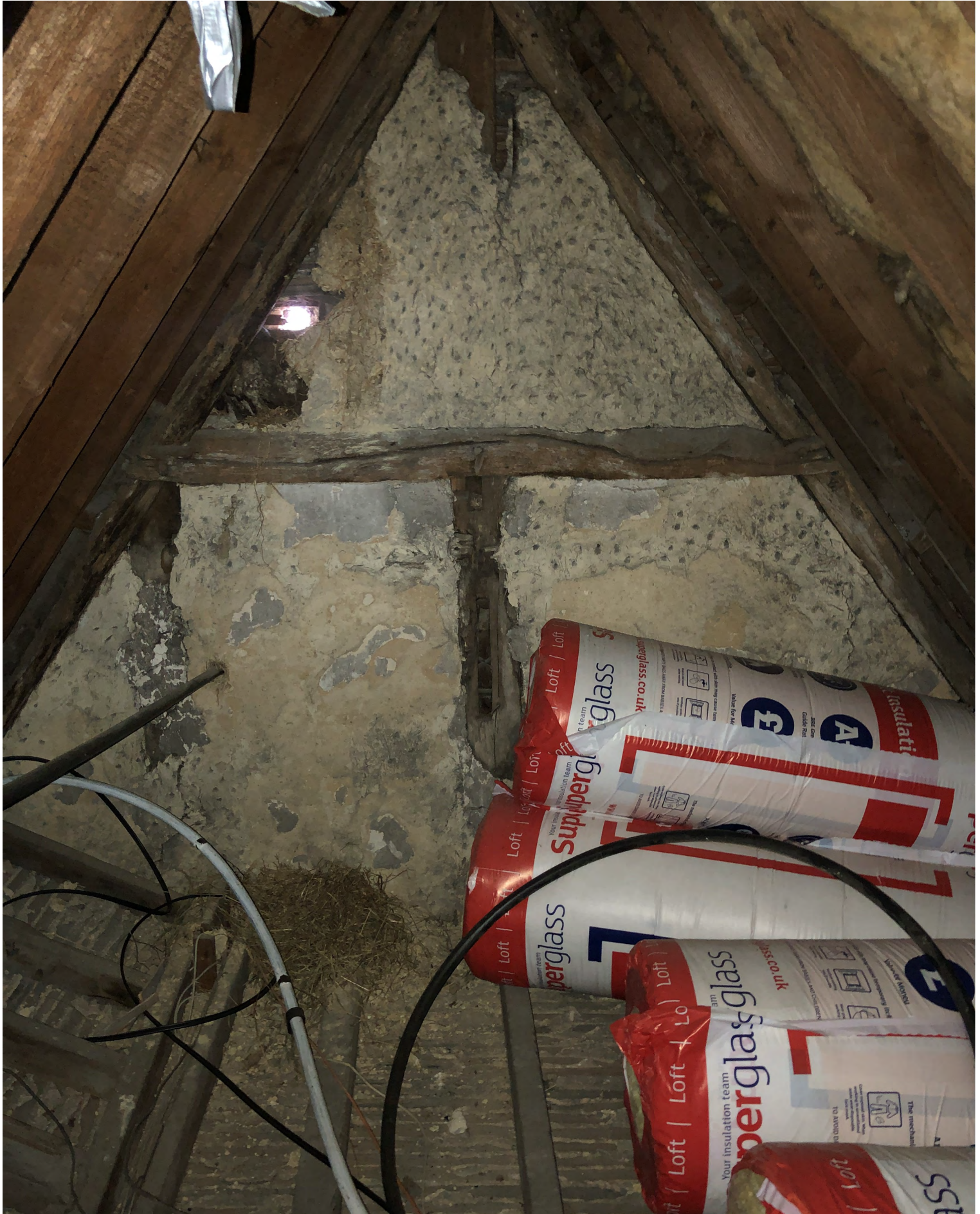
PHOTO 26 - TIMBER FRAME AND WATTLE & DAUB / COB INFILL TO WEST GABLE ELEVATION OVER REGISTRAR'S OFFICE TO BE REPAIRED
