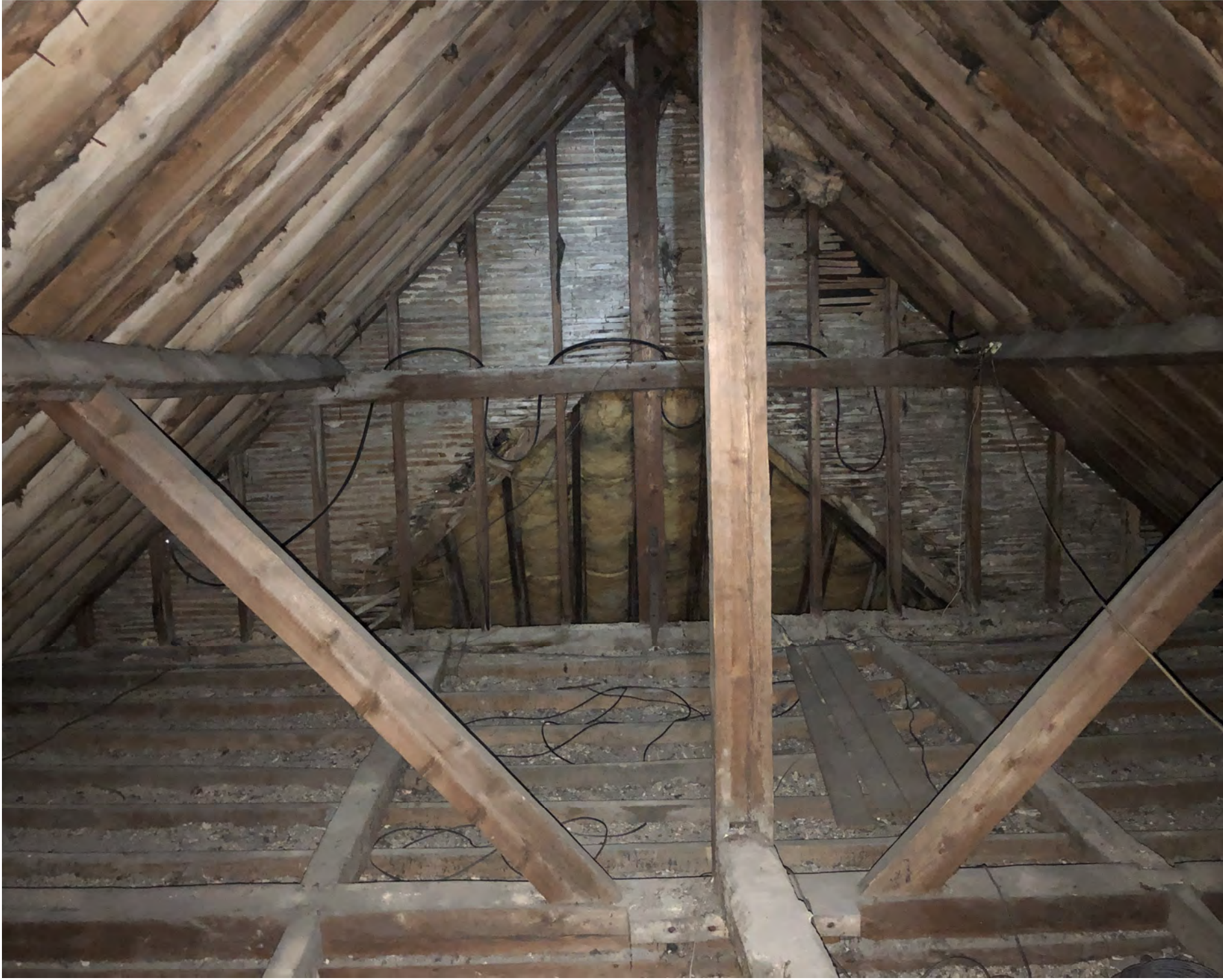
PHOTO 23 - TYPICAL ROOF TRUSS AND STRUCTURE OVER COUNCIL CHAMBER
