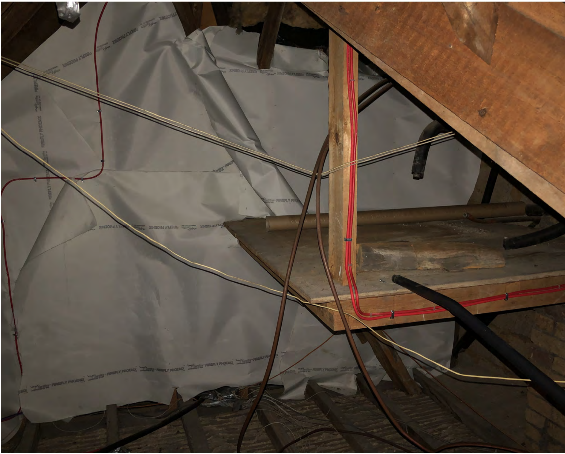
PHOTO 27 - MISC CABLES TO BE RE-ROUTED AND AND REDUNDANT TIMBER PLATFORM OVER REGISTRAR'S OFFICE TO BE REMOVED
