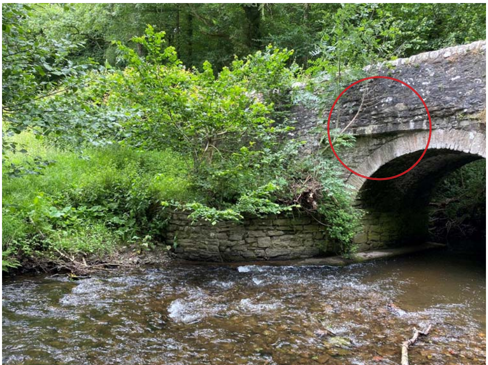
Photograph 2 - Bulge in upstream parapet
