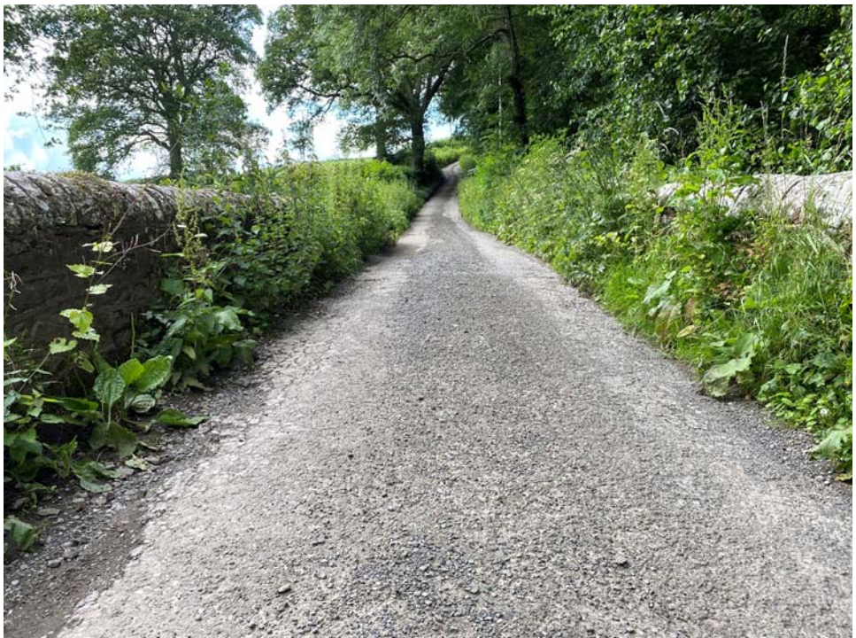
Photograph 1 - Small hump within carriageway and loss of surface dressing
