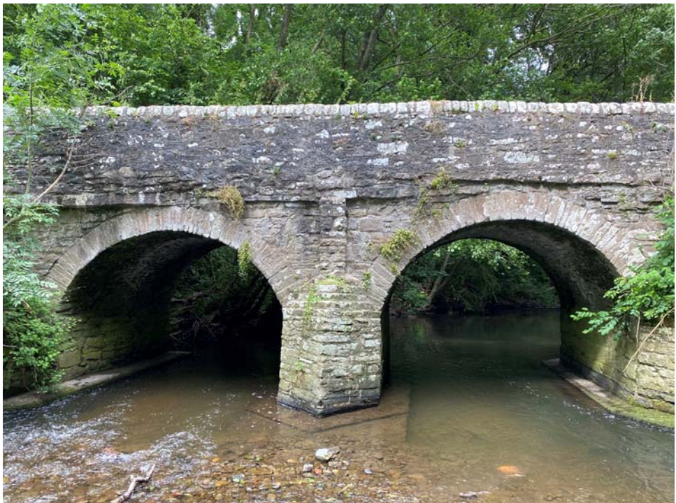
Photograph 3 - Noticeable lean on the pier (90mm)
