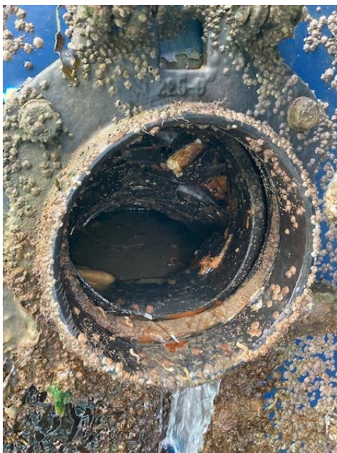
Typical poor condition flap
