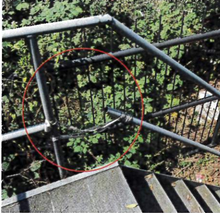
Fig 7. Broken hand rail to be repaired.
