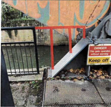
Fig 5. Indicative set up of small infill fence left bank.
