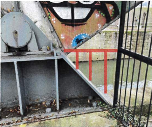
Fig 4. Indicative set up of small infill fence island side.
