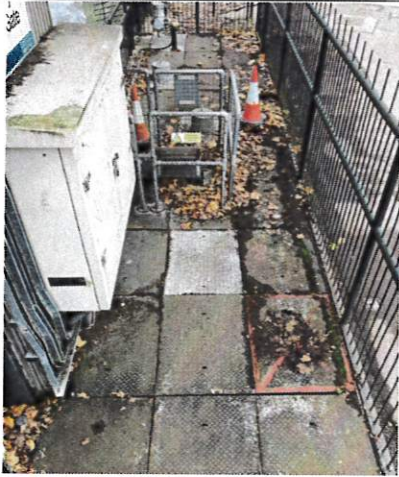
Fig 1. Metal cover plates to be replaced, left bank of sluice channel shown.
