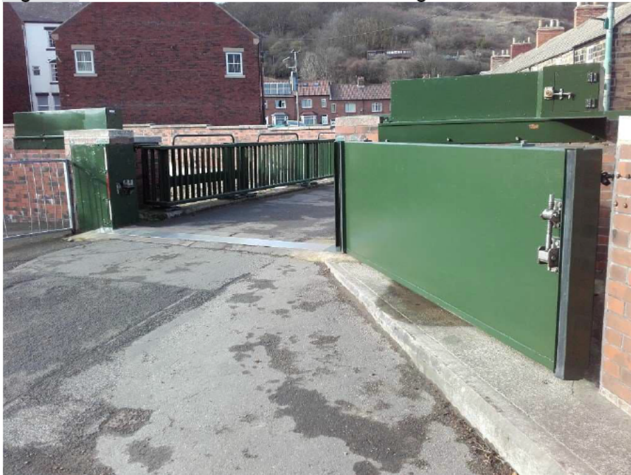
Figure 2 Stone Row Bridge flood gates and demountable parapets
