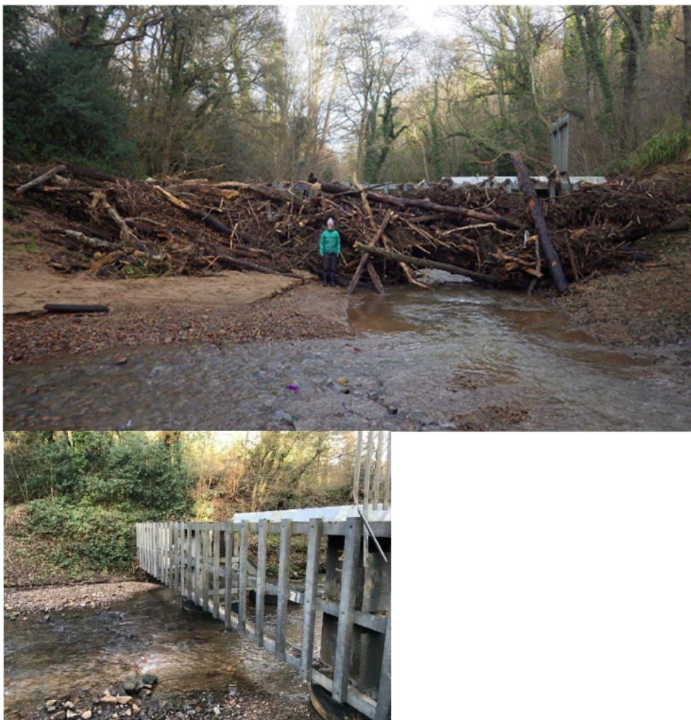
Figure 3 Log catcher clear (left) and fully loaded (right) after high flows.
