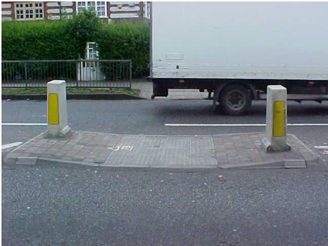
Surface: Pedestrian Deterrent (can be in pyramid as well as block form)
