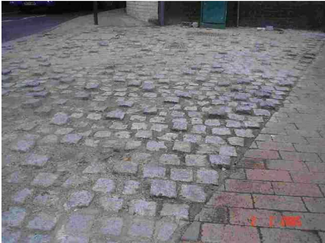
Surface: Pedestrian Deterrent (can be in pyramid as well as block form)
