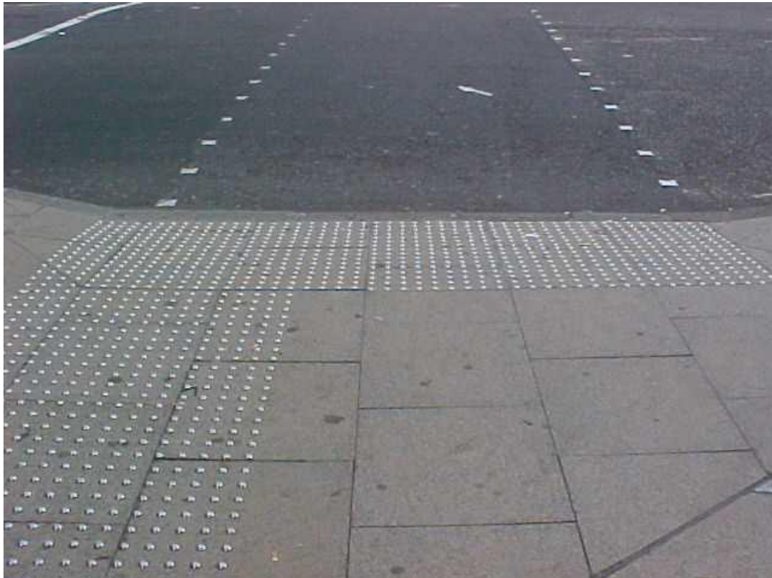
Type: With Tactile – Tactile: Studs
