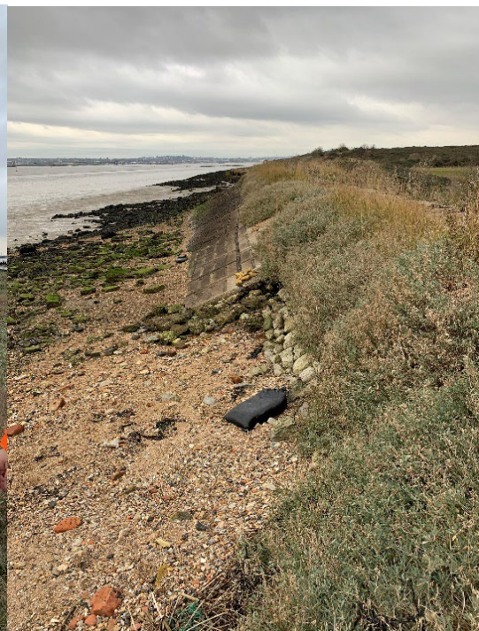
Front face vegetation and seepage area
