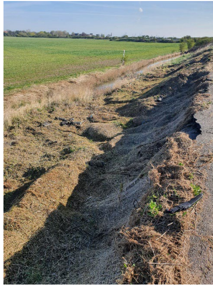
Front face vegetation and seepage area
