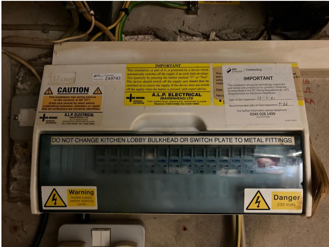
72. Electric Distribution Board
