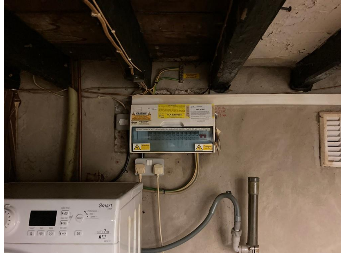
71. Electric Distribution Board
