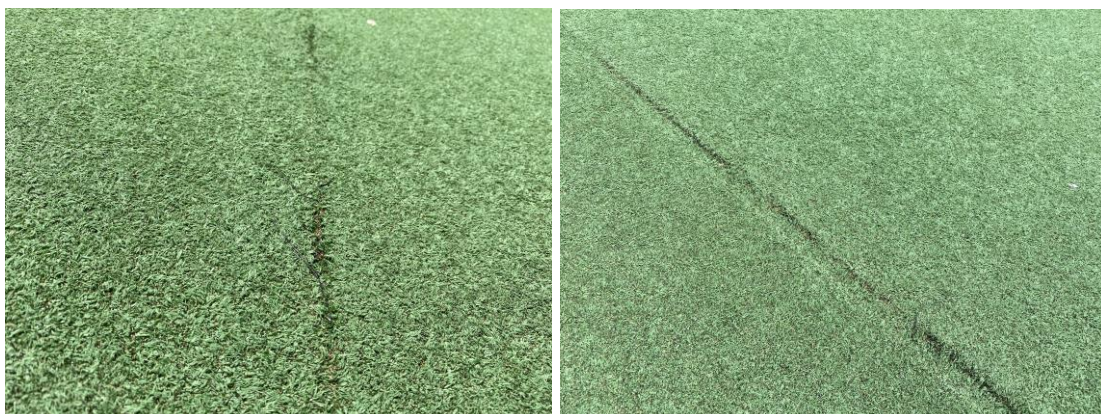
SEAM FAILURES
