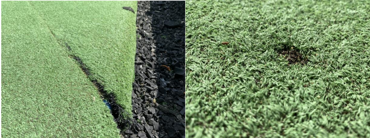
SEAM FAILURES
