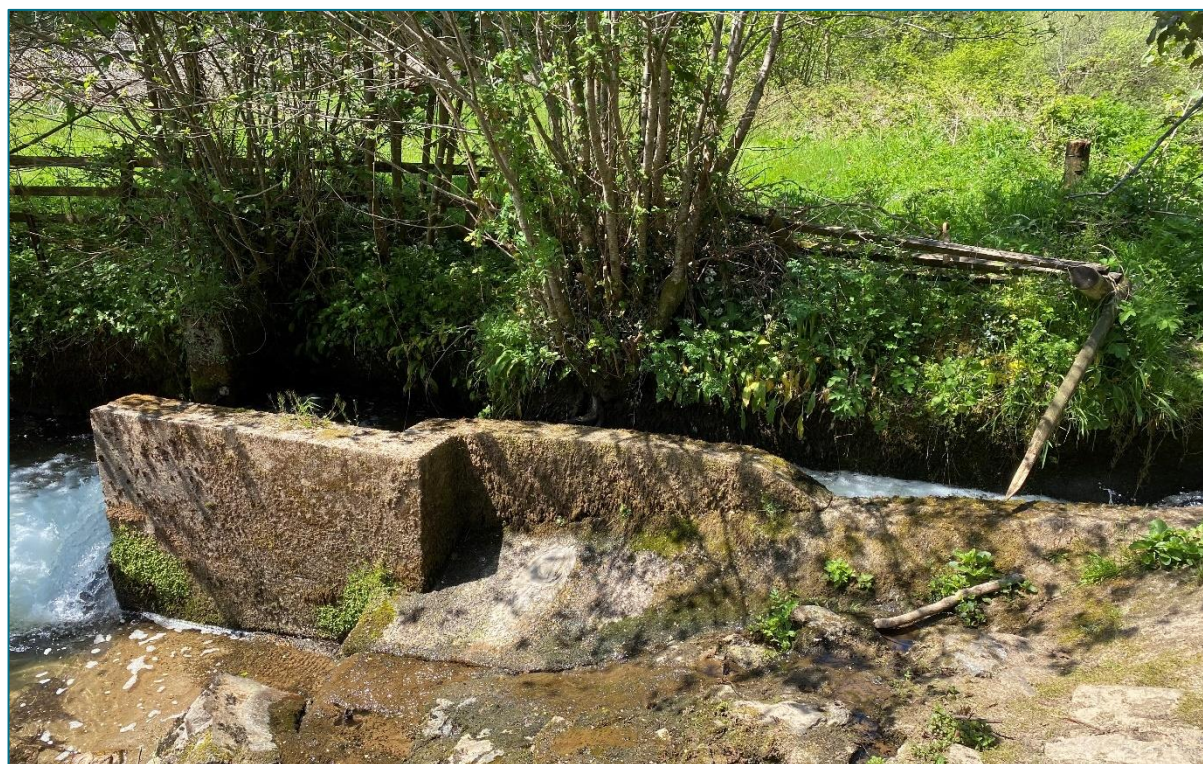
Photo 20: Close up of the existing fish pass channel to house the new fish pass (looking west).
