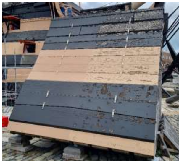
Ship Side Mock Up, June 2022. Note the difference of degradation of right side of mock up.
