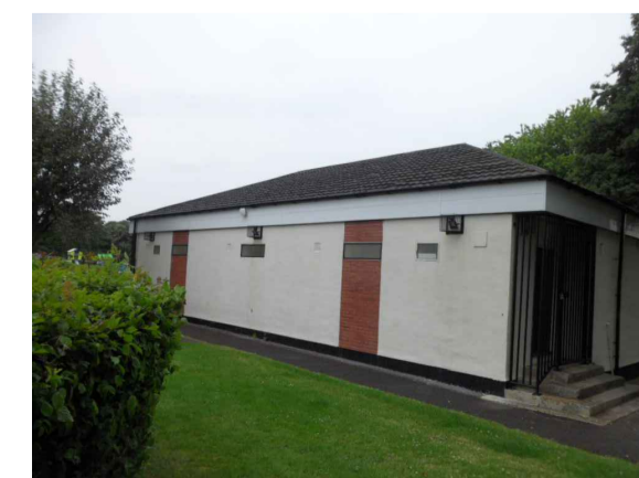
The Pavilion Reburishment
