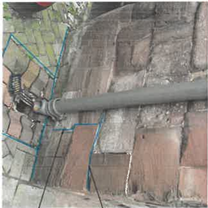
Rake out and deepack and repoint thin horizontal mortar joint under base of corner stone
