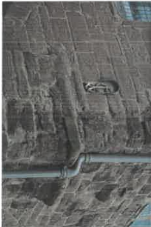
Minor areas of repointing required to the upper corner stone joints which may have been washed out from the overflowing guttering above. Gently clean the existing stone to remove staining and algae
