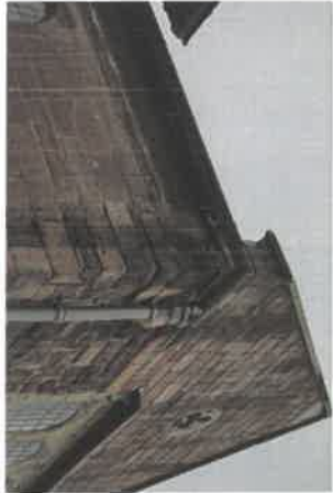
Minor areas of repointing required to the upper corner stone joints which may have been washed out from the overflowing guttering above. Gently clean the existing stone to remove staining and algae
