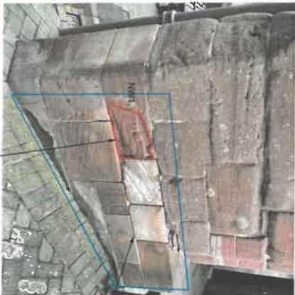
Carefully rake out and deep repoint the thin joints between existing stone blocks within the blue outline.
