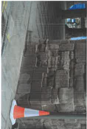
South east corner shown above demonstrating its close proximity to the adjacent highway. A likely contributory factor to the lower stone and mortar erosion.
