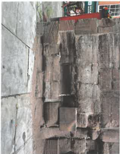
Area of stone corresponding to drawing Current condition of existing lower left wall to the south west corner.
