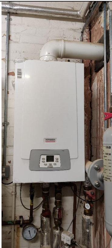
Photograph 3 - Wall-mounted Potterton condensing boiler – IN FAULT (flue through wall outside curtilage)
