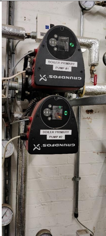
Photograph 5 - Grundfos boiler primary pump (connecting boilers to PHX, radiators and radiant panels)
