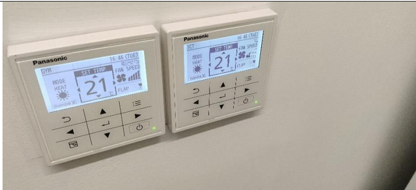
Photograph 22 - Retrofitted Panasonic room controllers
