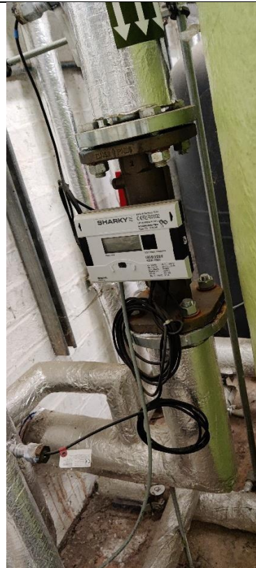
Photograph 10 - ASHP circuit heat-meter (not evident on BMS)
