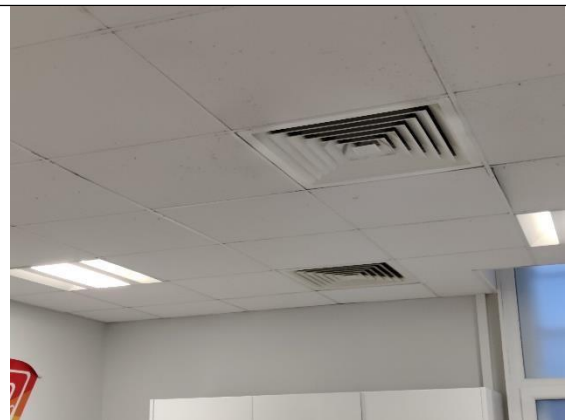
Photograph 25 - Typical classroom MVHR diffusers
