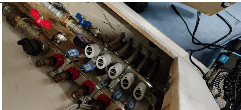
Photograph 16 - underfloor heating manifold in hall chair store cupboard
