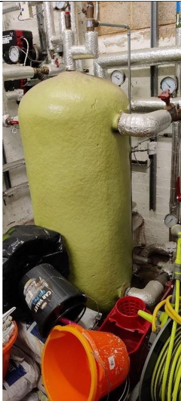
Photograph 9 - ASHP circuit buffer vessel in plant room (note materials stored in the plant room)
