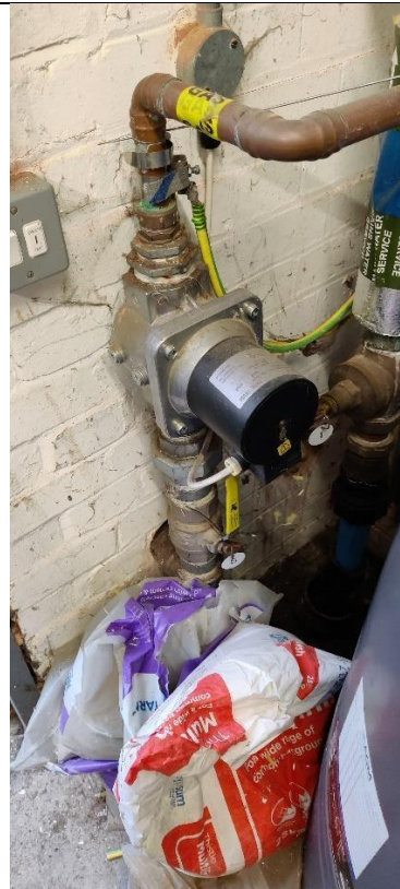
Photograph 2 - Gas supply & solenoid entering plant room
