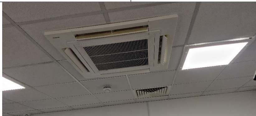
Photograph 21 - Retrofitted Panasonic classroom cassette unit
