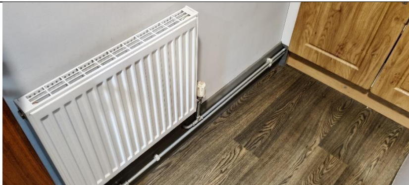
Photograph 12 - typical steel panel radiator in office (with TRV) - fed by boiler circuit
