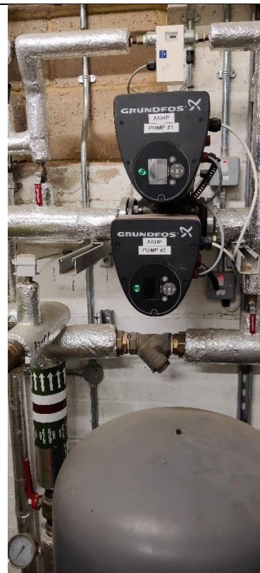
Photograph 8 - Grundfos ASHP circuit pump, connecting ASHP, buffer vessel, underfloor heating and MVHR's
