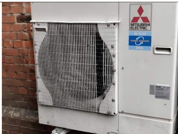
Photograph 18 - Original installation Mitsubishi outdoor unit
