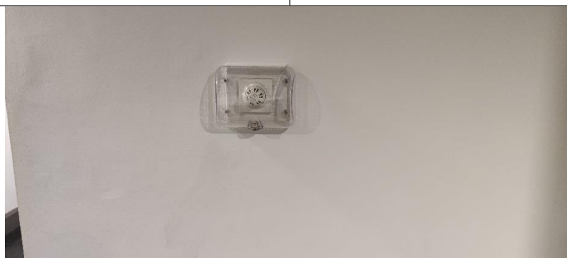
Photograph 15 - Radiant panel remote TRV head in protective Perspex box
