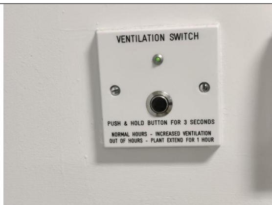
Photograph 24 - local ventilation extend/override control (stock in on position)
