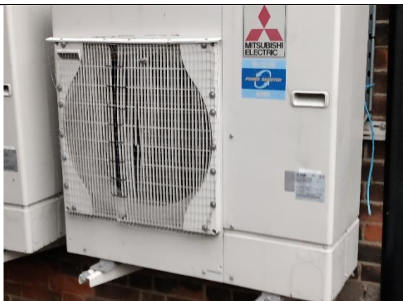
Photograph 17 - Original installation Mitsubishi server room outdoor unit
