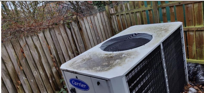
Photograph 11 - Carrier air source heat-pump in external enclosure (note standing water on unit and rubbish in enclosure)
