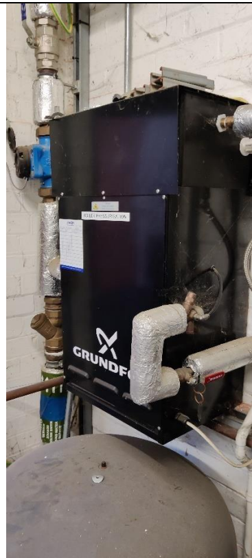
Photograph 4 - Gas heating pressurisation unit and expansion vessel
