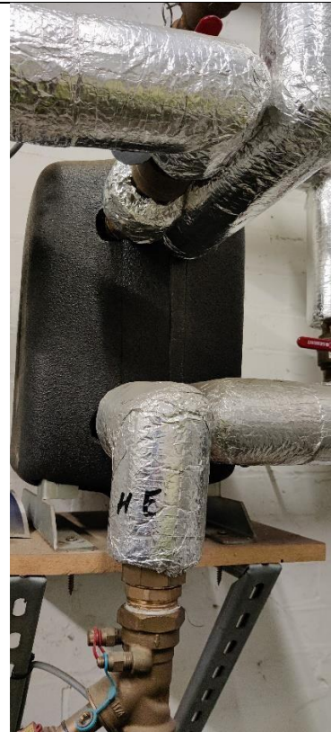
Photograph 6 - Plate heat exchanger between gas boiler and ASHP circuits
