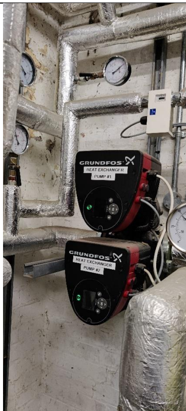
Photograph 7 - Grundfos PHX pump (connecting PHX to buffer vessel)
