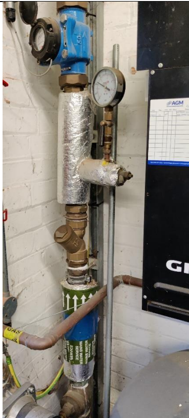
Photograph 1 incoming water main and meter in plant room
