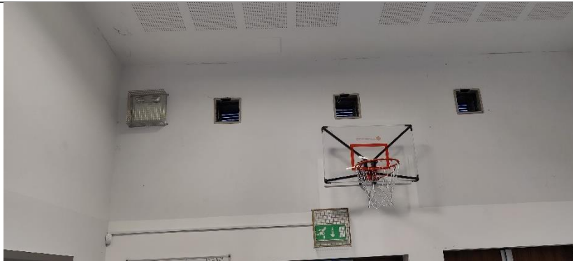
Photograph 23 - Missing hall high level extract fans (removed)
