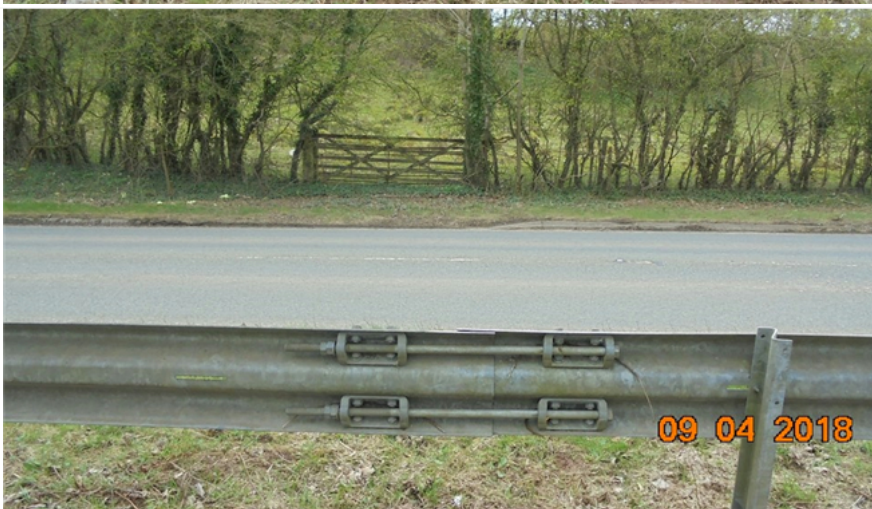
Lower Tension Assembly
