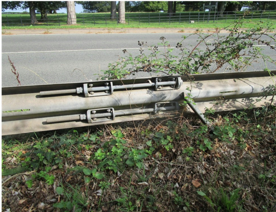
Damaged post next to Tension Assembly
