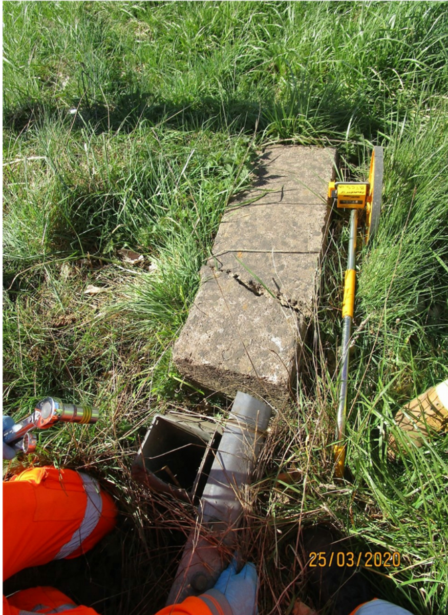
Departure assembly and damaged concrete anchor
