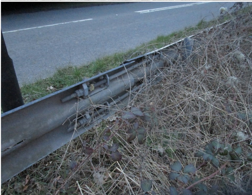
Middle tension assembly.
