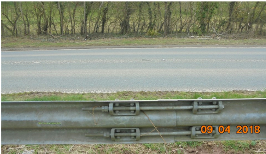
Middle Tension Assembly
