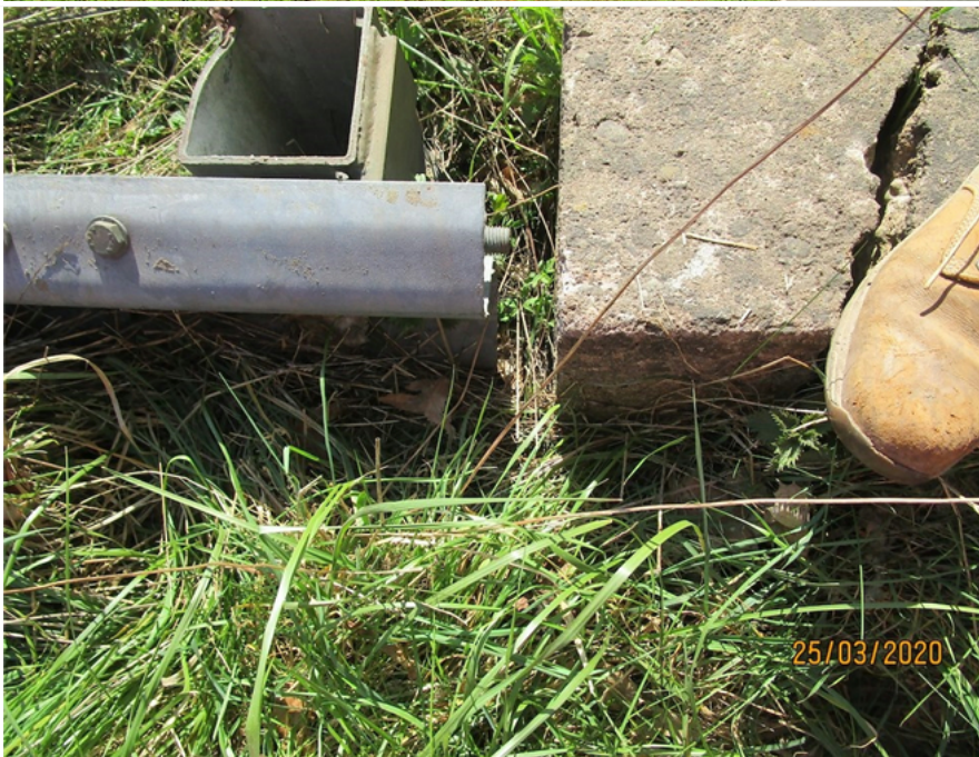
Departure assembly and damaged concrete anchor
