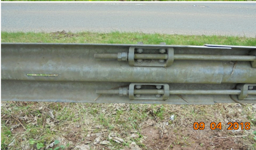
Middle Tension Assembly
