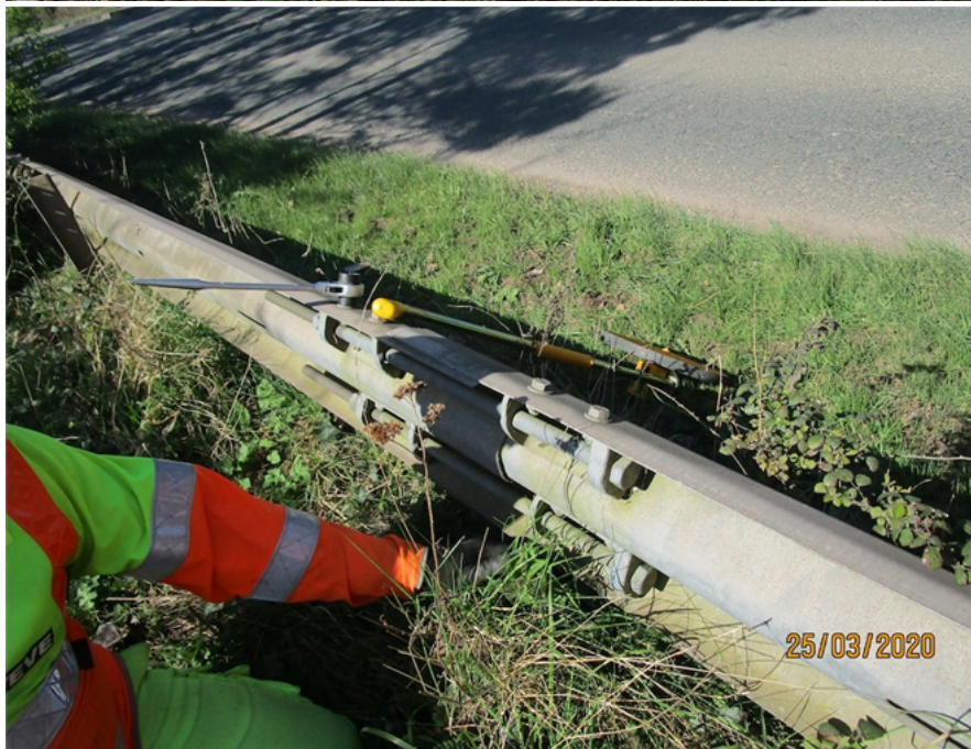
1st Tension Assembly
