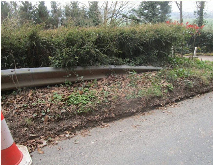
End terminal anchorage.
