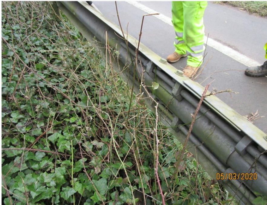
Middle tension assembly.
