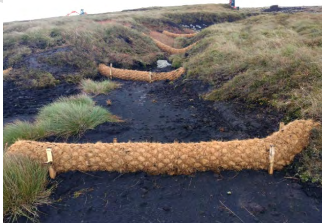
Figure 8 Top: Established heather bale dam (Photo credit: Moors for the Future). Bottom: Coir rolls on Pendle Hill, Lancashire. Photo credit: Conservfor Ltd
