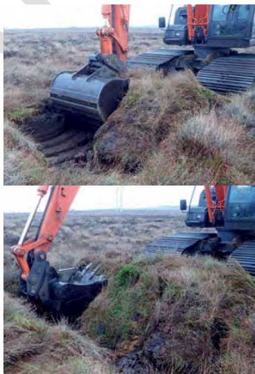
Figure 4 Creation of a wave dam (Short & Robson, 2016)
