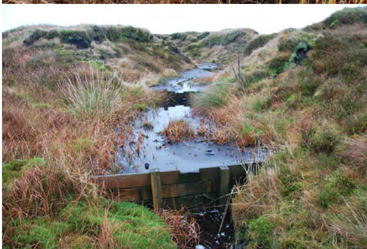
Figure 6 Top: Plastic piling in a raised bog (Thom, 2019); Bottom: Timber dams in a blanket bog gully. Photo credit: Moors for the Future
