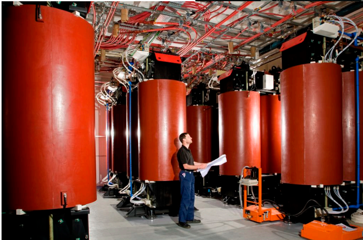
Figure A3: ISIS New Choke Room with Chokes in Situ
