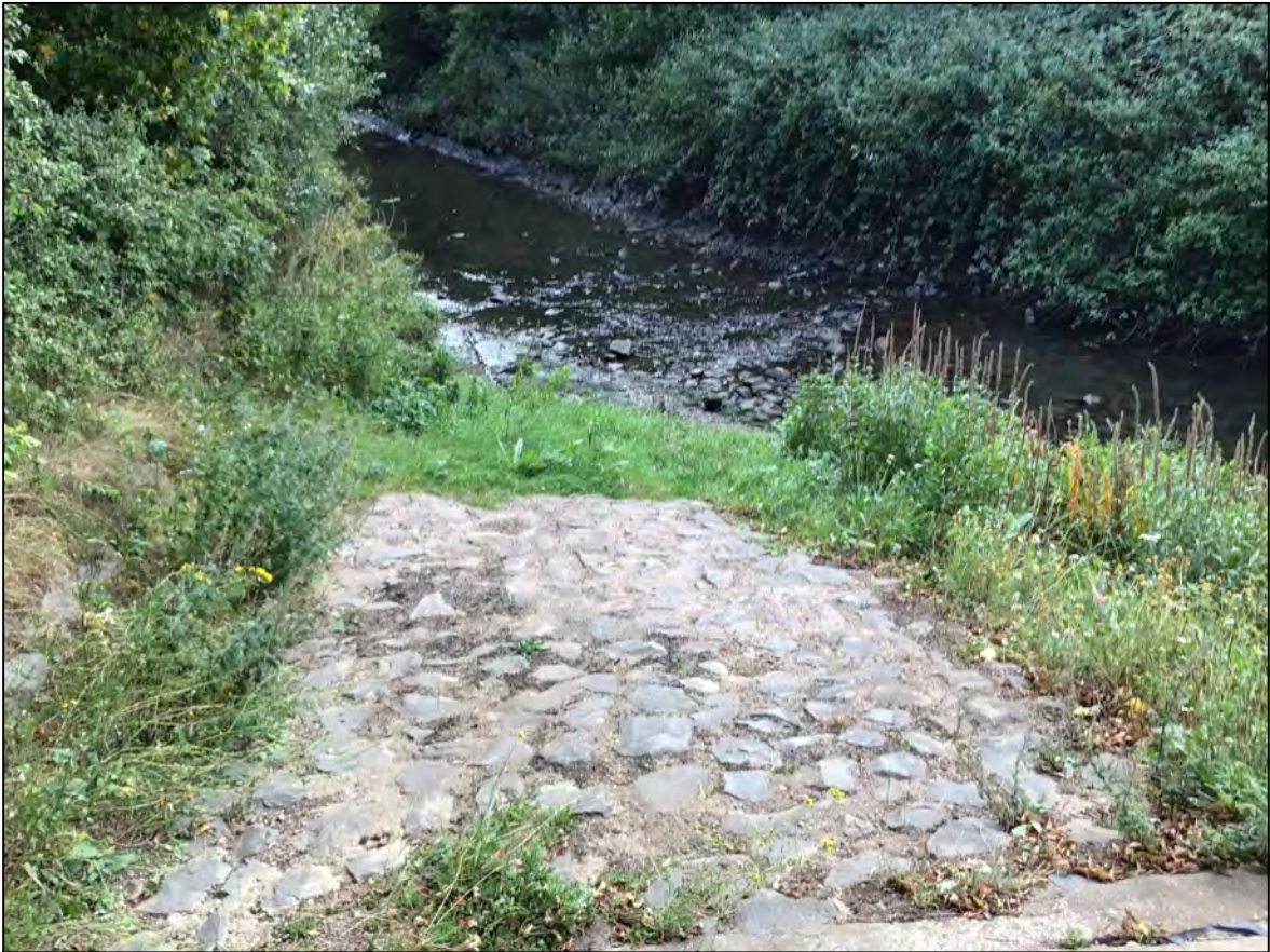
IMAGE 1 - EXISTING ROCK ARMOUR TO RAMP
