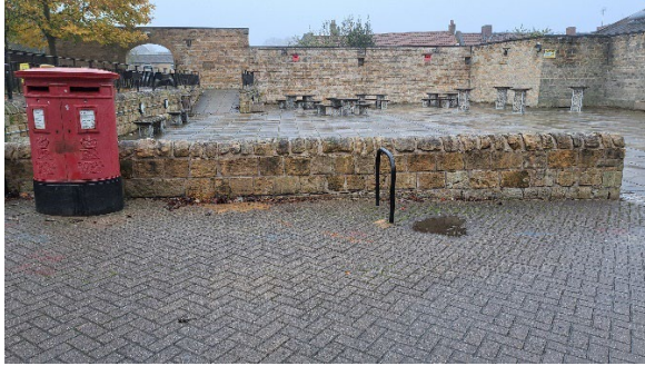
Figure 6 South elevation of stone wall to Cotton Street
