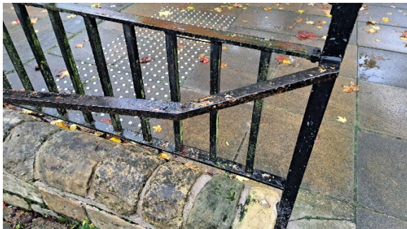
Figure 1 Upper end of existing handrail to be removed
