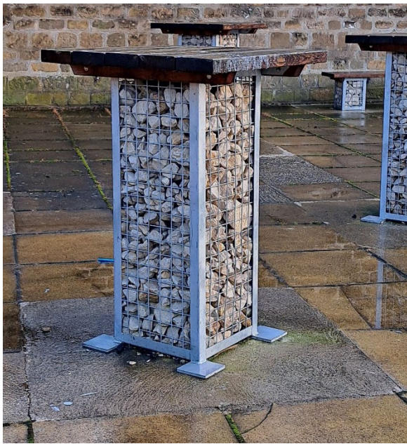
Figure 15 Typical bar table currently on site
