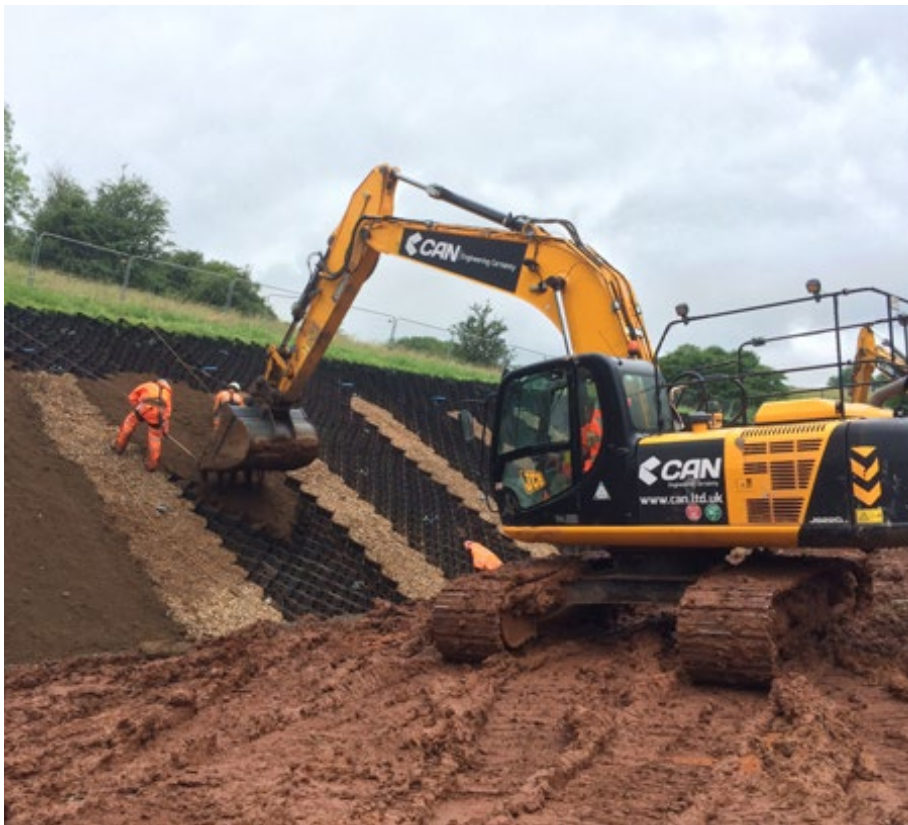
DYWI® Drill Hollow Bar & TECCO® overlaid with Geocell to retain topsoil on the face
