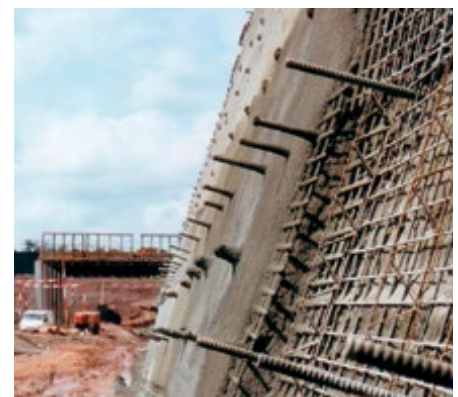
DYWI® Drill Hollow Bar shotcrete used to create a rigid face to a stabilised slope.
