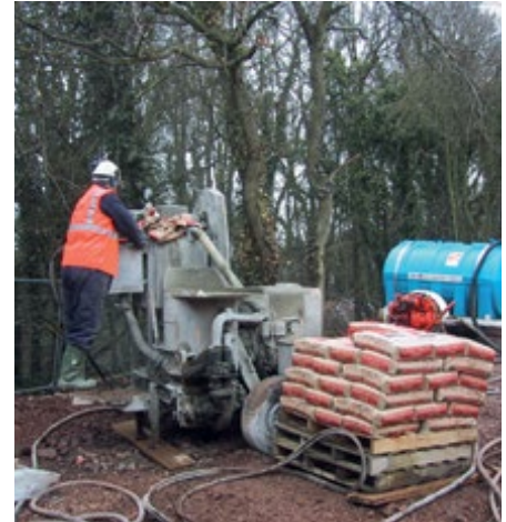
Typical grout plant set-up
