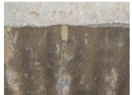
T76 Micro Piles forming a contiguous wall
