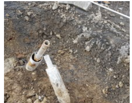
Raking T76 Micro Piles
