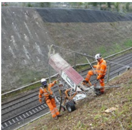
A Frame drilling at Watford Cutting
