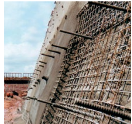
Grouted soil nails on shotcrete face
