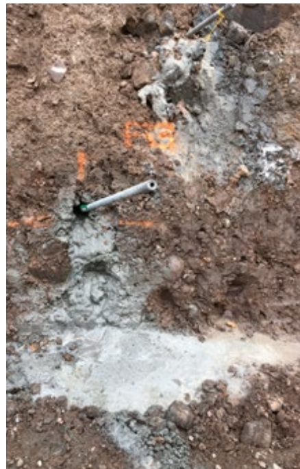
DYWI® Drill Hollow Bar installed with simultaneous drill & grout HoTV A465 South Wales
