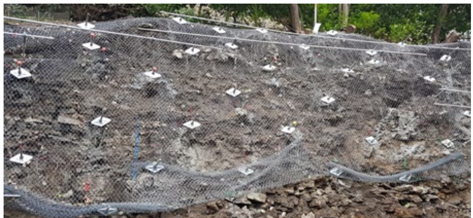
DYWI® Drill Hollow Bar & TECCO® G45/2 stabilising a new cut in Halifax
