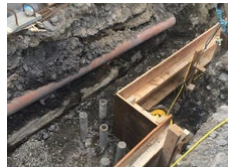
T76 Micro Piles forming a contiguous wall
