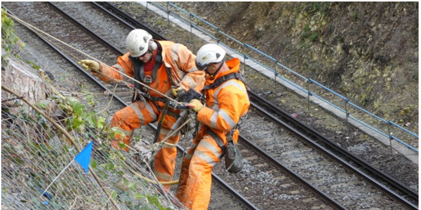
Hand drilling through DELTAX® at Hove
