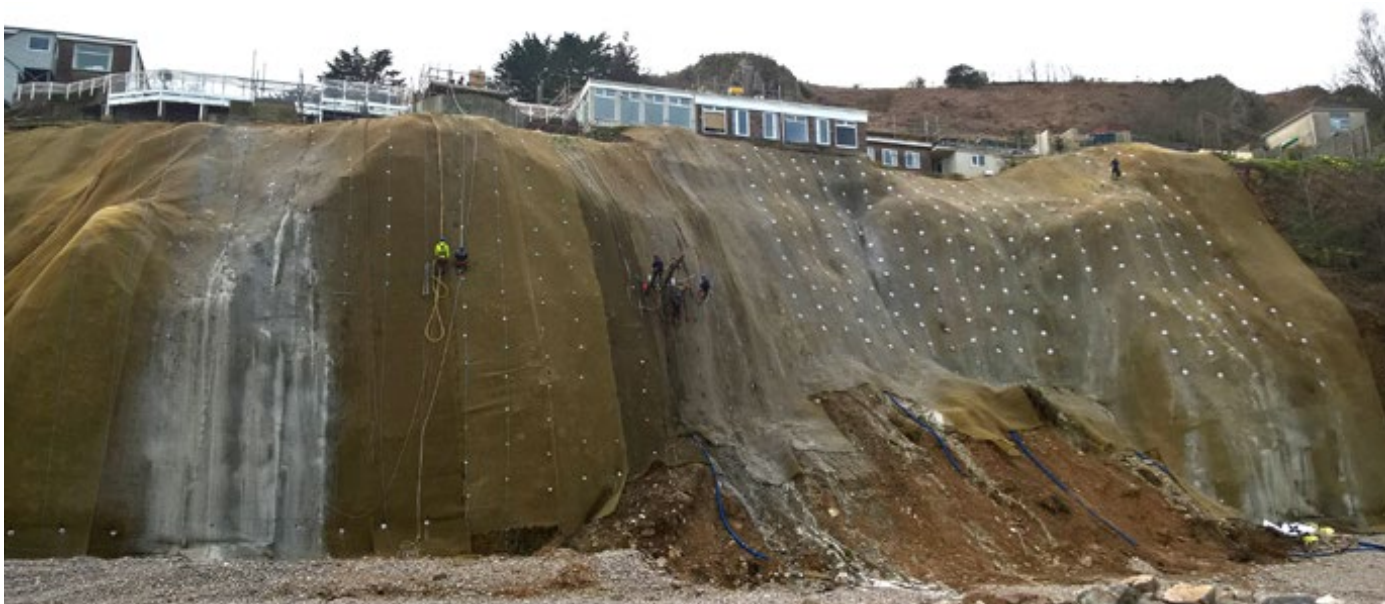
Spoil at toe left in place as erosion control and slope buttressing, DYWI® Mat Green used to prevent erosion.
