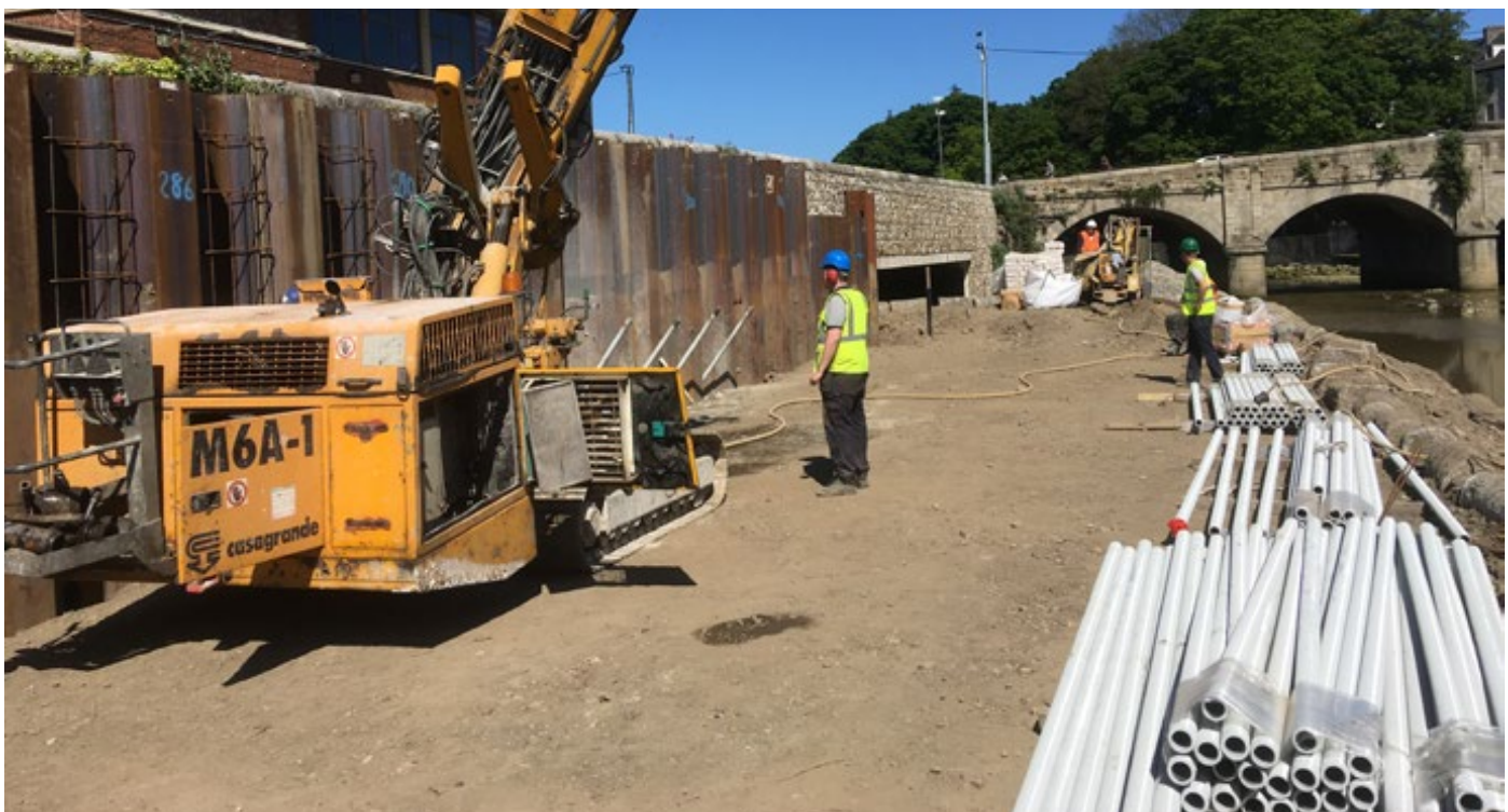
DYWI® Drill R51 Duplex coated Hollow Bar is installed on the River Dargal Flood Aleviation Scheme, Ireland
