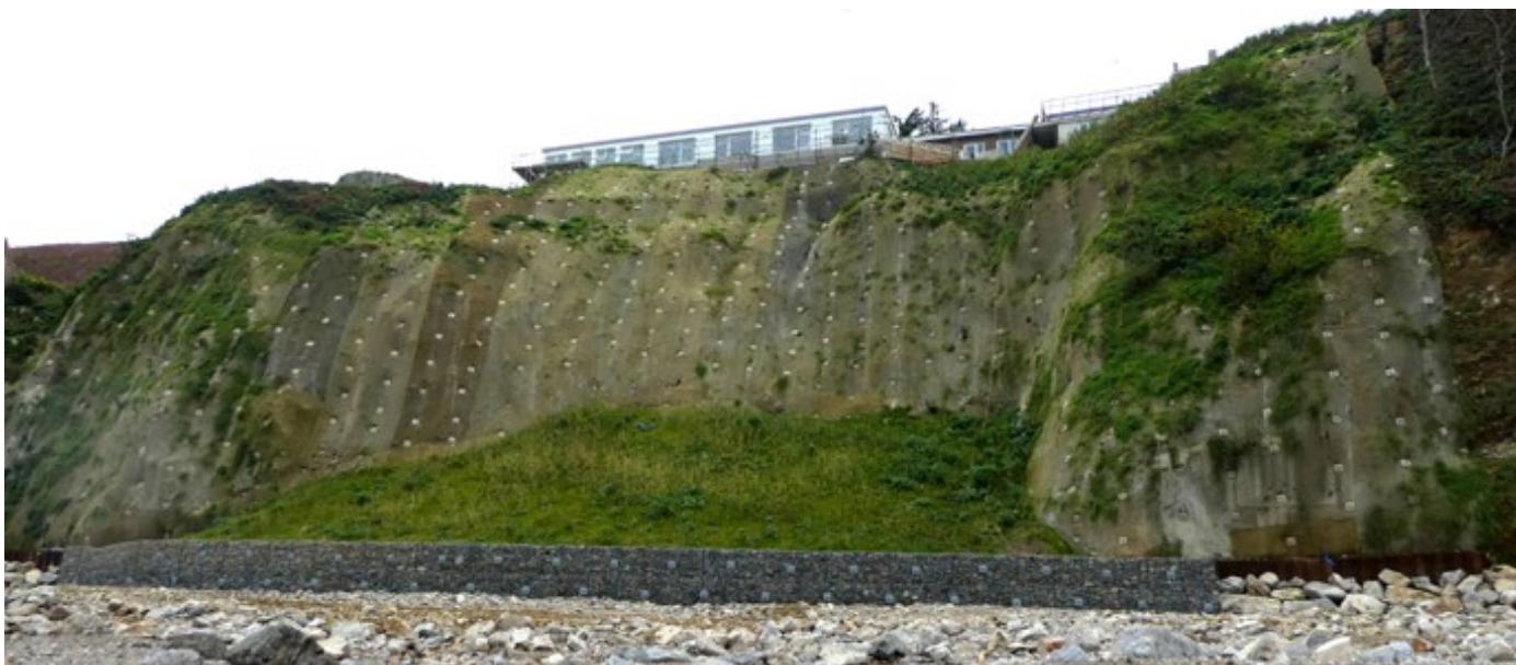
GREENAX® enables vegetation to establish on steep slopes, providing further reinforcement to the cliff face.
