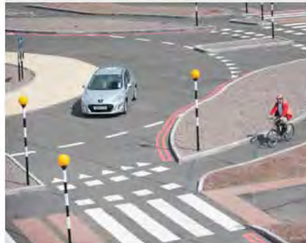
Figure 41: Dutch style roundabout being trialled at TRL
