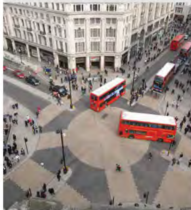
Figure 58: Coloured surfaces reinforce signalised diagonal crossings for pedestrian movements
