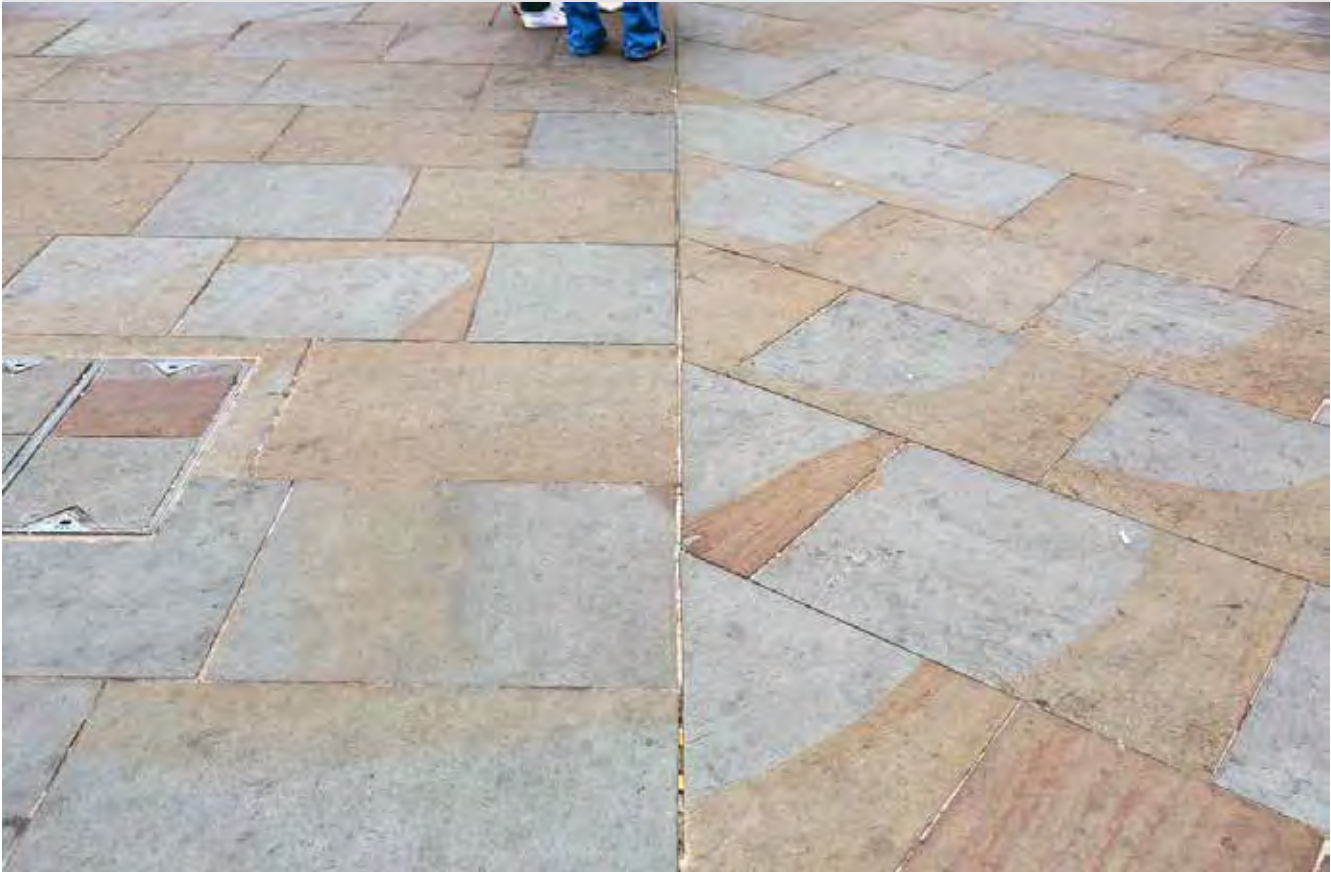
Figure 69: Careful attention should be given to the treatment and appropriate cutting at locations where surface materials of different types or alignments join. The footway on the left side of the cut line shown in this image has taken precedence, as the primary road of the two
