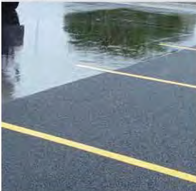
Figure 37: Permeable asphalt allows water to infiltrate
