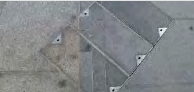
Figure 85: Paving pattern inset into an inspection cover
