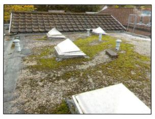
is now in a tired state of repair and we recommend that this is scheduled for renewal short term. At the same time, the various lead flashing details at the junctions can be addressed. Many of these have various splits and have suffered UV degradation over the years. Quite a lot of the lead flashings at junctions are made in lengths greater than would be best practice, resulting in some splits and cracking due to thermal expansion and contraction.
