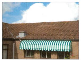
South facing roof slope finished in the delta roof tile. The ridge tiles are bedded in mortar but the joints to the ridge tiles are open in places and lacking pointing.
