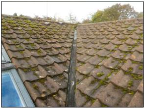
tends to result in a need for reroofing, as the secondary means of weatherproofing is reduced.
