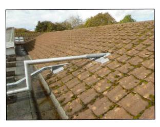
Two conduits enter this roof slope is finished with lead flashings. This arrangement appeared to be satisfactory.
