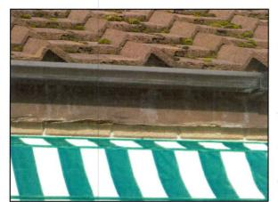
The various UPVC sections are generally all serviceable but showing signs of UV degradation in places.
