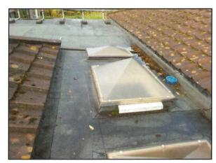
chipping has worn away from the substrate in several areas. This will subsequently reduce protection against the sunlight and will tend to accelerate the deterioration thereafter. There is also slight blistering evident to the North West corner.
