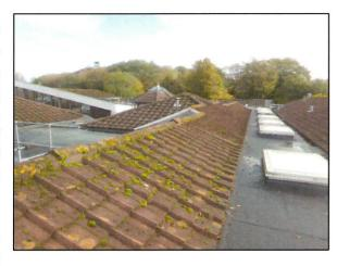
concrete interlocking tile with a distinctive angled profile. The overall size of the tile is 430 x 380mm and a tile of this nature can be laid to a minimum pitch of 17.5°. The minimum headlap for the tiles was originally 75mm but research suggests that Redland changed the specification to a headlap of 100mm for pitches below 22°. This was probably in reaction to direct damp penetration to shallow pitched roofs in exposed areas.
