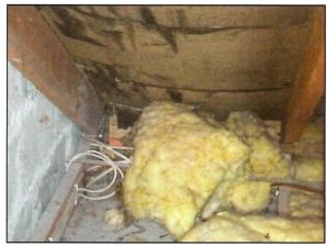
There are some pipework penetrations through the blockwork wall adjacent and the penetration needs to be fully infilled with intumescent foam or similar for fire separation.
