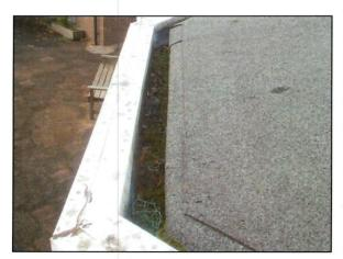
edge, with a PVC capping. The PVC capping and cladding is generally satisfactory, although some of the workmanship is perhaps slightly untidy.
