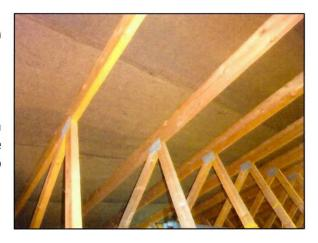
In this case, there is a bitumen based sarking felt present beneath the majority of the pitched roof coverings, above the trussed rafters, beneath the battens and tiles.
