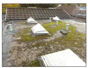
The top layers of such roofs is normally protected with a layer of stone chippings or solar reflective paint to protect against UV degradation from sunlight. This can rapidly degrade the top layer of material if it is not adequately protected. The condition and description of each section of flat roof is further described below. Later mineral felts have a crushed slate or similar aggregate impregnated in the top layer and are therefore generally without need of an additional protective coating.
