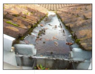
These are two substantial horizontal valley liners between facing roof slopes. These areas are lined in GRP.
