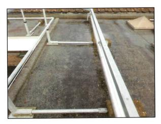
The flat roof here is generally satisfactory. The mineral felt finish opposite to where the roof lights are is now showing signs of generally weathering and you can see that the impregnated grit finish is lifting from the sub-strate. It would be sensible to schedule in some maintenance here during the coming years and the roof covering in this area could likely be overlaid with an additional layer of felt to add to the service life.
