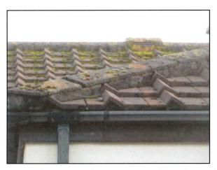
There is a generally need to clear out gutters in this area and remove moss from the roof slopes.
