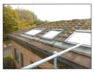
There are three Velux roof lights incorporated into P11 and these have almost certainly been retrospectively fitted at a later date. You can see a slight trace of modern breathable sarking membrane at eaves level beneath and some of the tiles under also appear to have been replaced. This is an observation as opposed to a problem and this all appears to be satisfactory.
