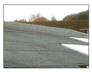
However, there are several large blisters beneath the felt, which has caused some debonding to at least the top layer.
