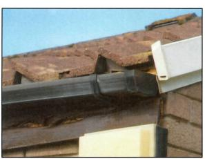
towards the right hand side. In addition, the wall plate supporting the roof structure at eaves level has also suffered slight deterioration and the sarking felt in this area has degraded around eaves.
