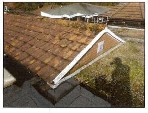
At the East end, there is a slightly raised gable above the flat roof. The lead flashing detail at the junction with the flat roof has suffered the effects of UV degradation over the years. This is becoming slightly brittle and has cracked. There is no immediate concern but this flashing will require renewal in time, certainly when the older section of flat roof adjacent is renewed.
