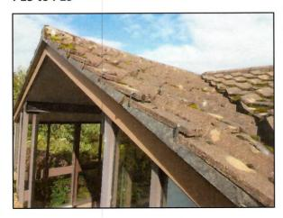
The roofs here are all over the entrance foyer. Here there are concrete tile lined valleys and the verges to either end of the entrance foyer are finished with a fibre cement slate undercloak and the gap between this and the underside of the tiles is infilled with mortar, with additional metal clips.
