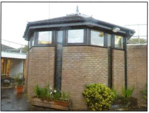
Towards the centre of the building there the octagonal structure accommodates the chapel. This is identified as room 89 on the existing floor plan. The structure in this area is formed with a timber frame and there are principle timber columns on each corner of the structure corresponding roof timbers above, held together with a series of metal ties. There is continuous glazing around the head of the structure and, below, some
