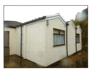
This small section of the building is almost certainly in timber framed construction, although we have not inspected the interior of this section of the building in detail to confirm.
