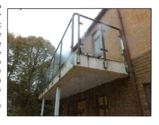
Regardless, we advise that this area is further inspected in due course and the water-proofing layer and wearing course on top assessed. It is important to try and keep water out of such structures as much as possible to prevent any possibility of reinforcing steel becoming wet and therefore corroding. Similarly, the edge protection will need routine maintenance and likely upgrading with 10 years.
