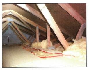
Again, insulation is lacking. To the North side of the roof void there is no insulation at all over ceilings. Consideration ought to be given to improvement in this regard.
