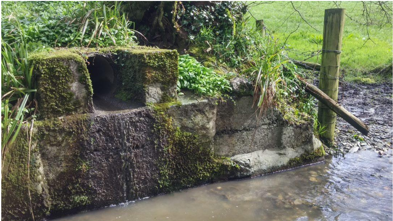
Pic 9: View of left-hand bank concrete highway drain outfall
