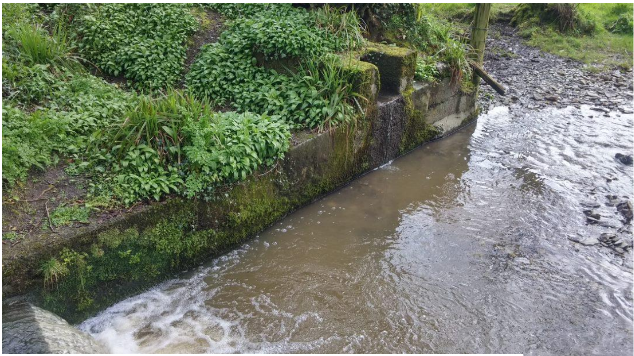
Pic 8: View of left-hand bank concrete wingwall
